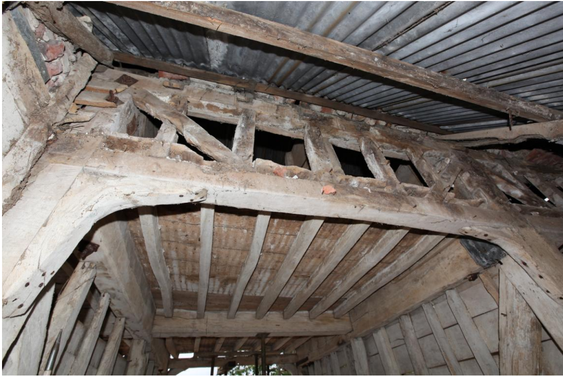
Illus. 11. Detail of the penultimate northern bay seen from the western lean-to, showing tenoned studwork and carpenter's numerals to the mid-rail and storey post. Both the mid-rail and storey post to the left are numbered III.
