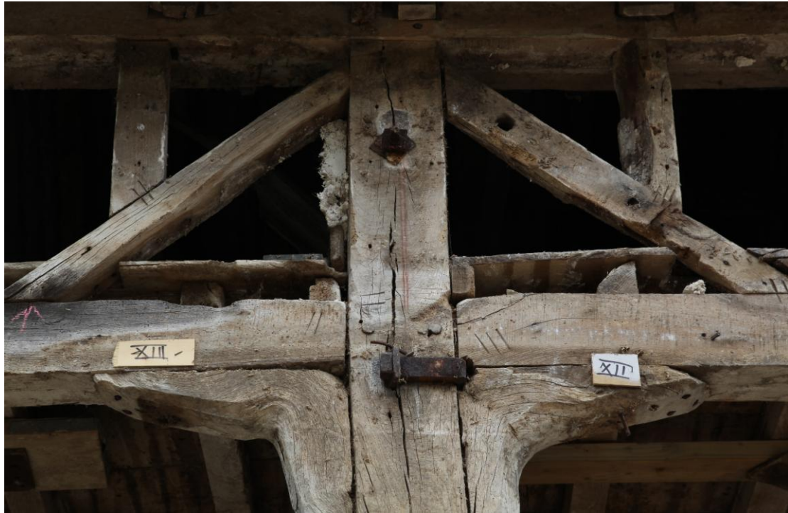
Illus. 5. Detail of the carpenter's numerals to the eastern exterior (section 3 of 10 from south to north (left to right) as photographed in Appendix 1). The mid-rail of the southern bay to the left is numbered II, as is the corresponding joist in the storey post, but the numbers II and III overlap the joints between the diagonal wall braces and the studs and mid-rails to left and right respectively.
