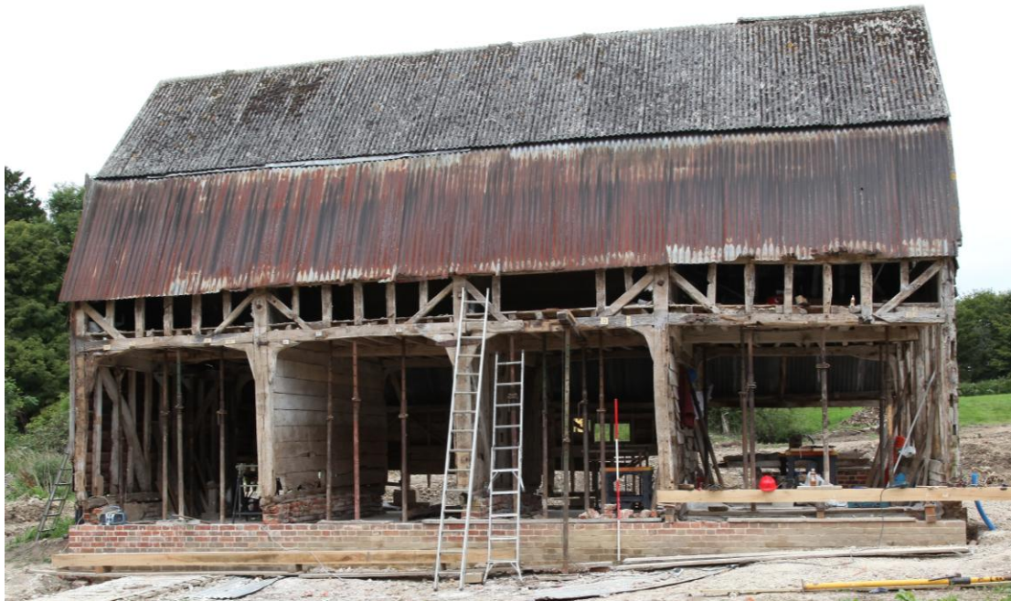
Illus. 3. The eastern exterior stripped of its cladding and showing the original knee-braces to the three formerly open southern bays to the left and the originally enclosed northern bay without knee-braces to the right.
