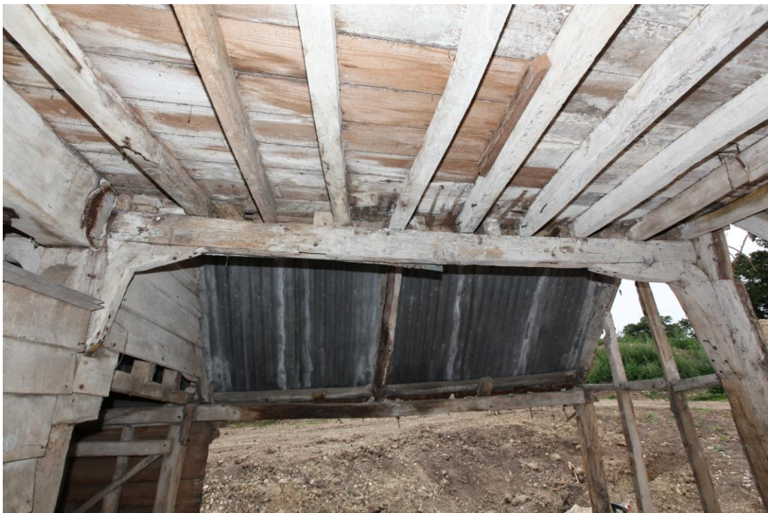
Illus. 12. The interior from the east of the wider northern bay showing two empty pegged stud mortises in the underside of the mid-rail with later knee-braces of unequal size. The front (eastern) mid-rail of this bay contains identical mortises and lacks knee-braces, suggesting the bay originally formed an enclosed vehicle or storage shed alongside the three open bays of the cart lodge.
