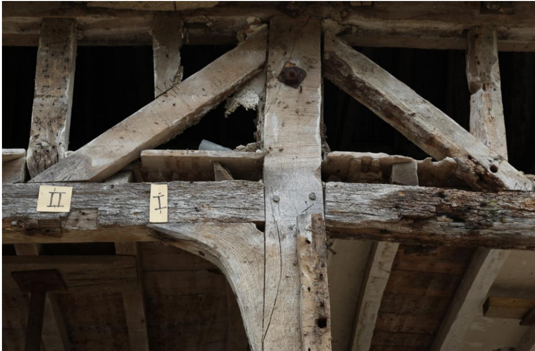
Illus. 7. Detail of the carpenter's numerals to the eastern exterior (section 7 of 10 from south to north (left to right) as photographed in Appendix 1). The numbers VII and VIII overlap the joints of the diagonal braces. Note the crude notch in the mid-rail to the left for a secondary stud of the 'stable' conversion.
