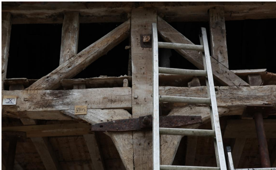
Illus. 6. Detail of the carpenter's numerals to the eastern exterior from (section 5 of 10 from south to north (left to right) as photographed in Appendix 1). In this case the numbers VIII and V overlap the joints between the diagonal wall braces and the studs and mid-rails to left and right. This 'block' system of marking, and the overlapping of the joints (which would have rendered the numbers very difficult to read in isolation) is unusual.
