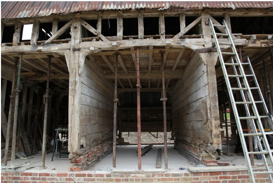
Illus. 4. Detail of the eastern exterior showing the central open bays with original nailed knee-braces to both front and rear. There are no mortises for original studs or wall braces beneath the mid-rails to match those which survive to the granary floor above, and the studs of the 'stable' conversion recorded in 2008 were notched and nailed in the standard manner of secondary insertions
