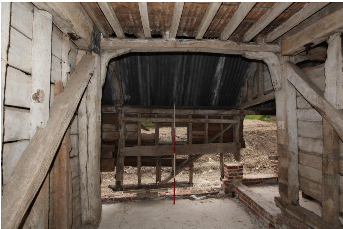
Illus. 10. The interior from the east of the penultimate northern bay showing the nailed knee-braces to its rear mid-rail and the narrow studs of the lean-to.
