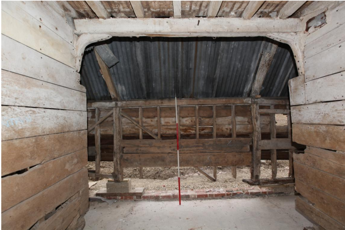
Illus. 9. The interior from the east of the penultimate southern bay showing the original nailed knee-braces to its rear mid-rail. The narrow studs of the rear lean-to, each crudely notched over a continuous fillet of timber nailed to the underside of the roof-plate, contrast dramatically with the quality of the main structure and suggest the lean-to is a later addition relating to the 'stable' conversion.
