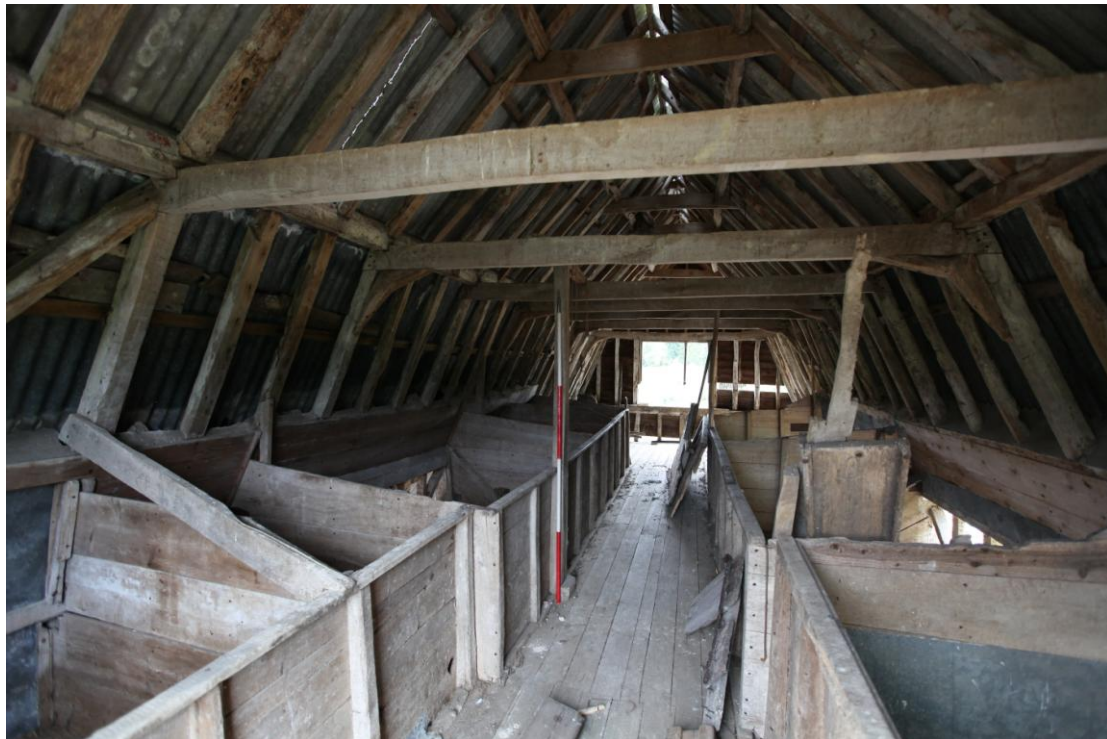
Illus. 8. The interior of the first-floor granary from the south showing the impressive array of 19 th century boarded grain bins with an axial passage leading from the external entrance to a window in the northern gable.
