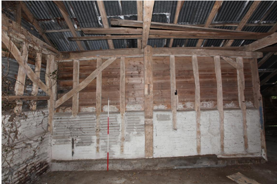
Illus. 9 The eastern interior of the intact northern bays (A and B) showing their internally trussed wall braces (truncated by the later entrance to the threshing floor to the right) with mortises for a first-floor partition and binding joist in the central storey post with the apparent notches of a hay rack beneath.
