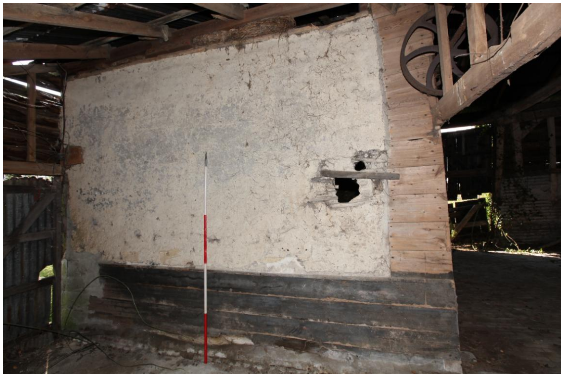
Illus. 4 The original eastern external whitewashed roughcast clay render to the 18 th or early-19 th century southern bay (D) with later tarred boarding to its base (seen from the 20 th century lean-to (E) and showing the pulley wheel attached to its tie-beam to the right)
