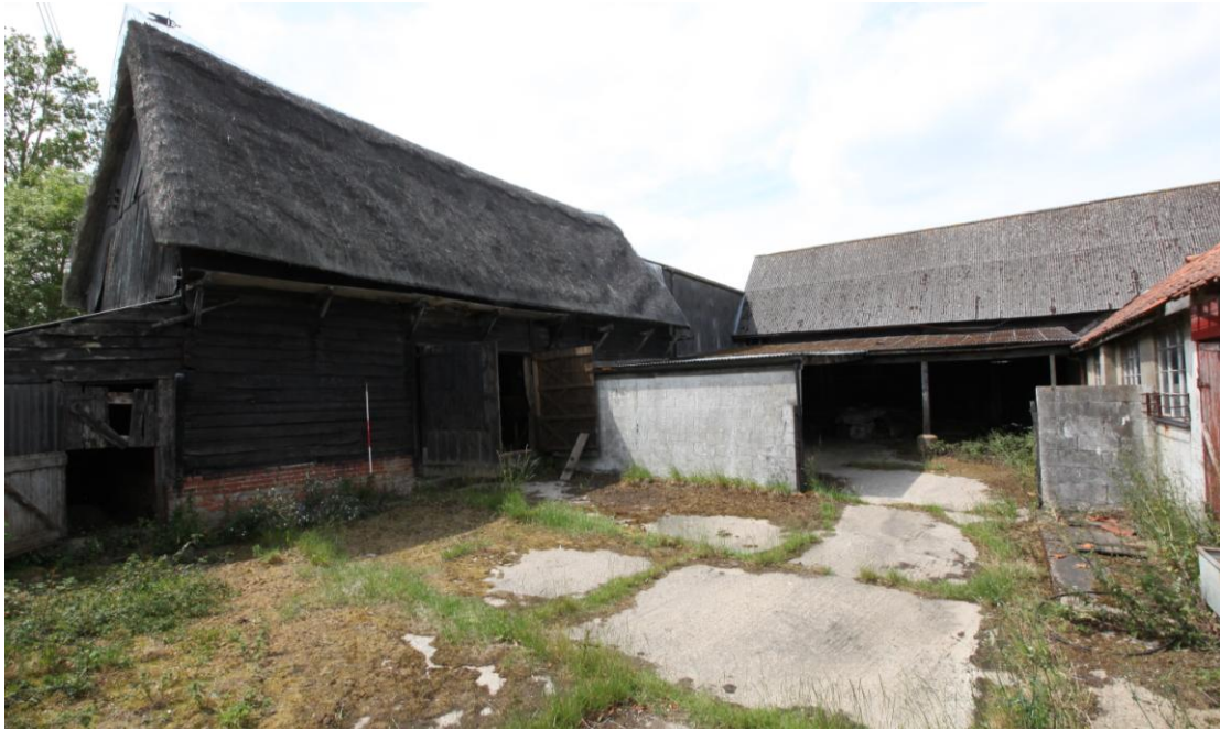
Illus. 3 The eastern exterior of the thatched barn (1) from the adjoining yard showing its close proximity to the contemporary middle barn to the right. Note the unusual guttering of corrugated iron supported on wooden brackets beneath the thatch eaves. The framing and condition of the two barns are almost identical but the thatch of the middle barn has been replaced with corrugated asbestos.
