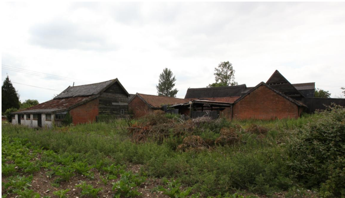
Illus. 12 The farm complex from the north-east showing the 19 th century brick shelter-sheds of the two eastern yards (5 and 6) with the two barns in the rear and the well preserved 19 th century weatherboarded stable to the left.
