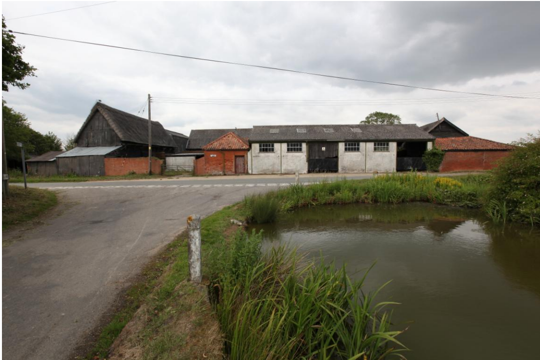
Illus. 1 General view of the farm complex from across the farmhouse moat to the south, showing from left to right the grade II-listed 16 th century thatched barn (1) with the contemporary ‘middle barn’ (2) in the rear, the brick dairy range (7) and 20 th century covered yard (6) in the centre and the 19 th century weatherboarded stable (4) with its brick southern lean-to to the right.
