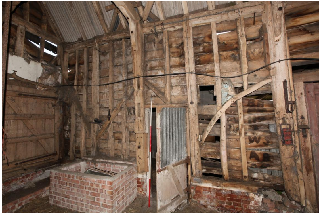
Illus. 11 Middle barn (2). The southern interior of the two eastern bays (2E and 2D) which originally formed a stable with a loft. The present door and the main entrance to the extreme right (bay C) are secondary, the latter replacing the previous thoroughfare in bay B in the 19 th century. The majority of the common studs are 19 th century replacements but the stud to the right of the central door is original and contains the mortises of a diamond-mullion loft window sill to its left and the lintel of a blocked door to its right.
