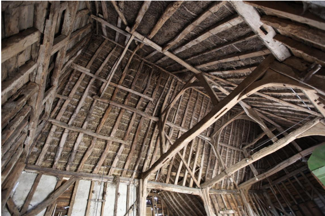
Illus. 4 Thatched barn (1). The fine late-16th century queen-post roof structure from the south-east, showing the evidence for an original half-hip with a gablet to the southern gable. The present vertical gable is part of an extensive 19 th century refurbishment which included the insertion of a new ground sill and brick plinth, along with the replacement most of the original wall studs. Note the empty mortises of the arch-braces to the tie-beams replaced with knee-braces at the same time.
