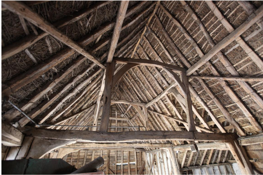
Illus. 5 Thatched barn (1). The queen-post roof structure from the south showing the original ridge-piece and the purlin braces that are confined for decorative effect to the threshing bay (1B). The middle barn (2) is identical in this respect.
