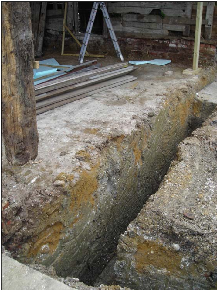
Plate 5. Footings, south east corner of extension. Looking west
