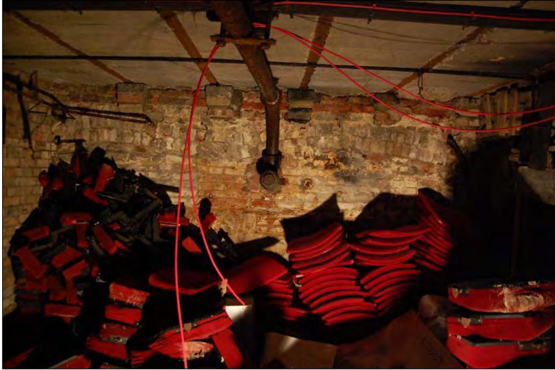
Plate 7. Above – Room 4, bricked-up archways, facing WSW
