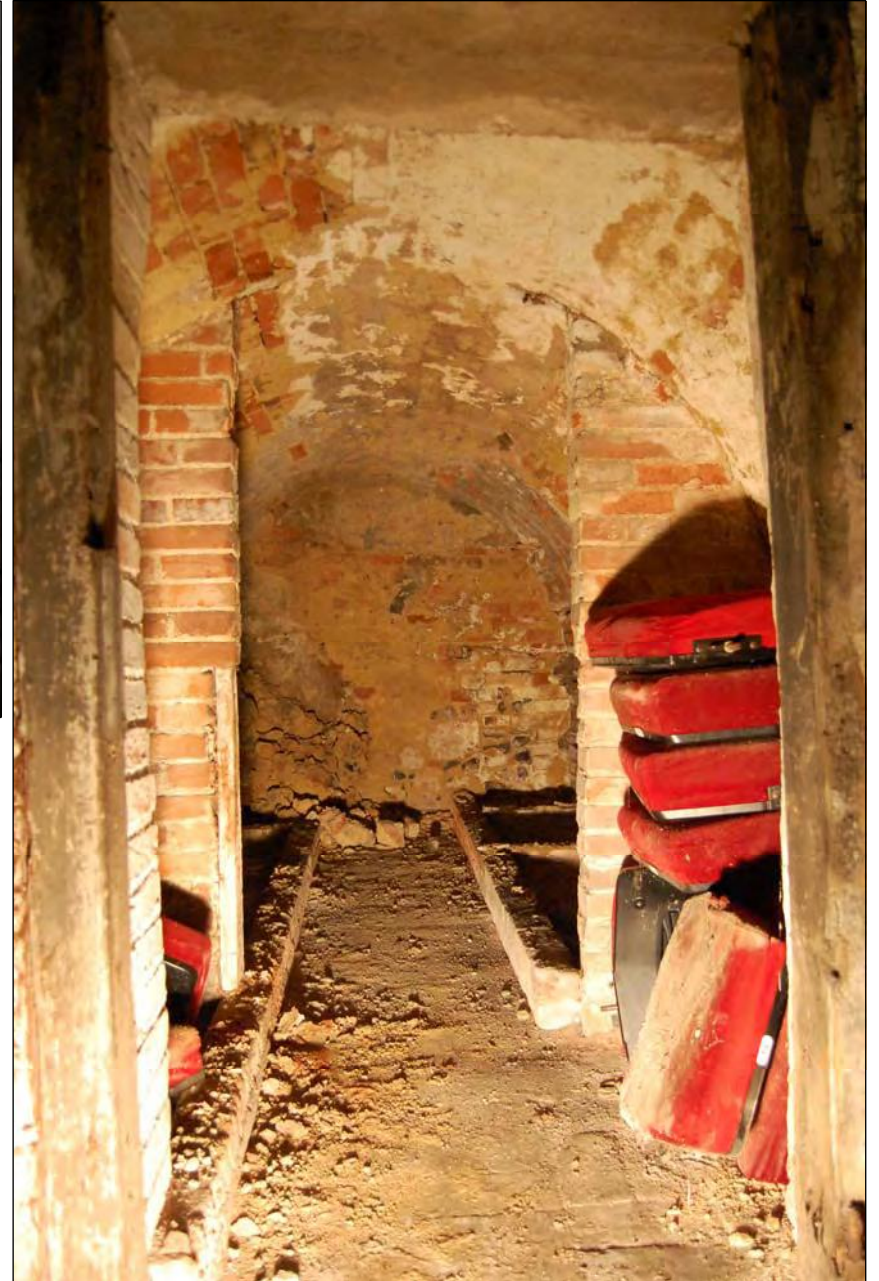
Plate 6. Right – Room 3 showing subdivisions in layout, vaulted ceiling, and brick floor divisions
