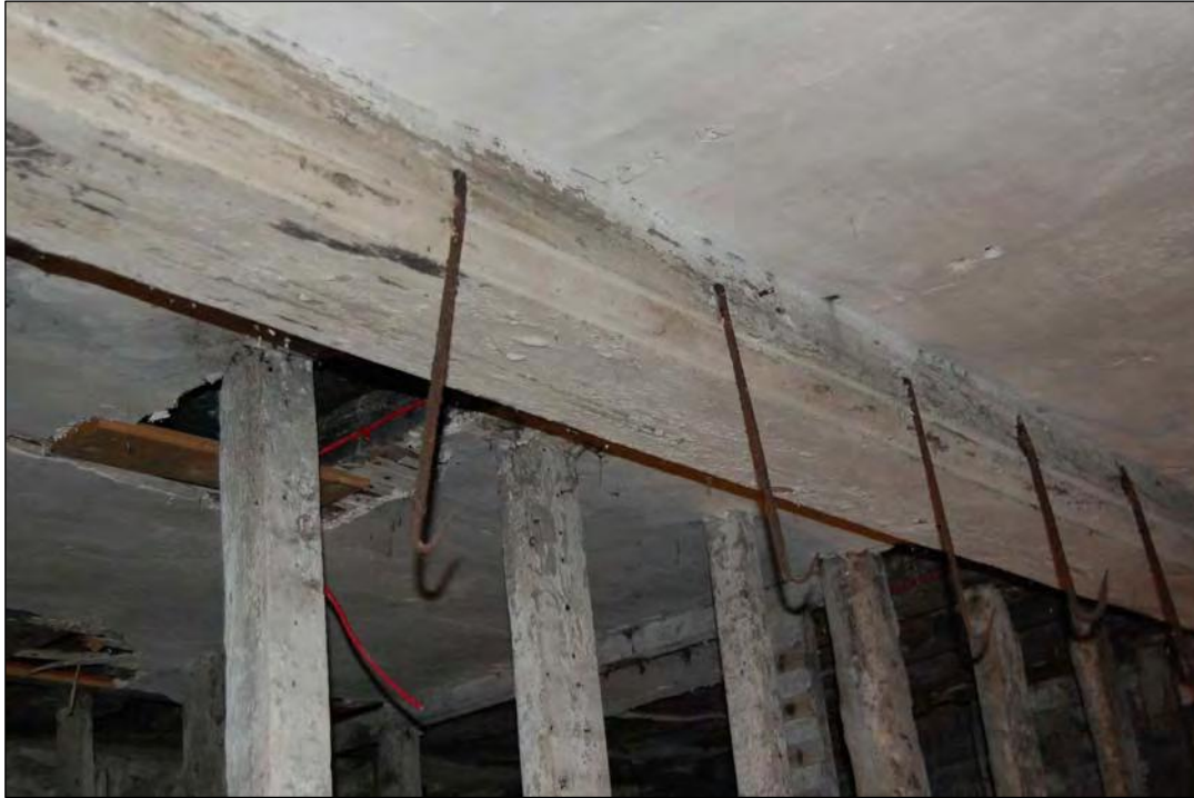
Plate 5. Above – Molded timber in Room 1 with iron hooks
