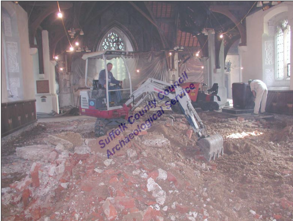
Removing Existing Floor Levels
