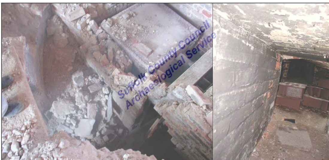
Plate 2 Firebox in Pit & Top of Firebox Seen From Vent
