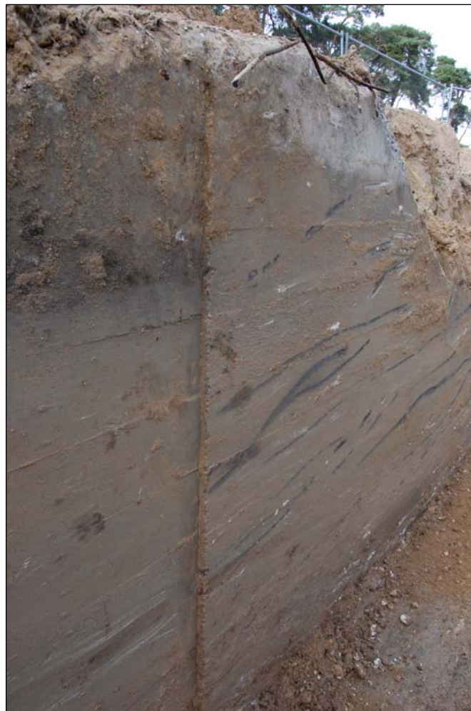
Plate 5. Internal shot of Air Raid Shelter wall, showing construction methods
