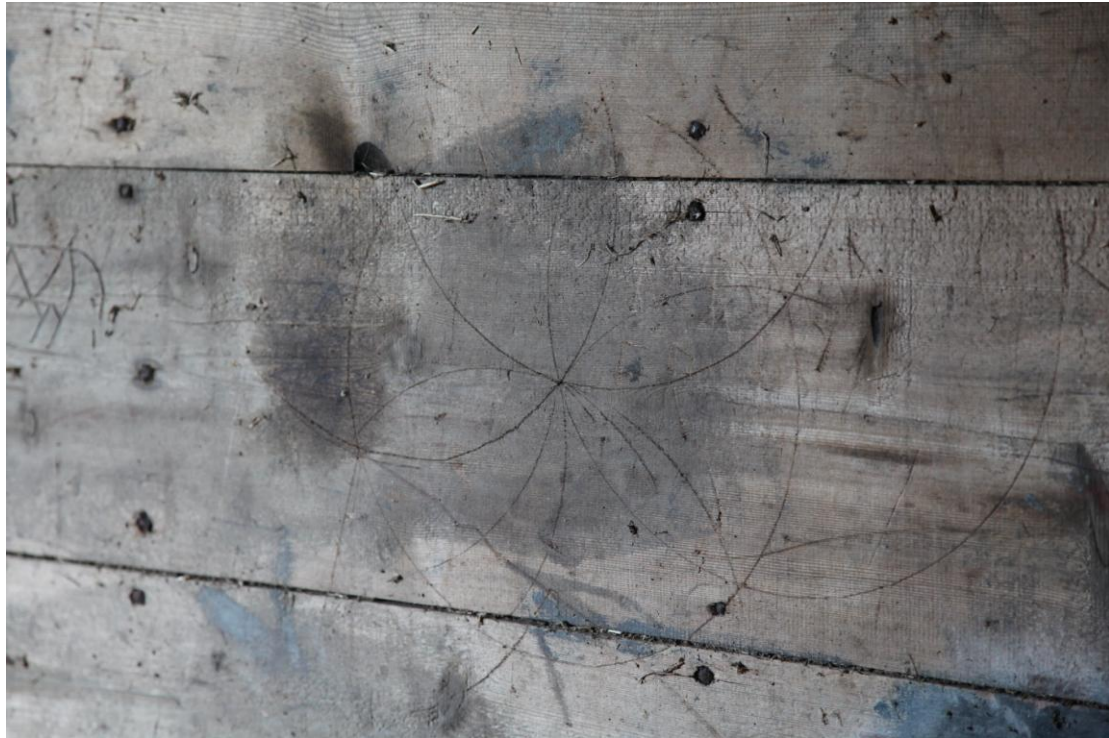
Illus. 11. The interlocking incised apotropaic circles on the deal boarding of the partition of stable (1b) exposed in the main barn (1a). Each circle is 33 cm (13 ins) in diameter.
