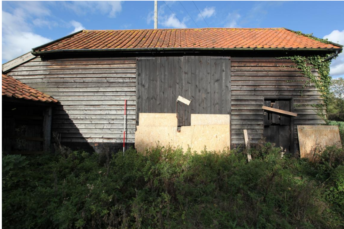
Illus. 5. The southern exterior of the main barn (1a) showing its renewed late-20th century weatherboarding and central entrance doors, with the half-hung door to the stable (1b) to the right and the open-sided section of the single-storied yard shed (1d) to the left.
