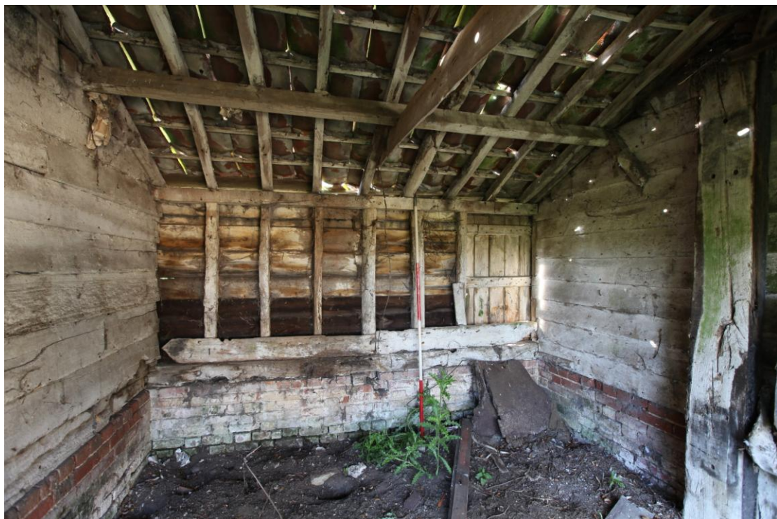
Illus. 6. The western interior of the open-sided yard shed (1d) showing its brick plinth with the feed loading hatch to the right and the boarded partitions of the enclosed southern shed (1e) and the lean-to shed (1c) to the left and right respectively.
