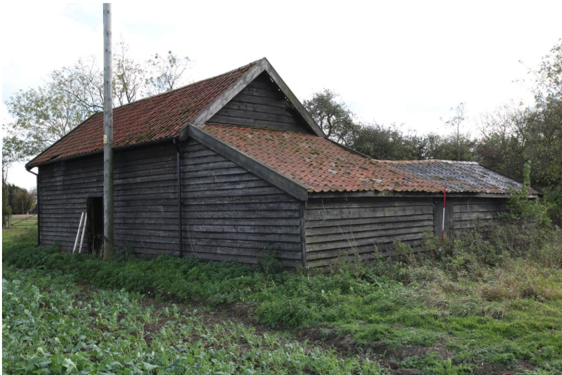
Illus. 4. The exterior of Saviours Barn from the north-west showing the pantiled lean-to shed (1c) adjoining the western gable with the single-storied yard shed (1d & 1e) to the right.
