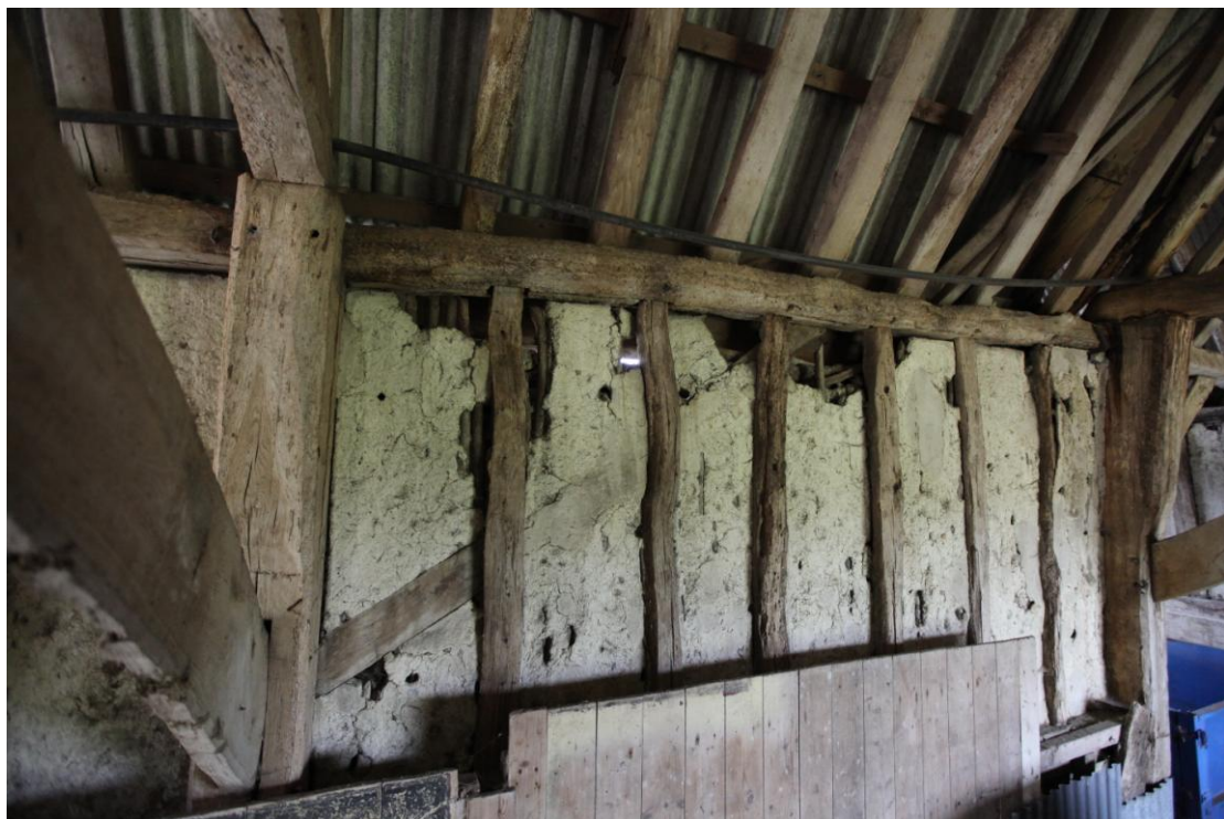
Illus. 10. The southern interior of bay D showing its intact external wall brace and wattle-and-daub, with entrance the entrance to the porch (1a) in bay C visible to the right.
