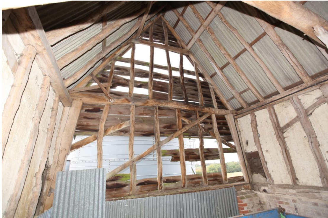
Illus. 9. The interior of the porch gable (1a) showing its original external wall braces to left and right with a later nailed internal diagonal brace in the centre. The mid-rail is an original feature but any evidence of the original doorway is obscured; the chamfered brick jamb to the right is an addition of the 19 th century.
