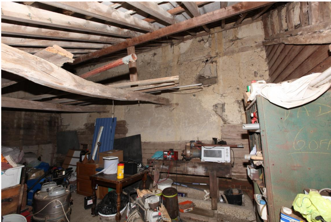
Illus. 4. Interior of lean-to shed (3) from south showing the original external render to the southern elevation of the barn (consisting of vertical coppice poles tied to nailed horizontal laths).
