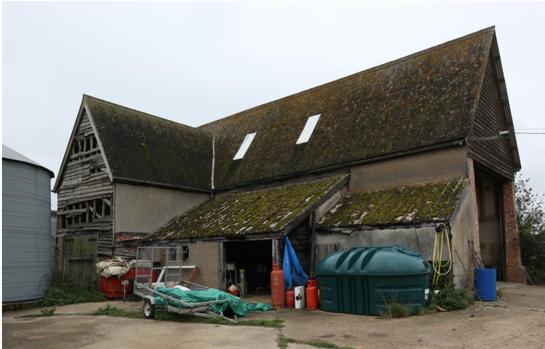
Illus. 3. Southern exterior showing original porch (1a) to left, lean-to tack room (2) to right and lean-to shed (3) in centre.
