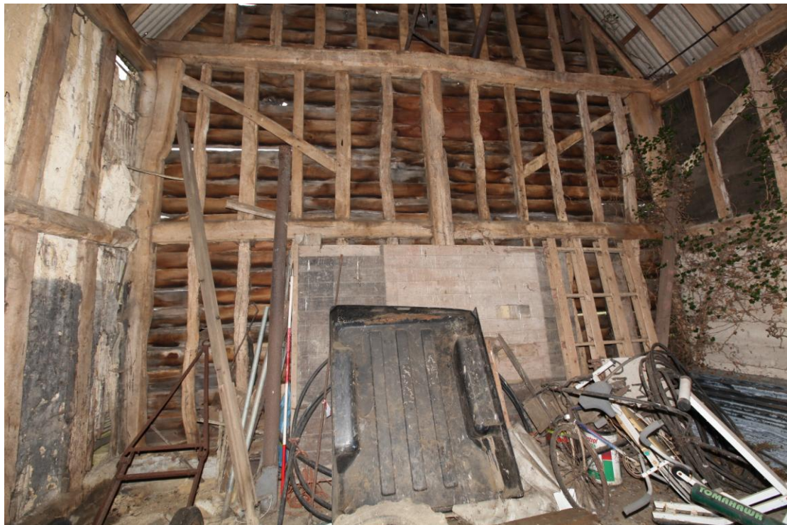
Illus. 6. Internal western gable showing the highly unusual original combination of an internally trenched wall brace to the left and external trenching to the right.
