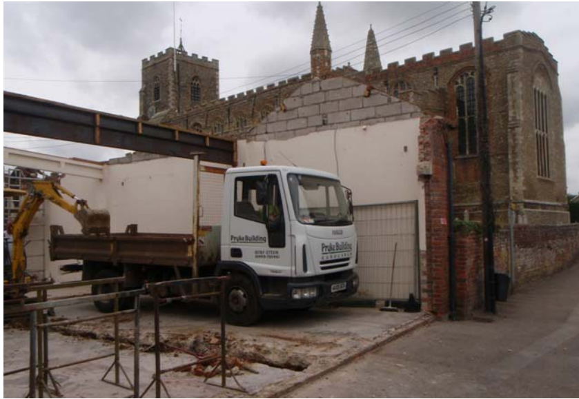
Plate 1. The site facing south.
