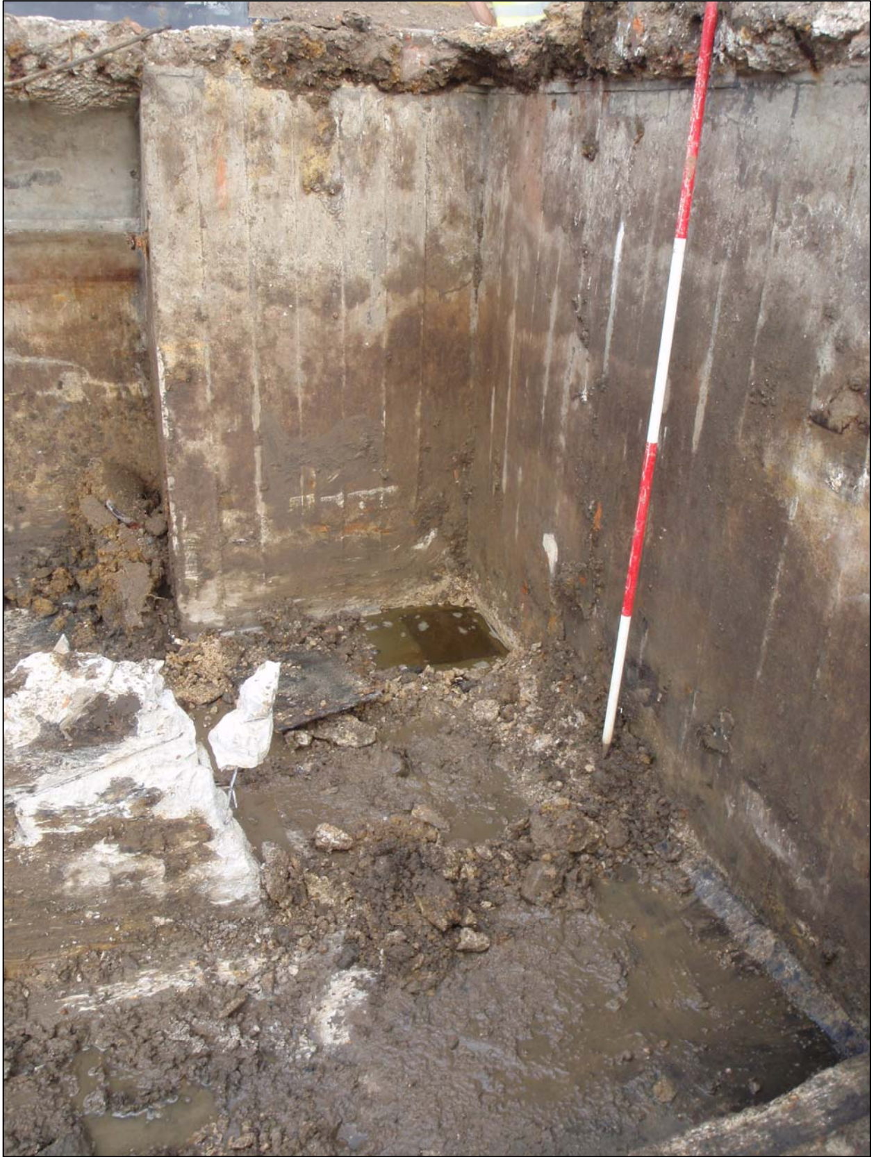
Plate 38 Shelter 4, showing the (water filled) drain in corner of passageway. The vertical lines from the timber plank shuttering are clearly visible (ref. HLQ 71)
