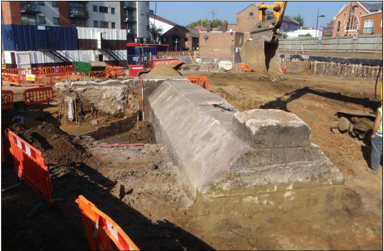
Plate 50 Shelter 6, camera facing north-west (ref. HLR 20)
