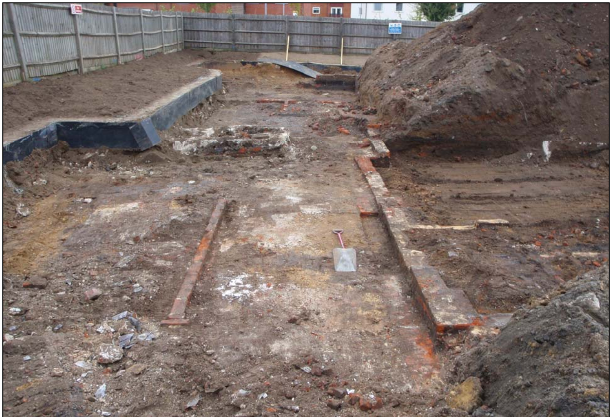
Plate 8 Walls 0065 (right, adjacent shovel) and 0116 (left), interpreted as supports for timber floor joists, between these Surface 0075 is just discernible (ref. HLP 26)
