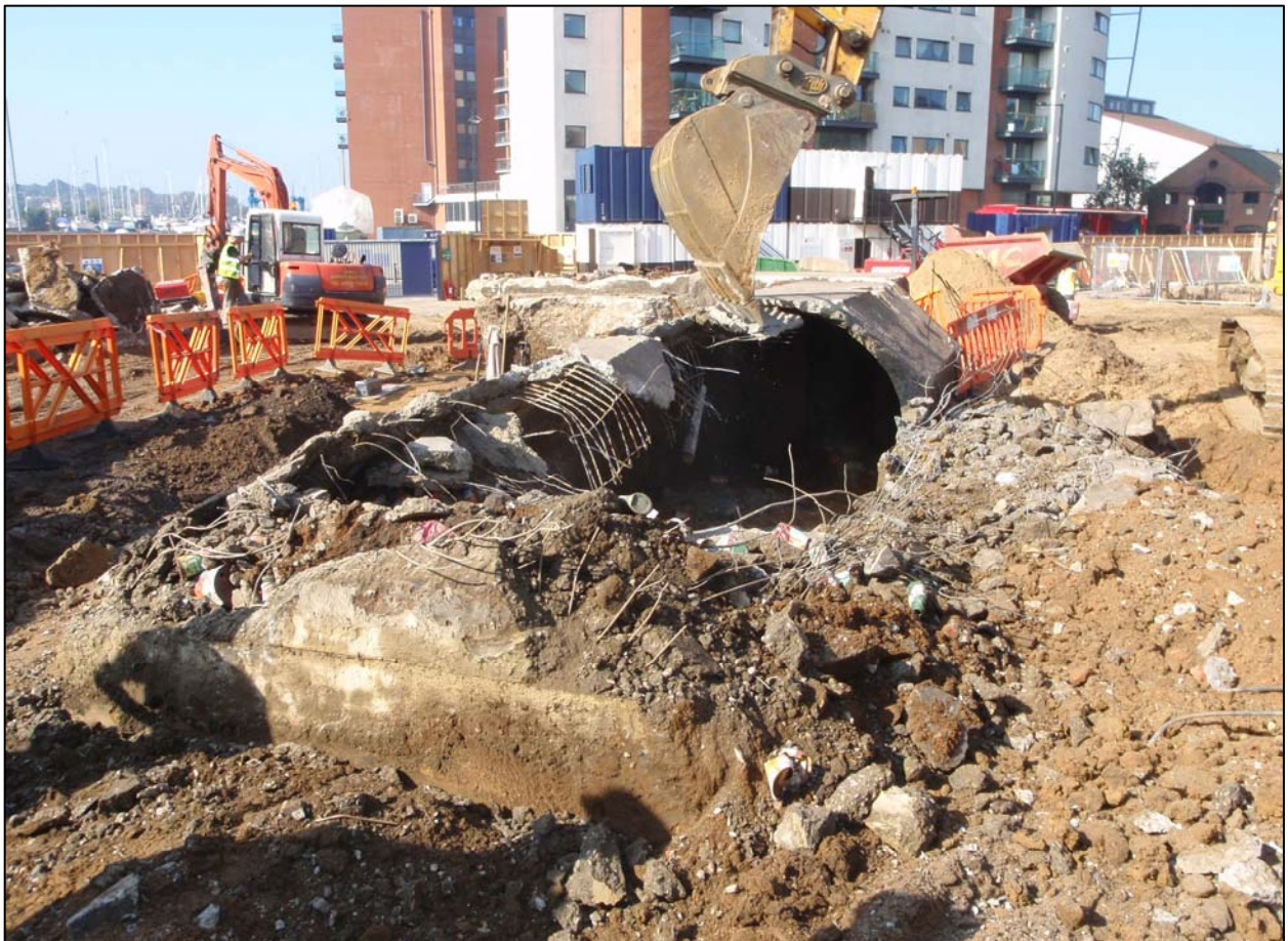
Plate 51 Shelter 6 during demolition, revealing the steel reinforcing (ref. HLR 23)
