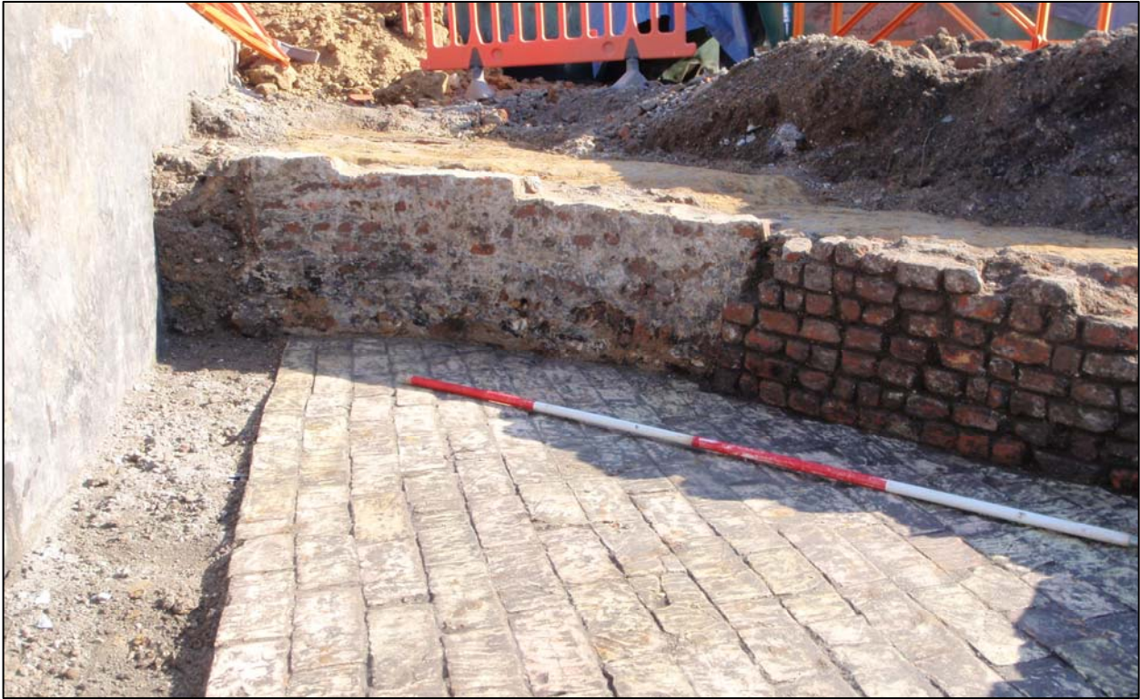
Plate 23 variation between Walls 0097 (left) and 0113 (right).
