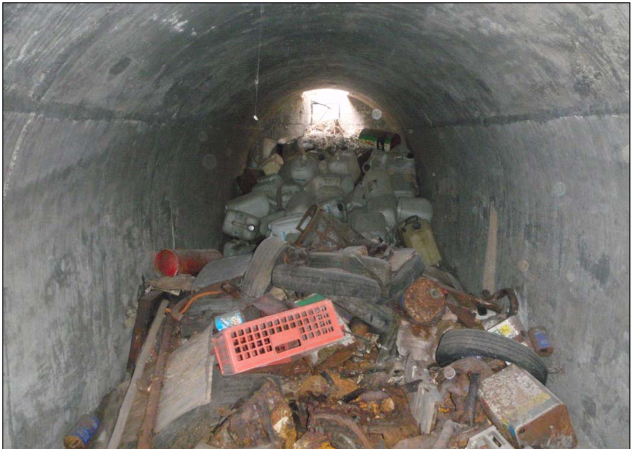
Plate 28 interior of Shelter 1 looking towards the escape hatch (ref. HLQ 35)
