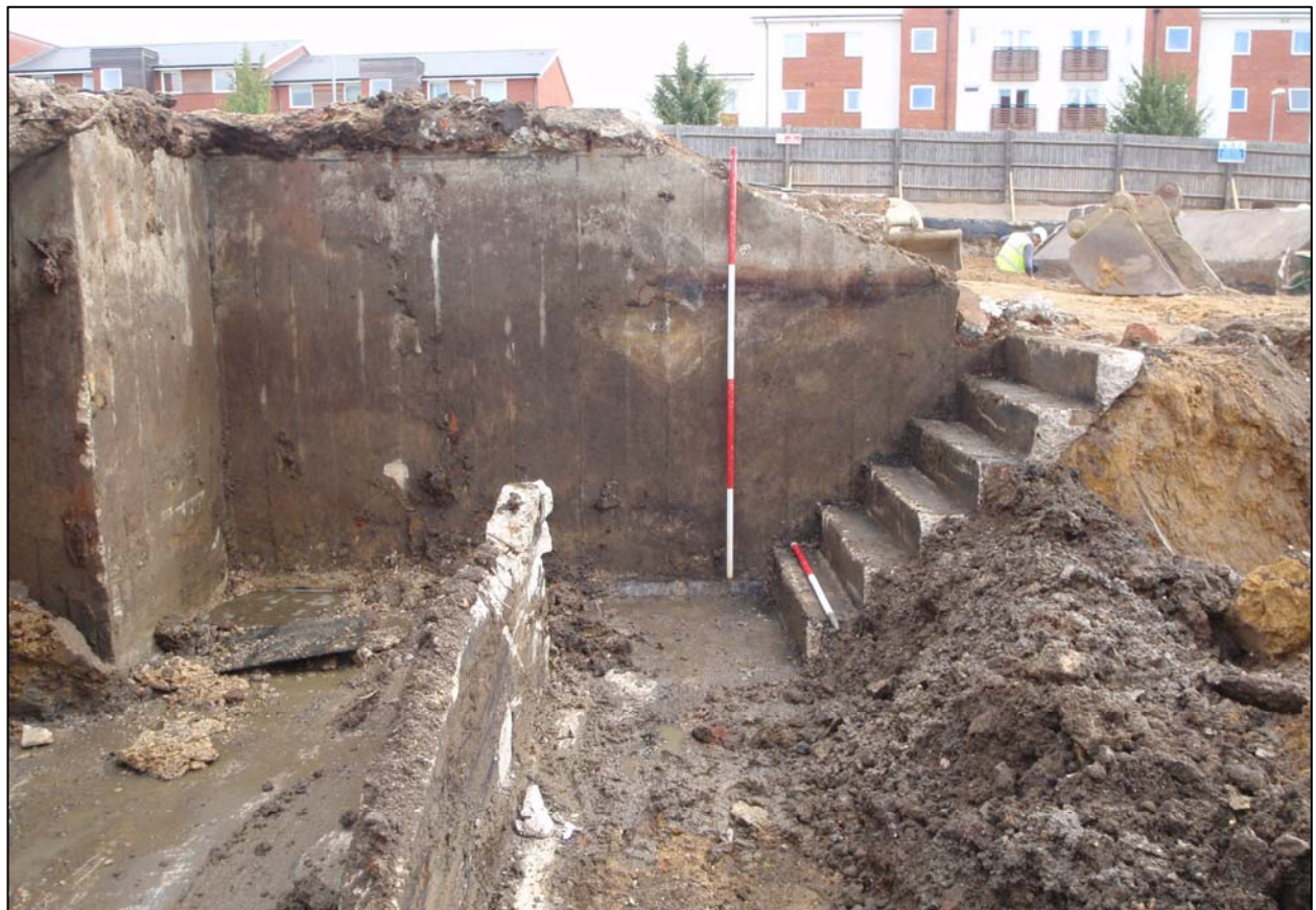
Plate 36 Shelter 4, during demolition, showing the stairs and entrance passage (HLQ 64)
