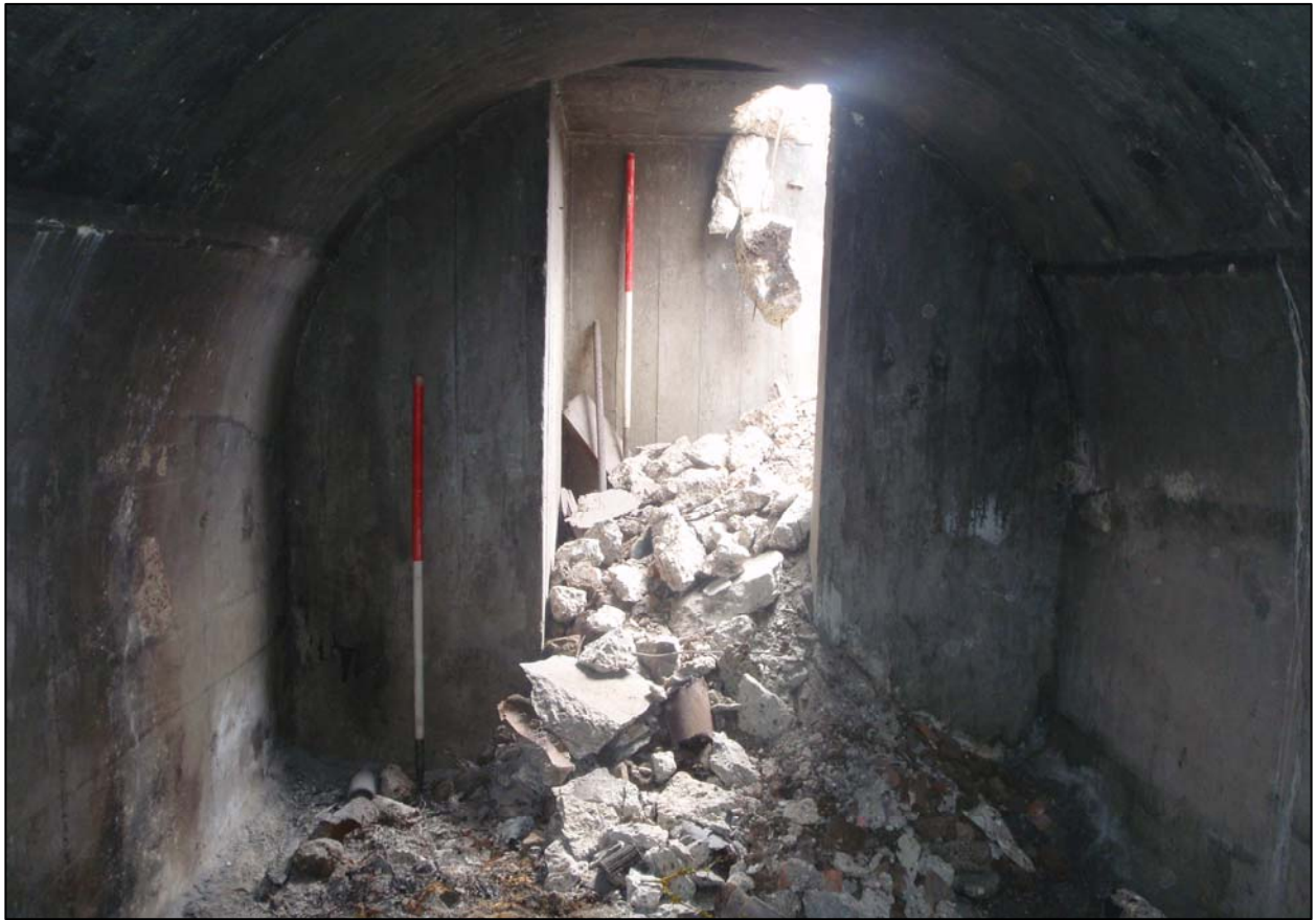
Plate 27 interior of Shelter 1 looking towards the main entrance (ref. HLQ 36)
