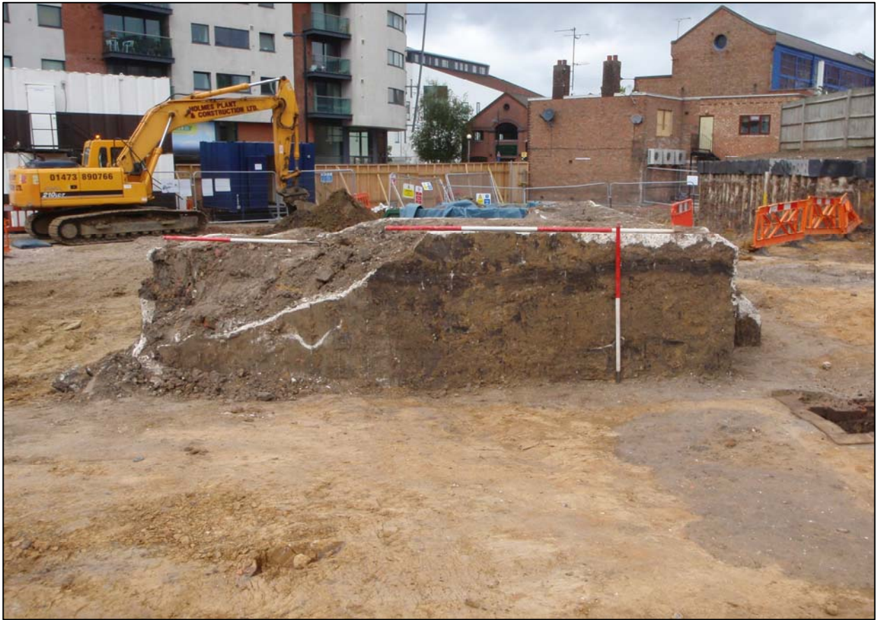
Plate 33 Shelter 4, camera facing north-west (ref. HLQ 53)
