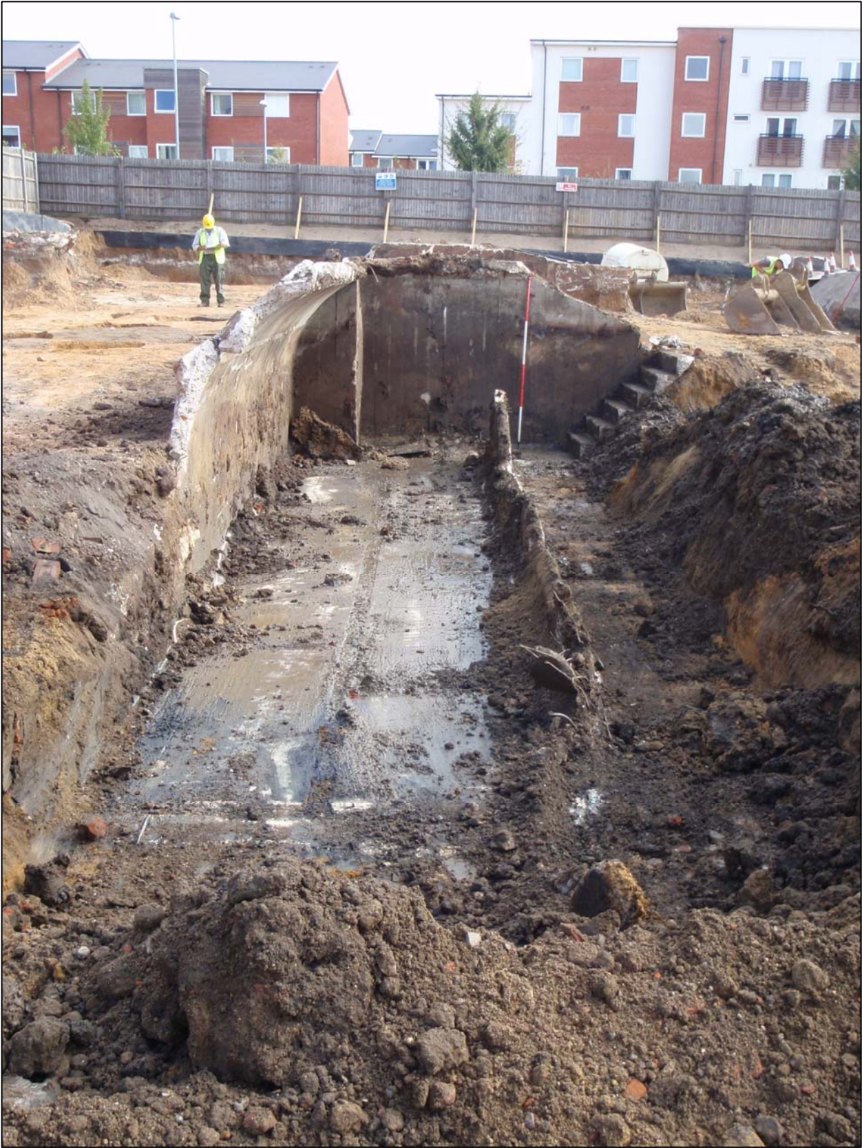
Plate 39 Shelter 4 during demolition, camera facing south-east (ref. HLQ 67)
