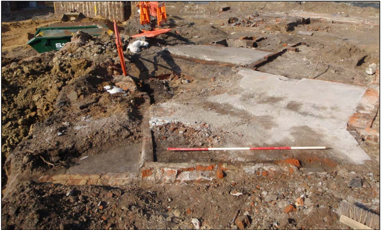
Plate 18 rear wall of houses 4 and 5 (0089) and backyard surfaces 0077 and 0076 beyond (ref. HLP 79)
