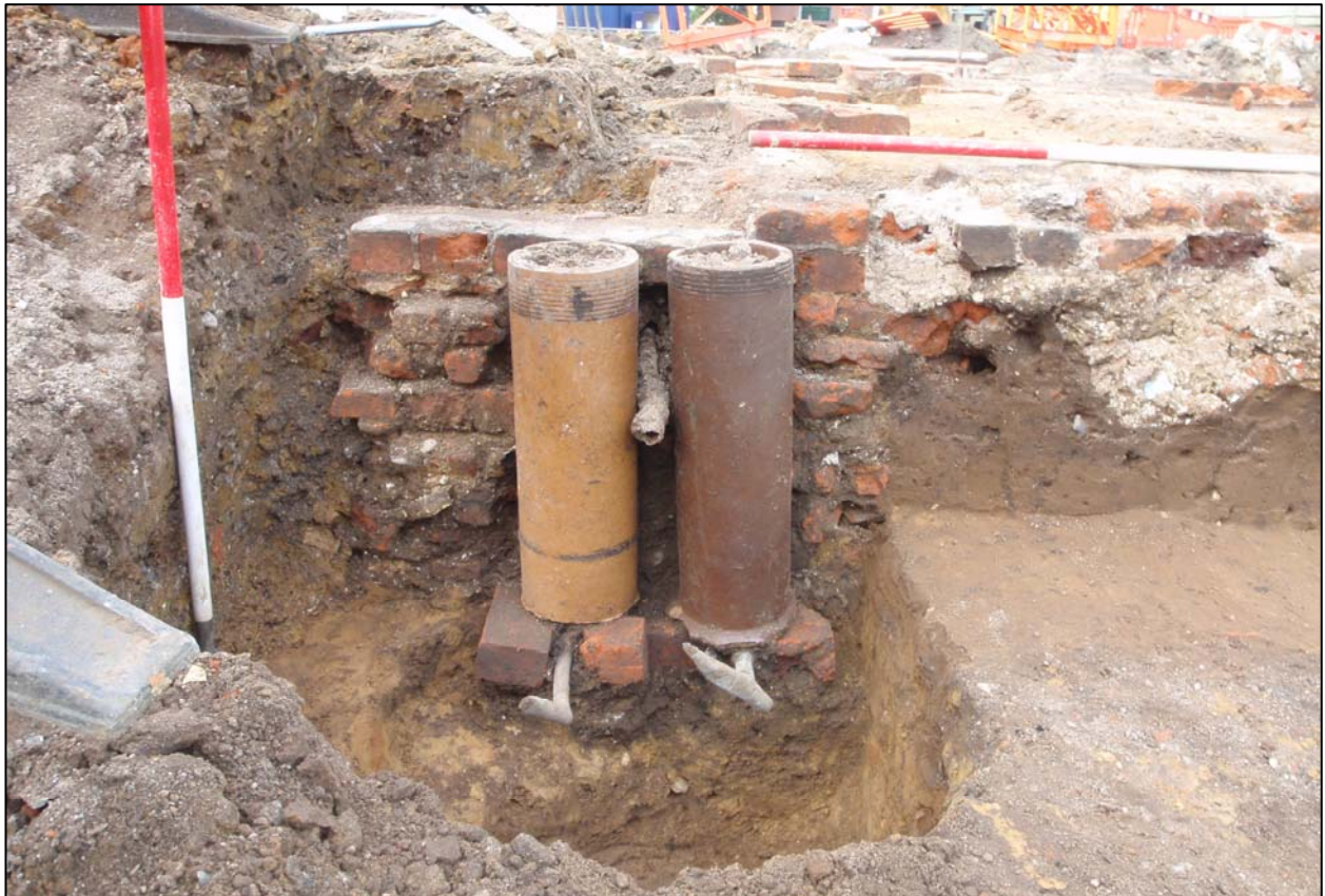
Plate 17 ceramic drainage pipes used to provide access to the stopcocks, the probable gas supply pipe is also visible (ref. HLP 72)
