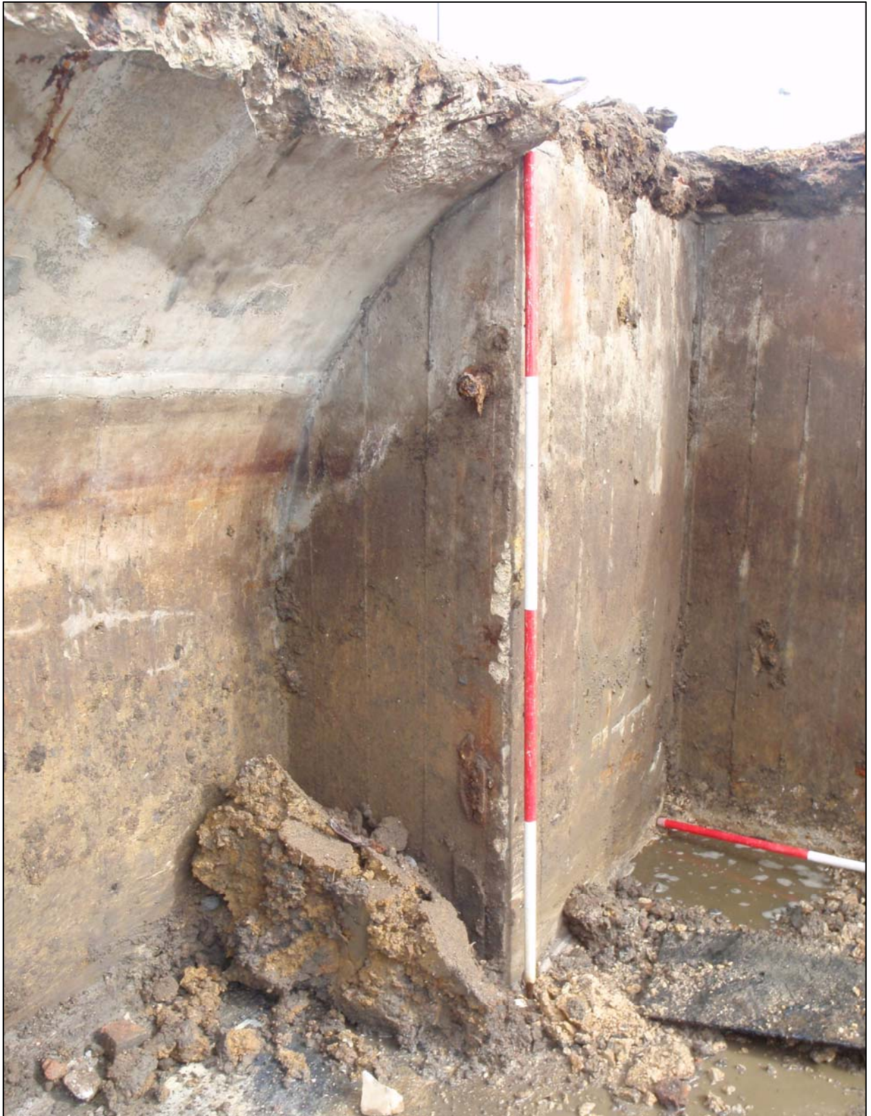
Plate 37 Shelter 4, degraded timber fragments, showing position of a door frame
