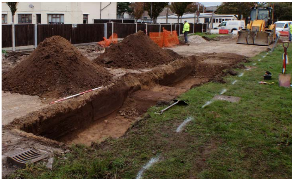
Plate 10. Trench 13 facing north (scale bars at 0.5m)
