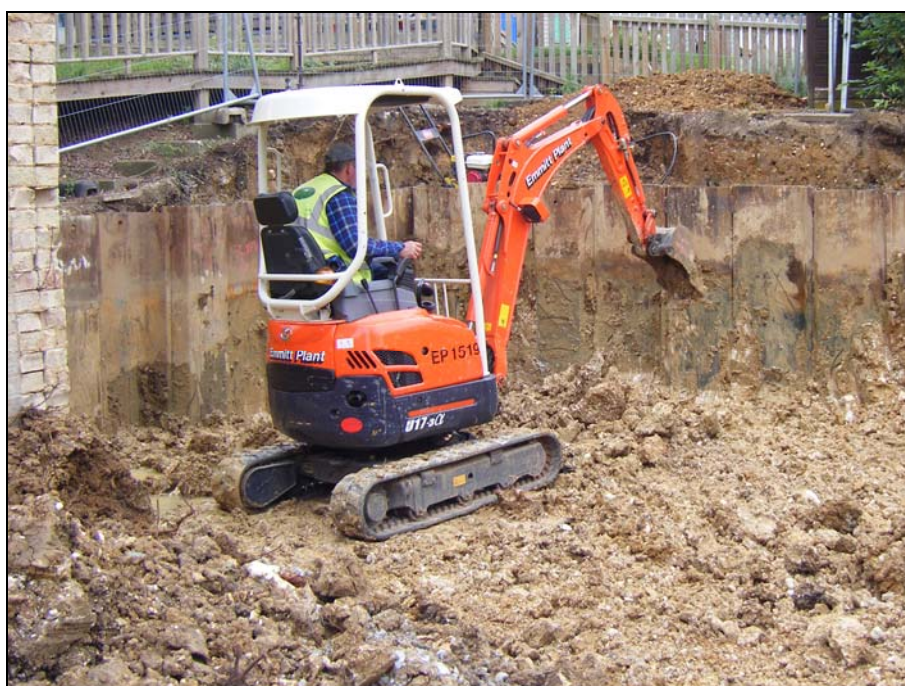
Plate 5. Chalky boulder clay beneath the extension, facing north east
