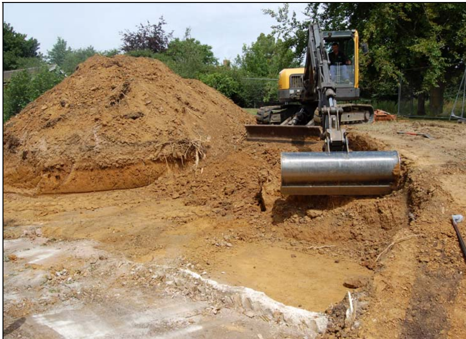
Plate 1. Stripping for the new car park
