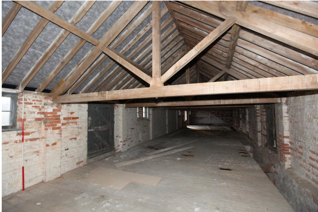
Illus. 13. The interior of the hay loft on the undivided upper storey seen from the north-east and showing the original prefabricated king-post softwood roof trusses with a hay drop in the floor to the right.
