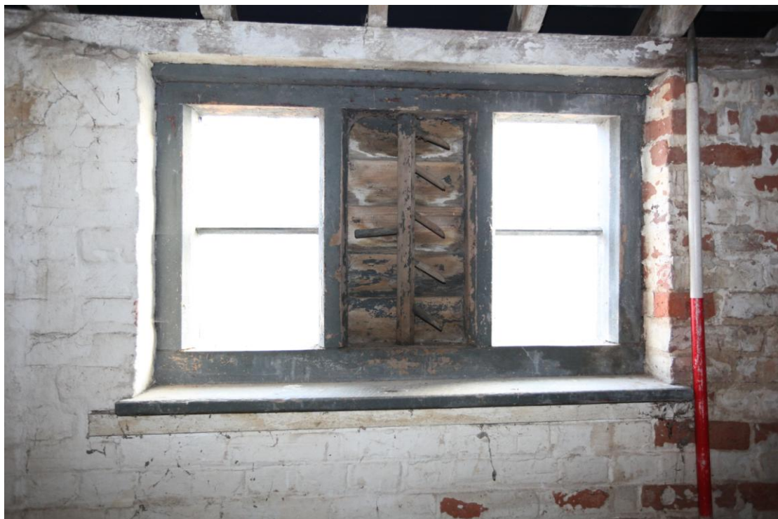
Illus. 14. Internal detail of an original hay loft window in the southern elevation showing the central louver in the closed position. Wooden pegs raise each slat when the vertical spindle is turned.
