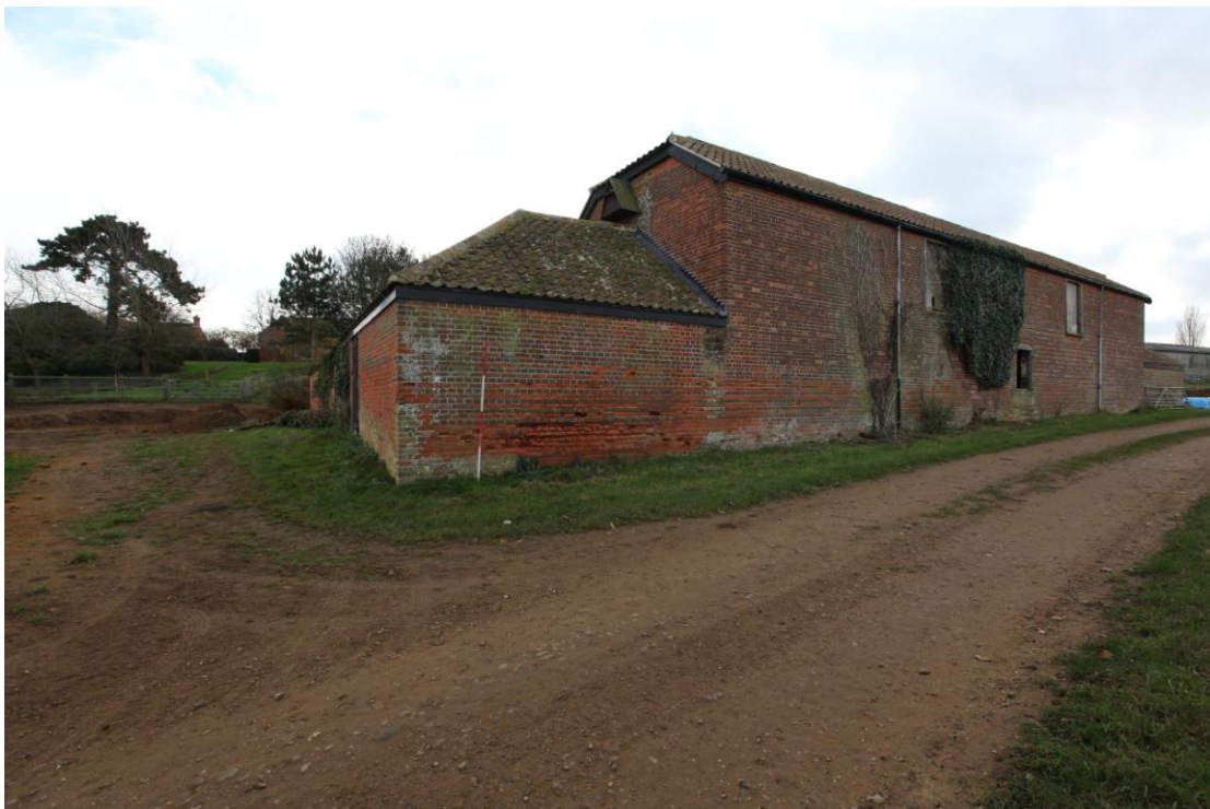
Illus. 2. The stable range from the north showing the chimney of the farmhouse in the rear to the left. The single storied sheds flanking the main stable range are integral features, and the central window to the tack room and both first-floor loft doors visible here are original.
