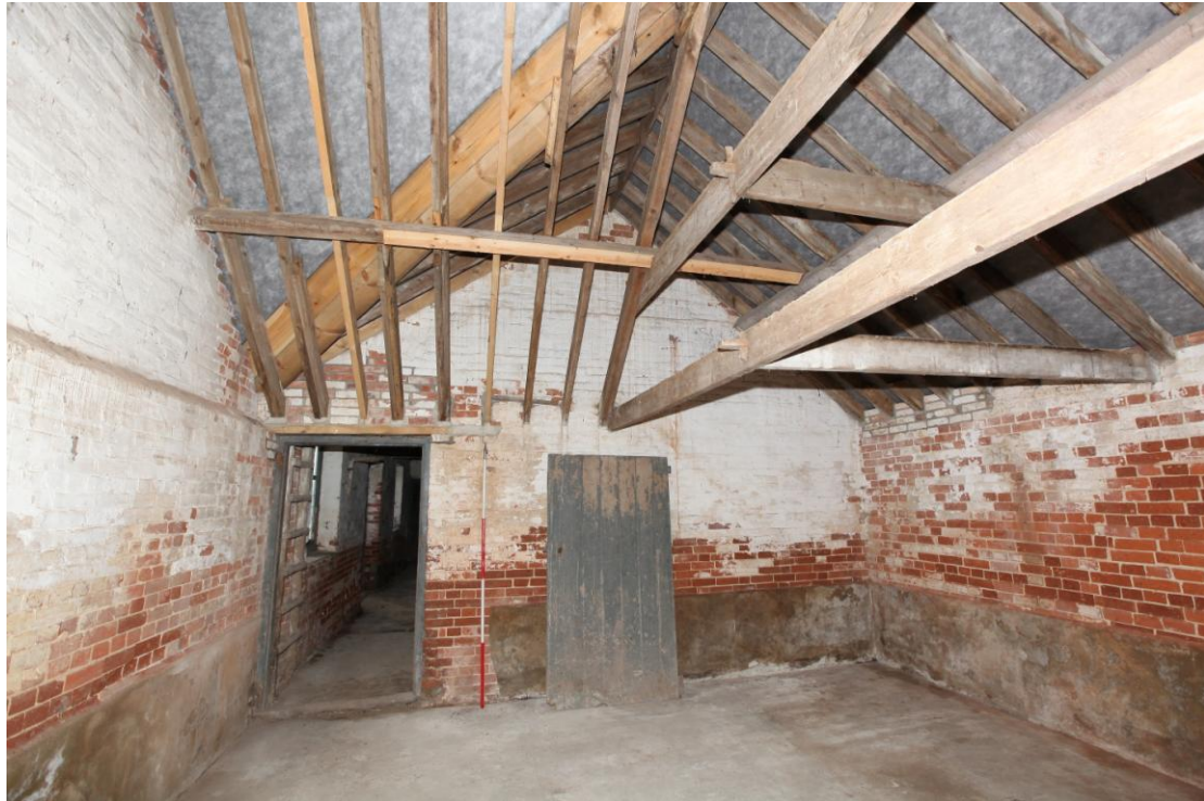
Illus. 7. The interior from the north-east of the single-storied eastern shed (E) showing its original softwood roof structure (with some recent repair) and the connecting door to the eastern stable (D).
