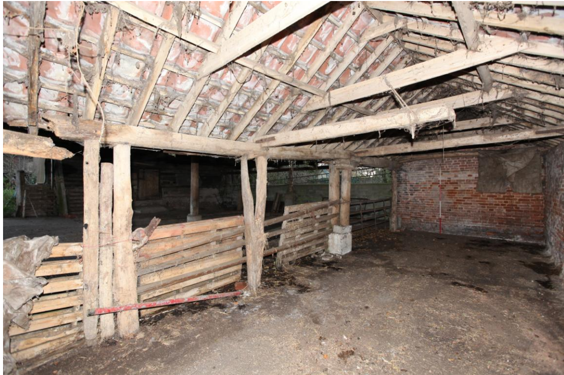
Illus. 7. The interior of the 19 th century brick shelter-shed (2) from the north showing its renewed cylindrical arcade posts to the left and the original softwood roof structure of clasped-purlins with nailed collars (typical of the latter part of the 19 th century).
