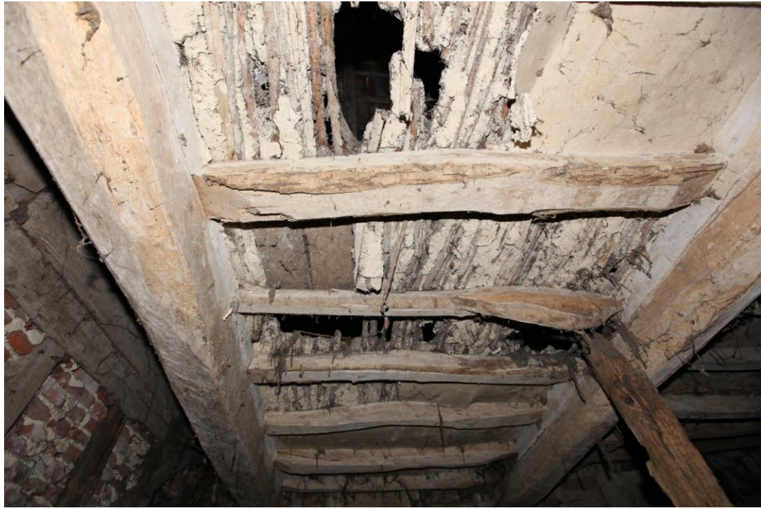
Illus. 11. A detail from the east of the ceiling in the southern stall of the stable (1a), showing the wattle-and-daub laid over the joists (under the loft boards) with the hay drop to the left.
