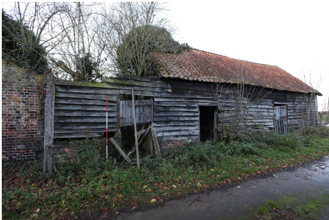
Illus. 4. The eastern exterior of the stable range (1) showing the three entrance doors to the partly collapsed loose-box (1c) to the left, the tack room (1b) in the centre and the stable (1a) to right.
