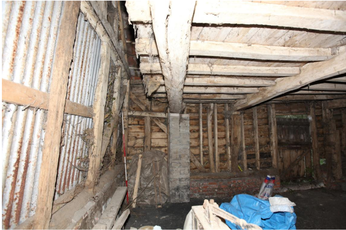
Illus. 9. The interior of the stable (1a) from the west showing the hay drop in the ceiling against the northern gable (clad in corrugated iron) to the left and the door to the farm track to the right.
