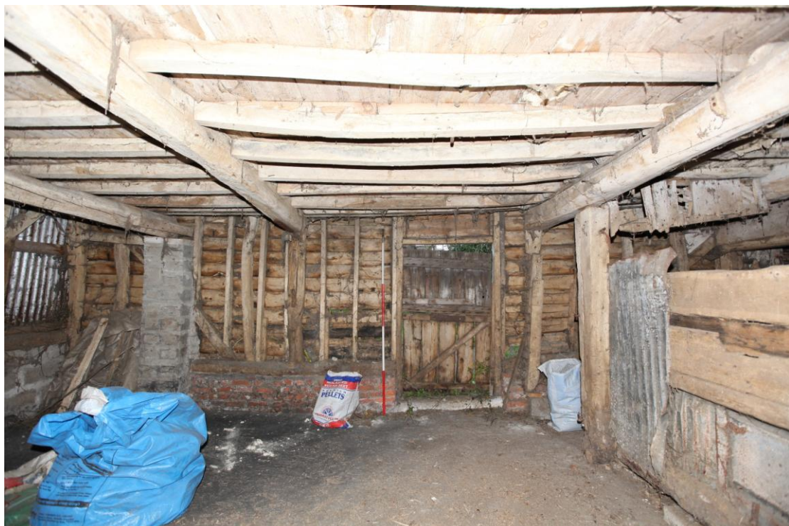
Illus. 8. The eastern interior of the stable (1a) showing the half-hung door to the farm entrance track with hay drops in the ceiling to both left and right (the mangers and racks removed). The boarded stall to the right is a later insertion and the floor is of 20 th century concrete.
