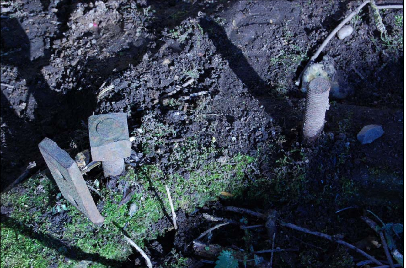
Plate 12. HFDF tower foundations, concrete sill and iron fittings
