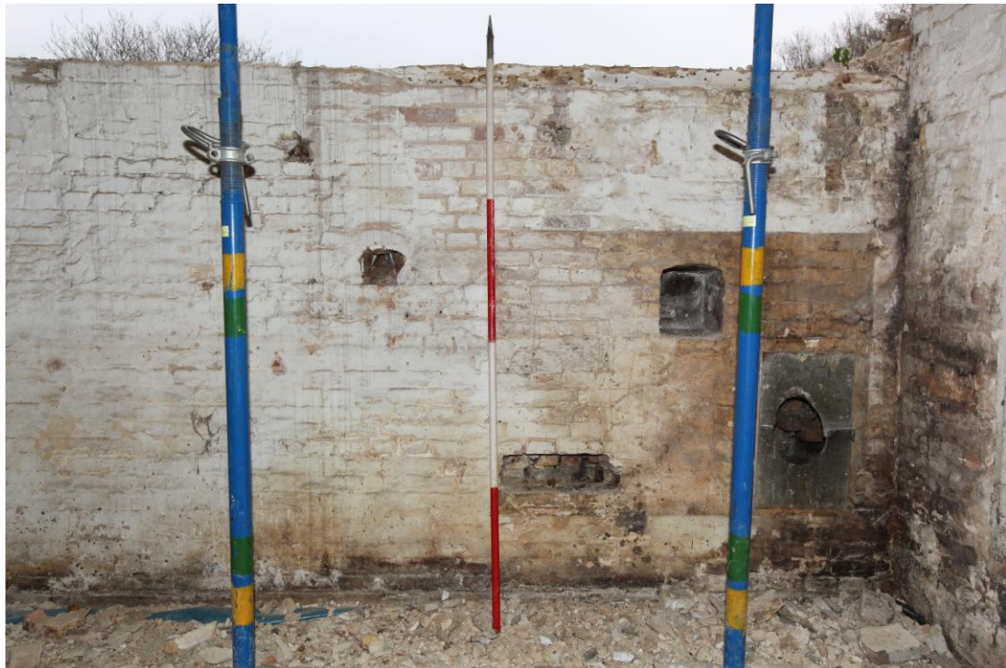
Illus. 6. The eastern half of the northern internal gable showing an original square niche to the right with a secondary metal-lined chute to the left and two additional secondary apertures.
