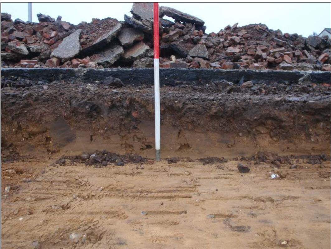
Plate 3. Trench 18, camera facing SE showing the truncation of the natural subsoil (ref. HLR81)
