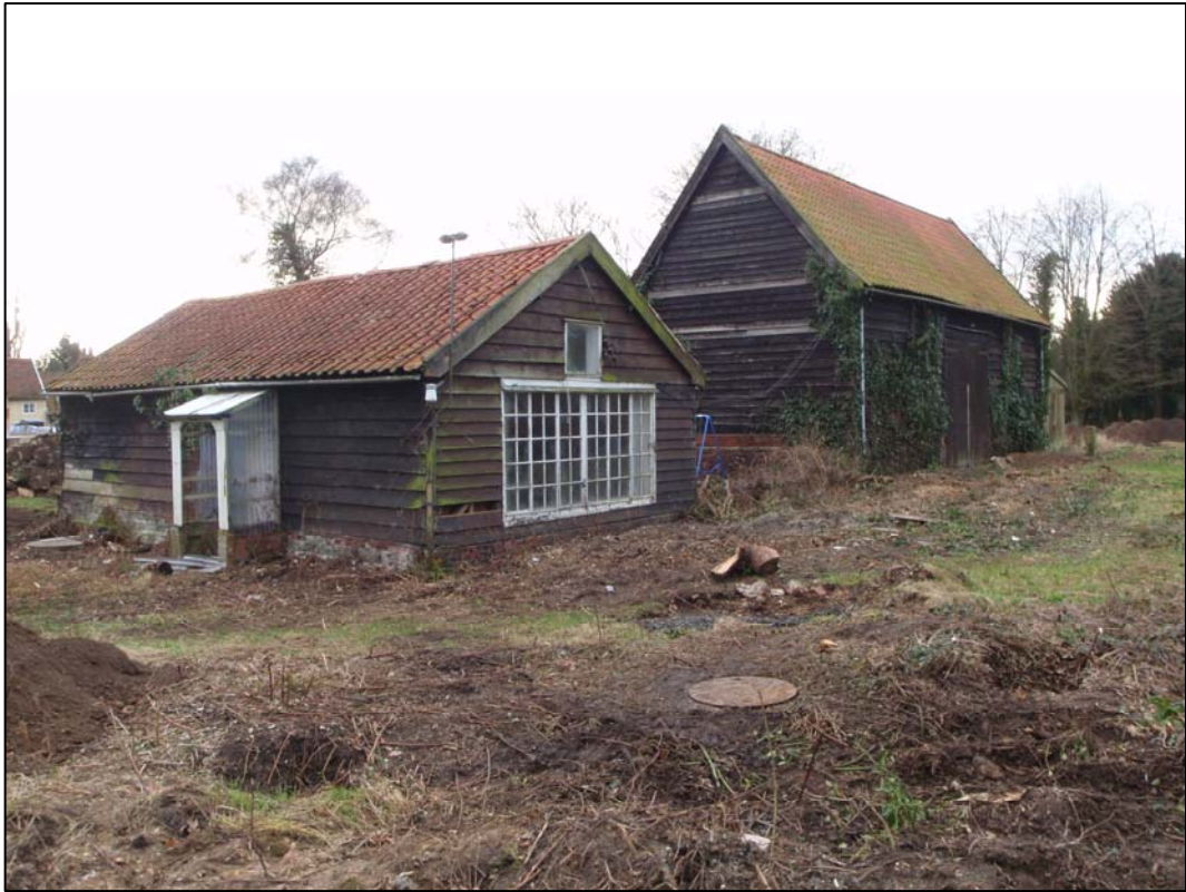
Plate 1. timbered shed and barn, camera facing southwest (ref. HLO21)
