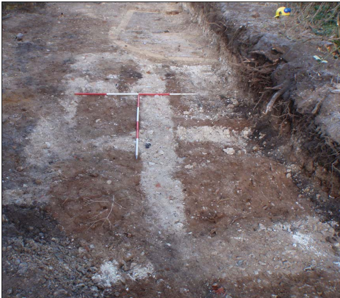
Plate 8. Footings 0115 in foreground, with wall 0114 to rear, facing north-west, 2x2m scale
