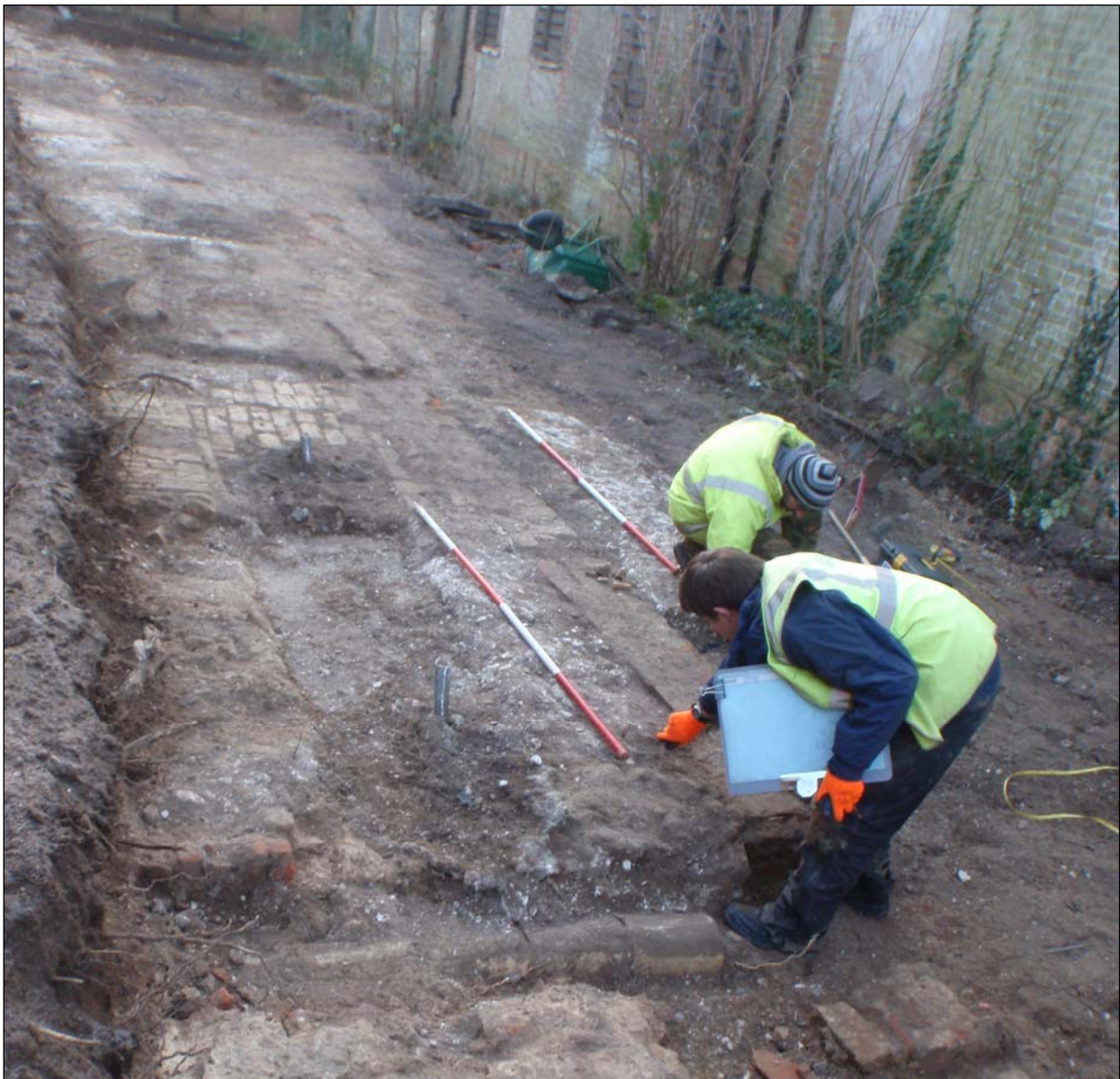
Plate 6. Walls 0105, 0113 and 0112, associated chalk and brick surfaces, and drain trench 0119, facing south-east, 2x2m scales
