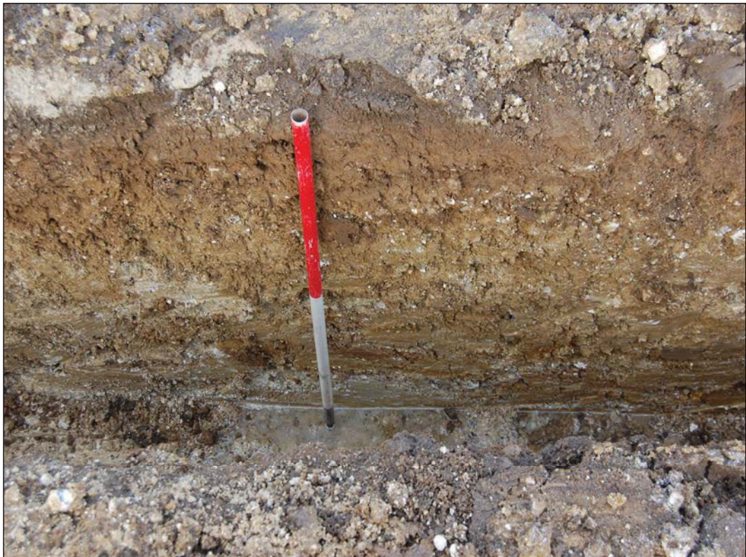
Plate 2. Sample section of pipe trench at southern end of development area, looking north (1m scale).
