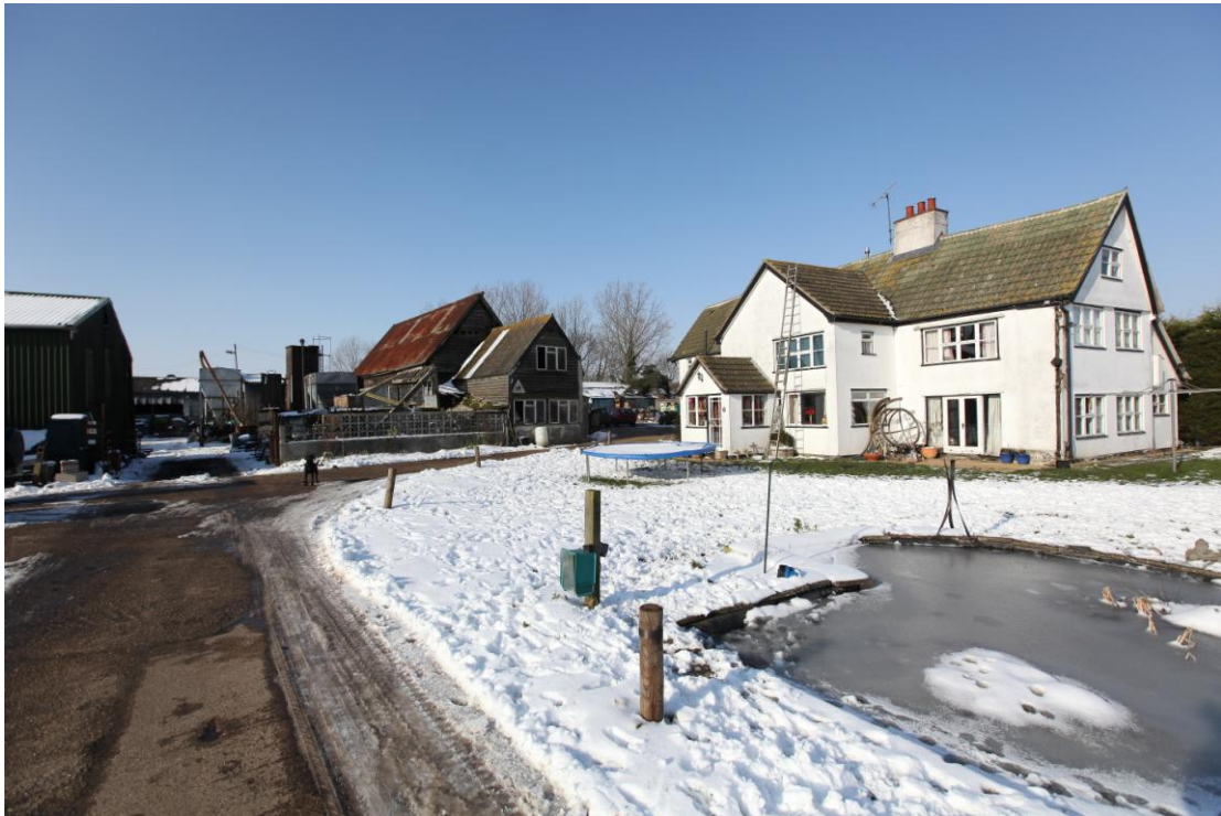
Illus. 1. General view of the site from the entrance track to the east showing the unlisted (but possibly 17 th century) farmhouse (7) to the right and the 19th century barn complex in the centre.
