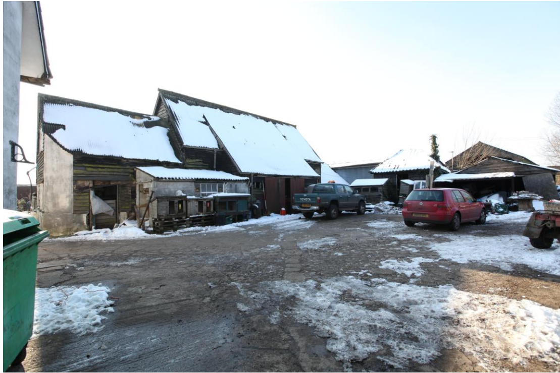
Illus. 3. General view from the north-east showing the detached granary with hipped pantiled roof (4) to the right (surrounded by 20 th century sheds), with the barn (1) and milking parlour (2) to left. The barn's lean-to porch (1a) is an original feature shown on the 1883 Ordnance Survey.
