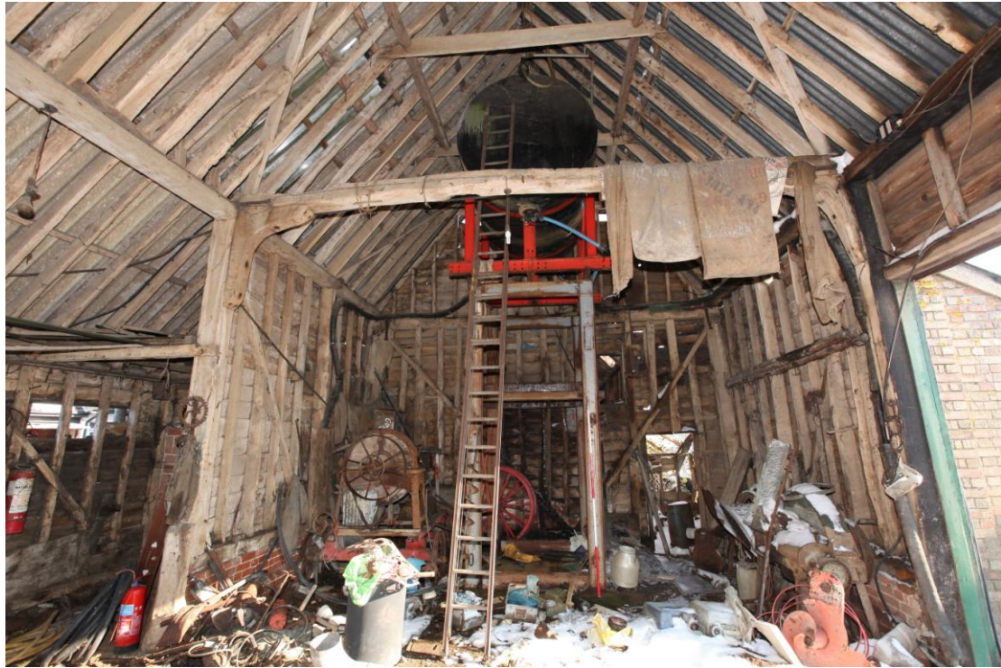
Illus. 5. The eastern interior of the barn (1) showing the original entrance in the central bay to the right and the contemporary lean-to porch (1a) to the left. The collars of the clasped-purlin roof are nailed rather than pegged to the principal rafters.
