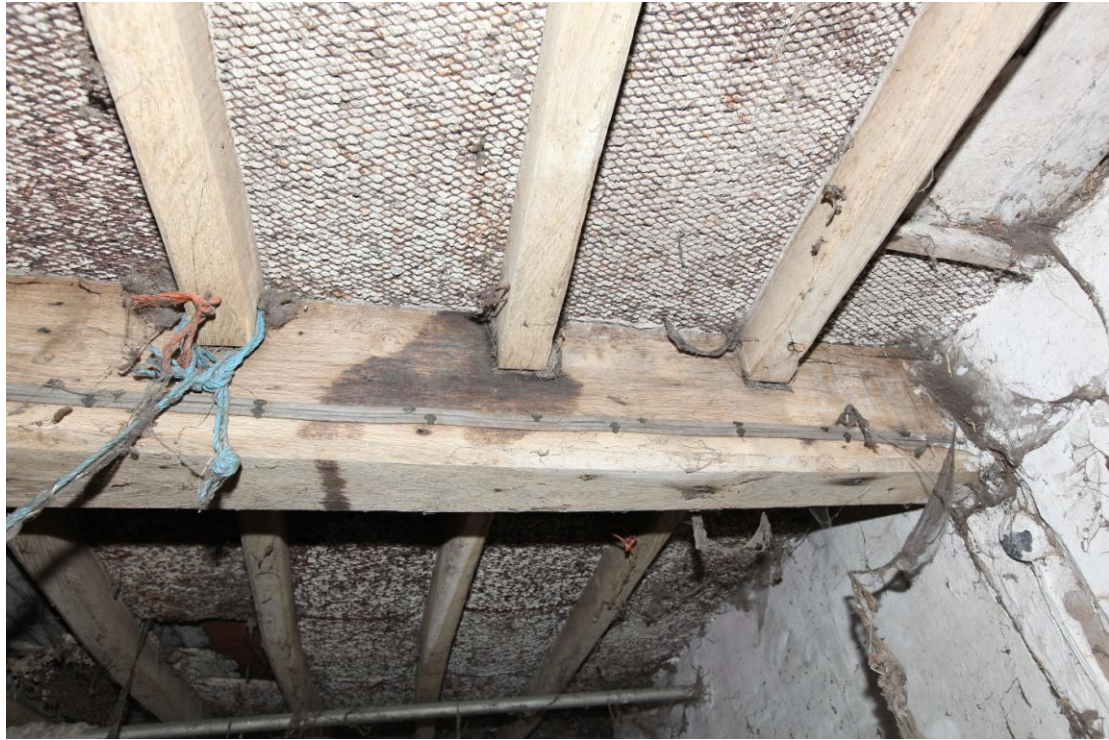
Illus. 7. A detail from the east of the original ceiling in the milking parlour (2) showing its neatly chamfered and stopped tall-sectioned oak common joists. There is no evidence of a hay drop but the original loft boards have been replaced with wire mesh.
