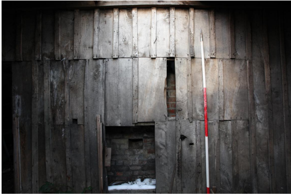
Illus. 9. Detail of boarded partition of forge (B) from southern lean-to (D) showing marks of circular saw and possible blocked hatch behind brickwork of flue.
