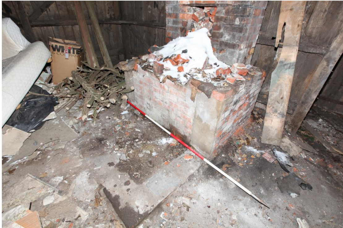
Illus. 11. Interior of forge (B) from north -west showing brickwork of forge against rear wall.
