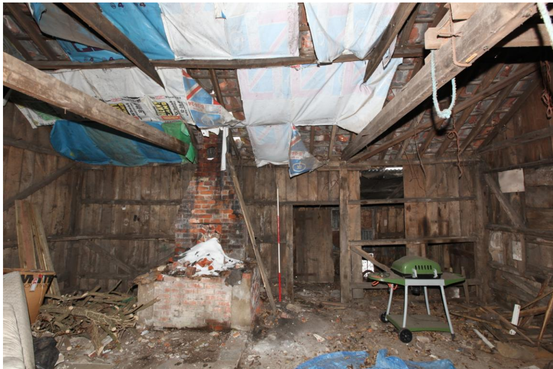
Illus. 10. Southern interior of forge (B) showing brick forge to left and door to rear lean-to (D) to right.
