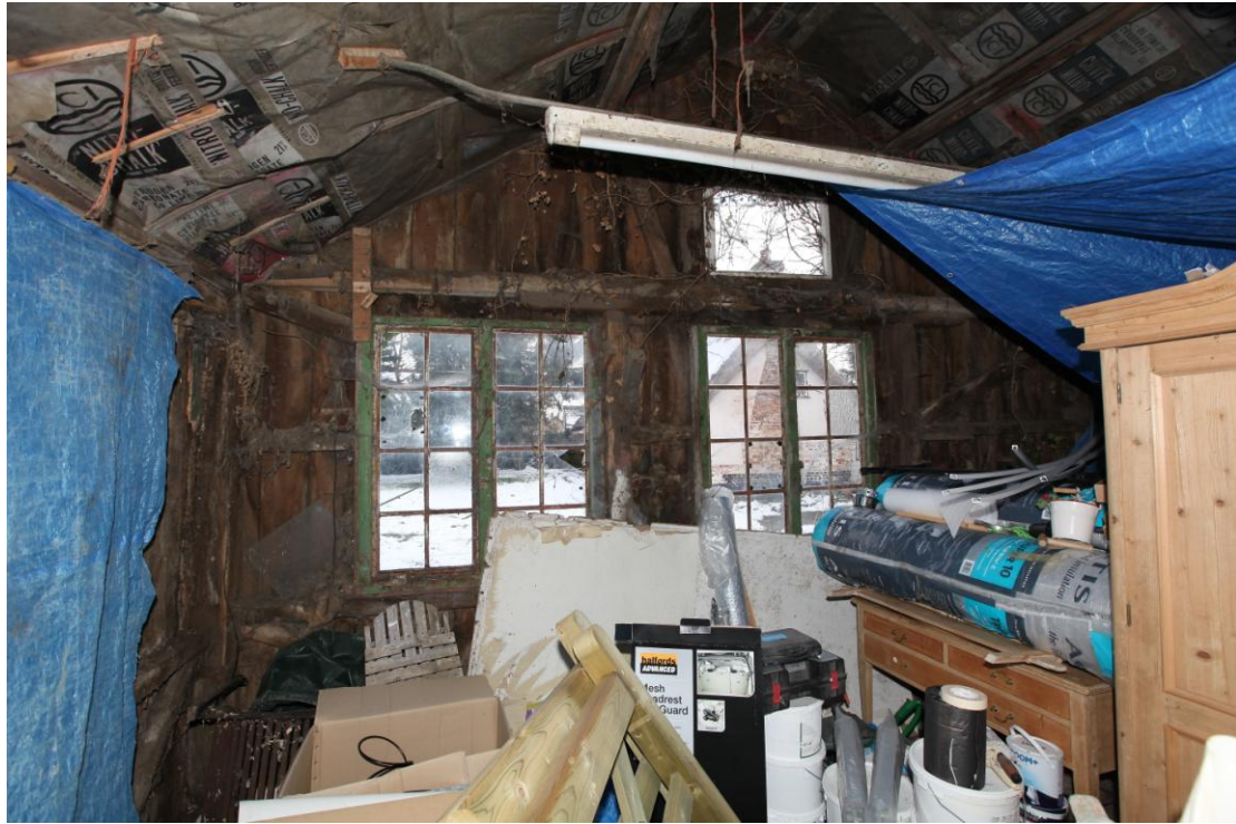
Illus. 7. Internal eastern gable of carpenter's shop (A) showing metal casement windows with red and green paint.
