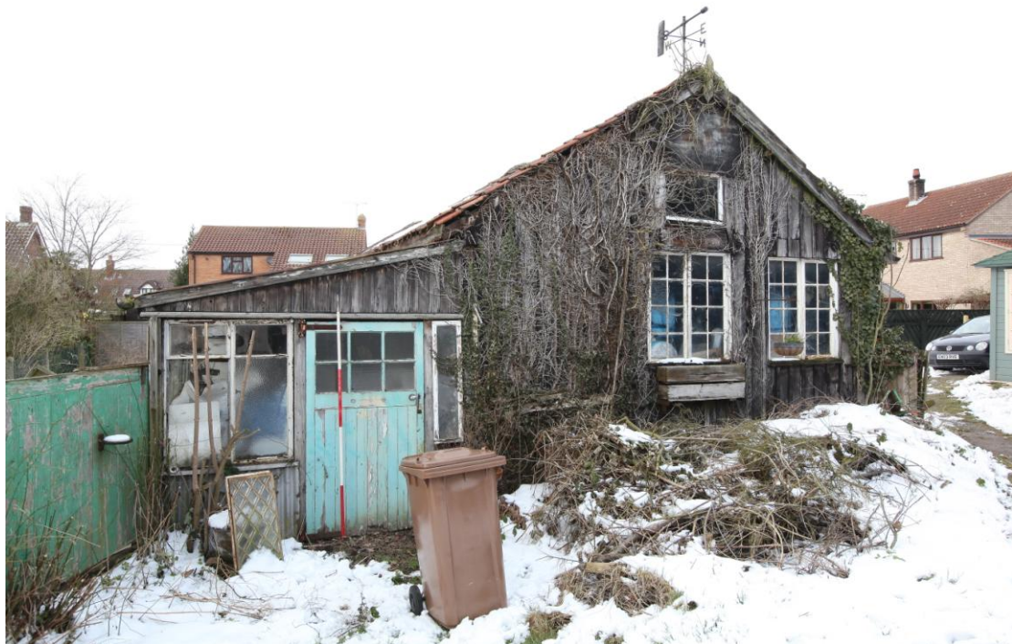
Illus. 6. Eastern external gable showing glazed lean-to shed (C) to left and windows of carpenter's shop (A) to right.
