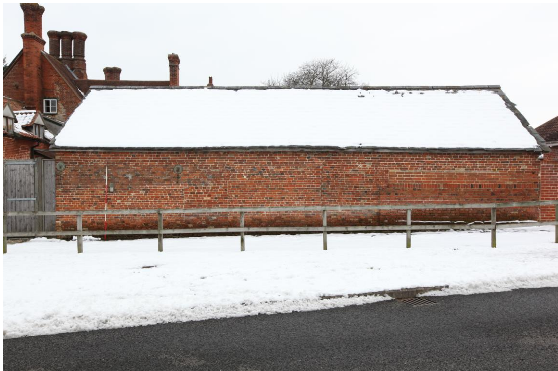
Illus. 2. Rear external elevation showing several phases of brickwork with earliest section to lower right.
