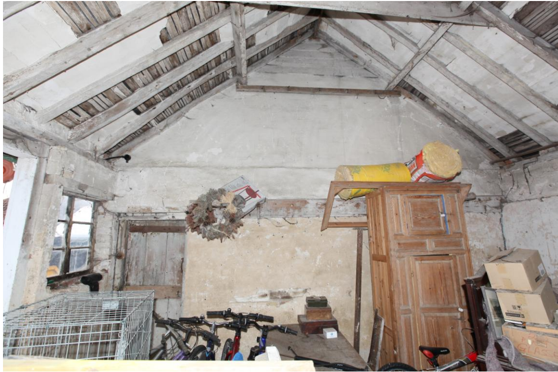
Illus. 9. Interior of central shed (B) from north-east showing internal door to southern shed (A) to left and harness hooks projecting from wooden rail in centre.
