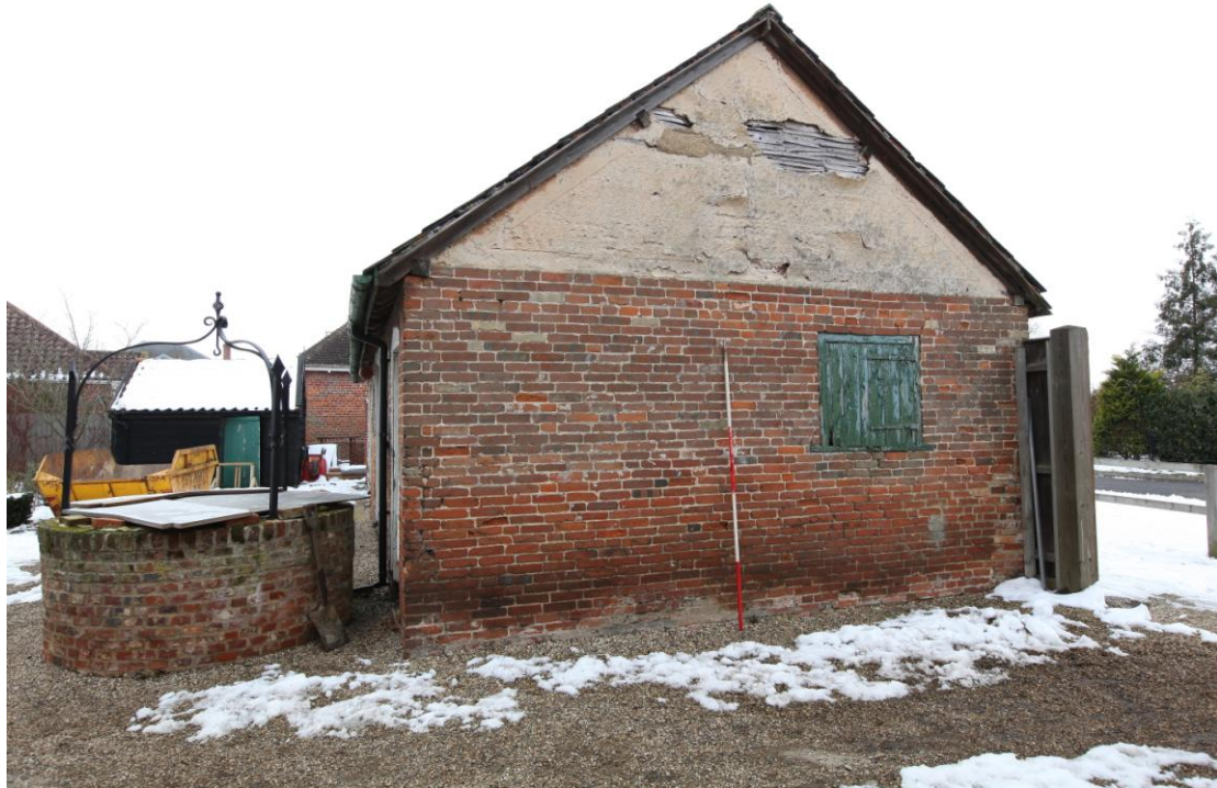
Illus. 3. North-eastern external gable showing secondary hatch and gate to Hill House Lane to right with cable-pattern pargeting to roof gable.
