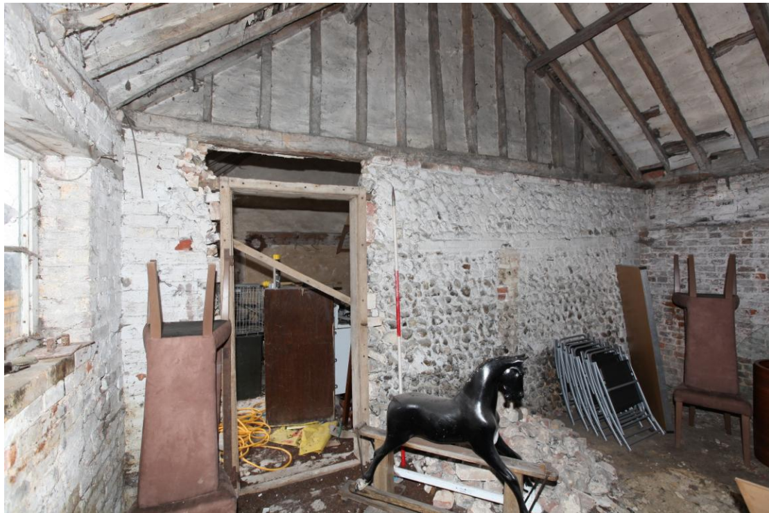
Illus. 12. The interior of the northern shed (C) from the north-east, showing the flint-rubble partition to the central shed (B) with evidence of a 'lift' above the brick course. The present doorway appears to have been inserted recently.
