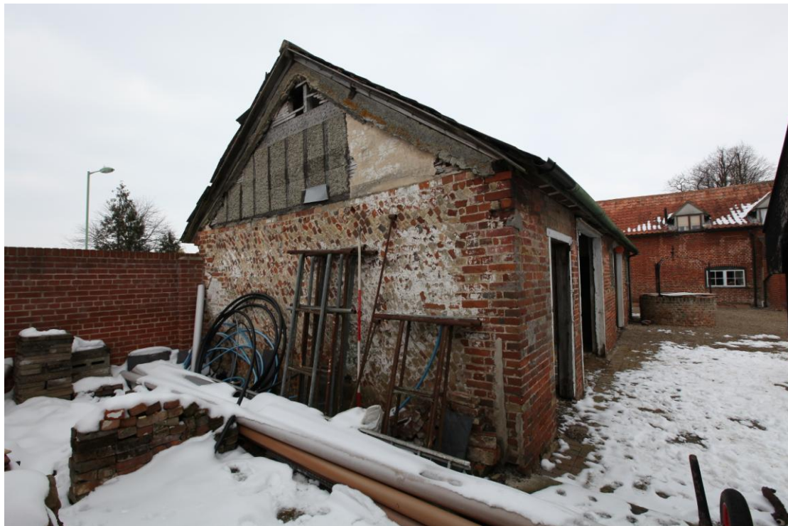
Illus. 6. South-western external gable showing rubble-bond brickwork and fragment of cable-pattern pargeing.
