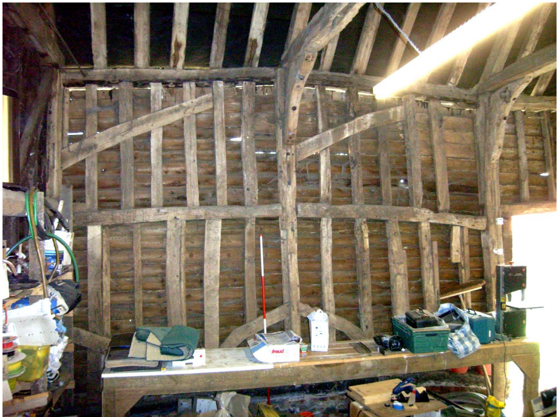
Illus. 8. Internal northern elevation to west of entrance showing symmetrical bracing and the re-used central post of a late-medieval domestic service partition.
