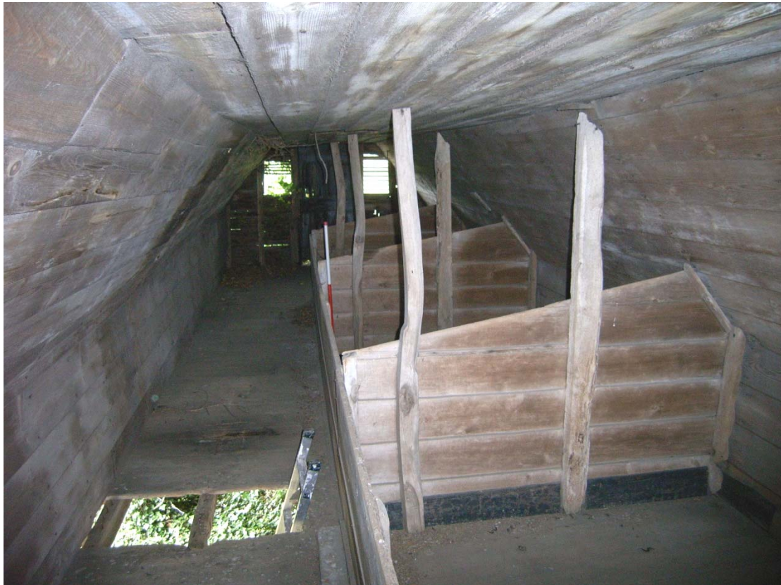
Illus. 4. Interior of granary (6) from east showing good boarded grain bins.
