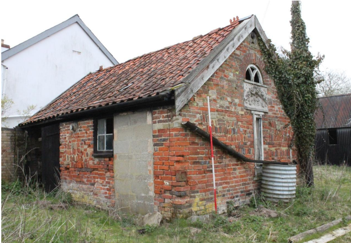
Illus. 3. Exterior from east showing blocked original door to northern shed (1a) with double doors to southern shed (1b) and farmhouse (3) to left.
