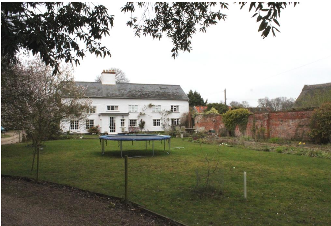
Illus. 2. General view of site from south-east showing facade of farmhouse (3) to left with roofs of dairy (1) and barn (2) to right.
