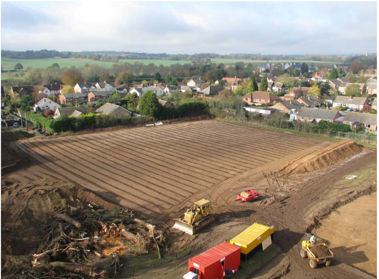
Plate 12. COG 028, backfilled and ready for construction, looking roughly west
