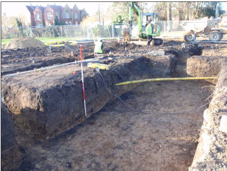
Plate 3. Excavated pads in northwest corner of new building. Looking north west
