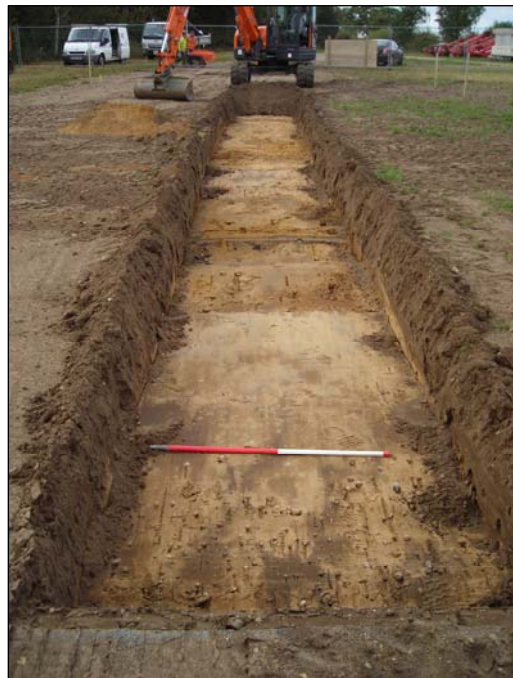
Plate 2. View of Trench 2, looking south west.
