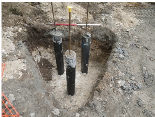
Plate 1. Sample treehouse footing
