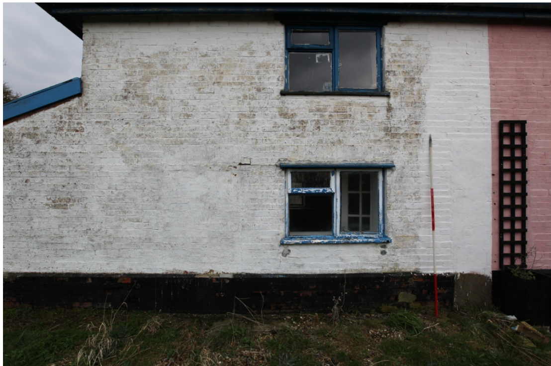
Illus. 4. The western facade of the northern cottage (2) showing the flat brick arches of the 19 th century entrance door to the left and the narrower window above the present 1960s window to the right. The central door of the 1960s conversion (since blocked) is visible to the right but lacks an arch and interrupts the brickwork.
