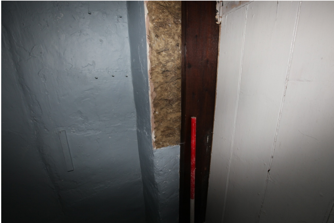
Illus. 9. A detail of the eastern pier of the door to the Bathroom (1) of the southern cottage showing an exposed area clay and straw fabric with no obvious sign of individual blocks.
