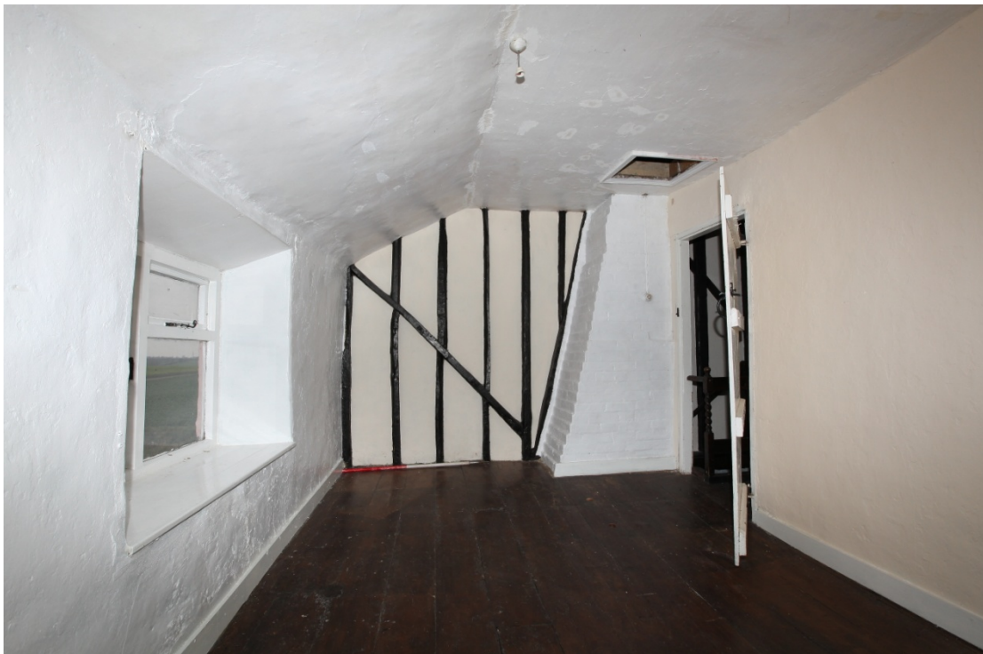
Illus. 10. The front Bedroom (1B) of the southern cottage from the south, showing the 19th century studwork partition to the west of the central chimney and the 0.5 m thickness of the external wall. The 19 th century plank-and-batten door opens onto the Landing (1).
