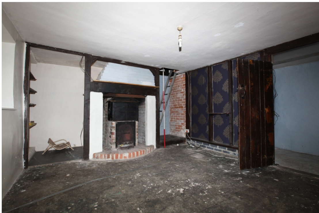
Illus. 8. The southern Living Room (1) from the south showing the 19th century brick fireplace with a recent studwork partition adjoining the Hall (1) to the right. The recess to the rear of the fireplace may have contained a copper as there is evidence of a bread oven to the front (illus 12). The studs framing the chimney are modern.
