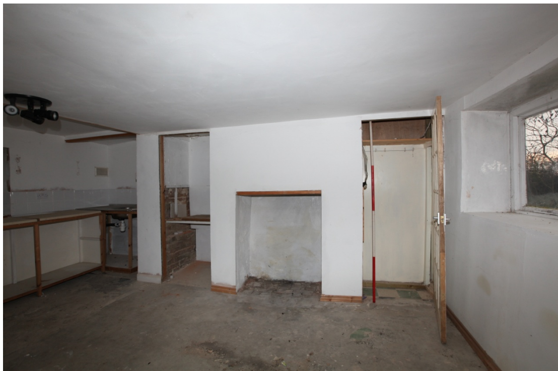
Illus. 6. The Living Room of the northern cottage (2) seen from the north, showing the 0.5 m thick front (western) wall to the right and the rendered fireplace with an exposed area of 19 th century brickwork to the left. A fragmentary shelf and a small original aperture in this brickwork probably indicate the position of a bread oven to the rear of the main fireplace.
