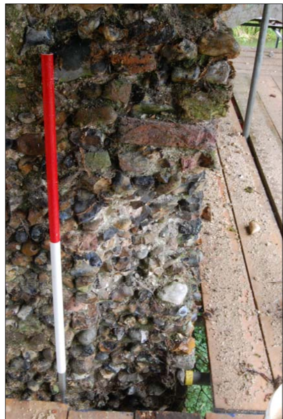
Plate 12. Rebated section in the NE corner of the NW corner tower (T5) possible setting for vertical wall post. 1 x 1m scale
