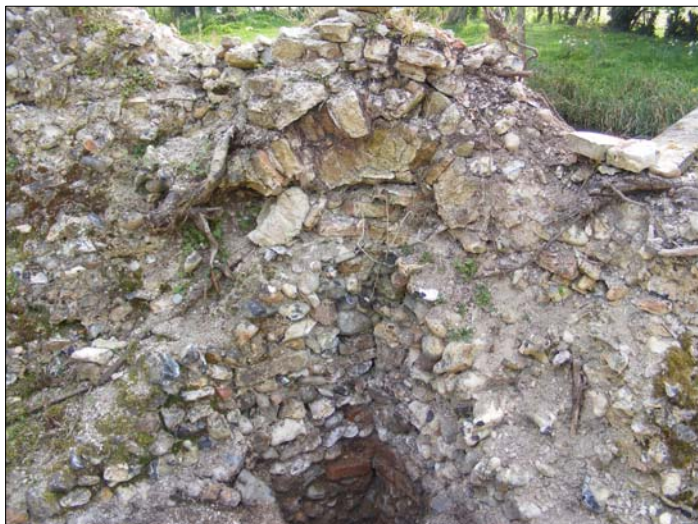
Plate 26. Brick squinch internal corner of the south curtain wall's west tower
