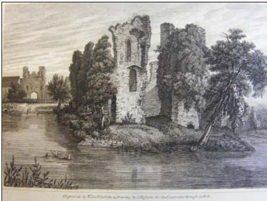
Figure 11. An engraving of the SW tower published in 1819 from a drawing by I. Higham. Note the entrances to the stairwell intact and the corbelled vault above the first floor to support the top half of the stairwell, also what appears to be a revetment to the moat island at the water's edge and drain outlet at the base of the mid tower (Ips. RO ref HD1678/97/2)
