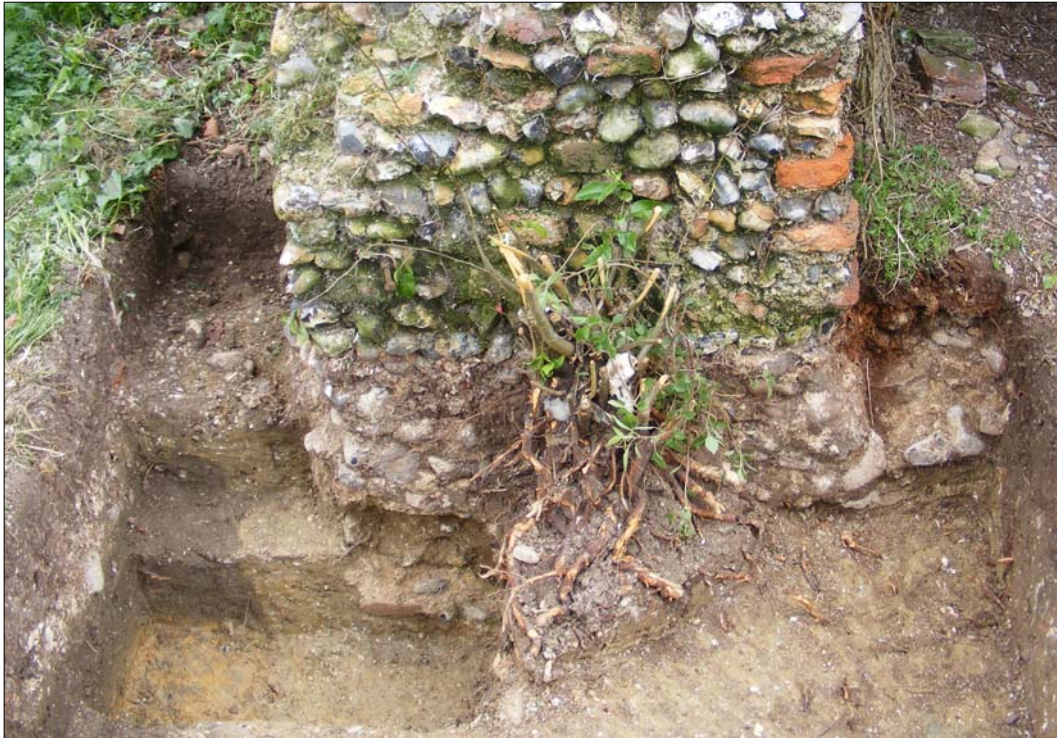
Plate 10. Foundation below NW corner of Mid-tower(T4) showing green clay packed trench cutting buried medieval topsoil. The brick quoin to the right is the edge of the west door opening; the lowest brick indicates ground level. Note bonded flint footing extends across the opening.
