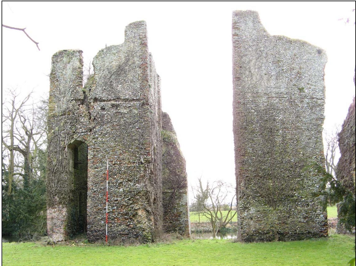
Plate 4. North side of the mid and SW corner towers (Towers 4 and 5) with the remains of the south curtain wall between them. The arched head of the ground floor door has collapsed giving the appearance of one elongated opening. Stair turrets project from the top of the inside corner on both towers. 1 x 4m scale
