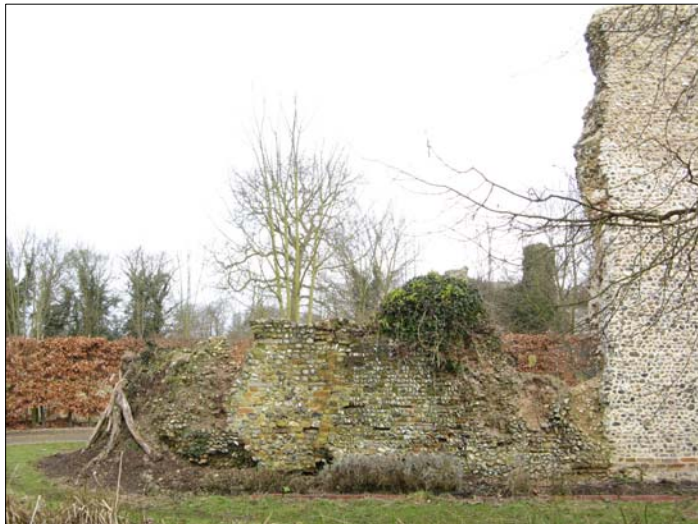
Plate 25. Vestigial remains of the corner tower at the west end of the south curtain wall
