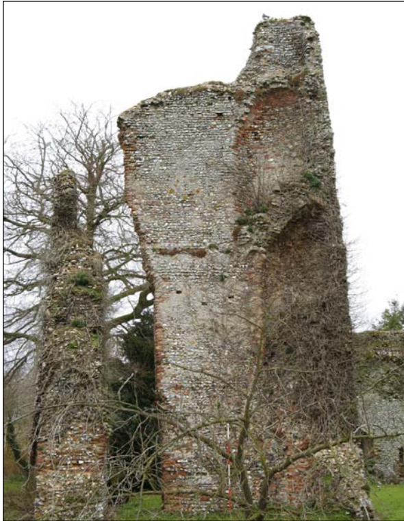
Plate 6. SW corner tower (T5). Interior of the north wall viewed from the south, showing spiral stair well and projecting stair turret above .
