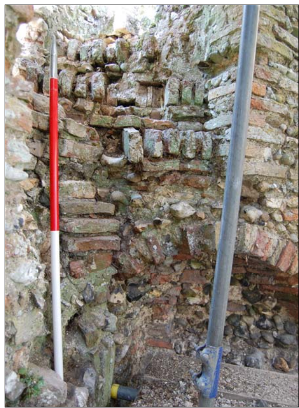
Plate 9. Mid tower (T4) Spiral stair to the roof underpinned by an arched vault across the NW corner of the tower. 1 x 1m scale
