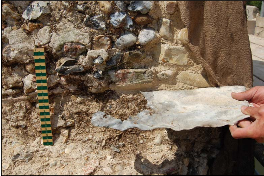
Plate 16. Lead flashing at the base of the parapet of the west curtain wall (15). 1 x 0.3m scale
