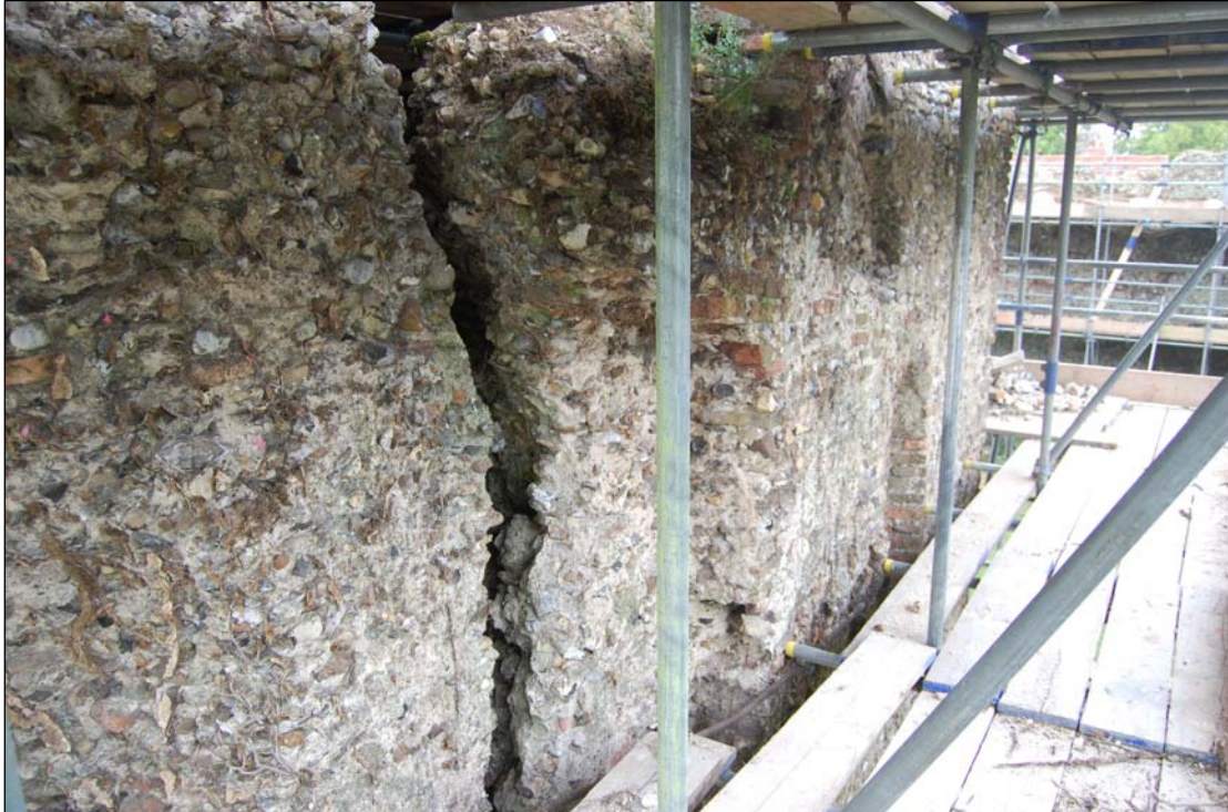
Plate 22. Stepped east face of the mid tower (T4), showing the south half of the wall face recessed back from the plane of the north. The recessed section enables a door to be opened flush to the wall.
