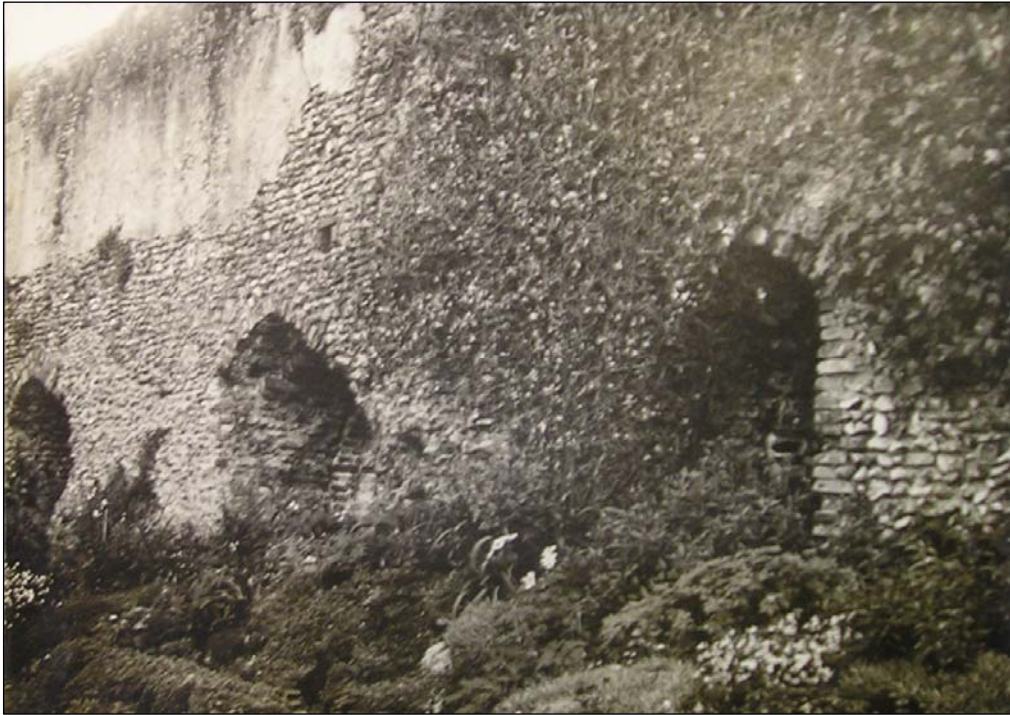
Image 6. Interior of the north curtain wall (1954)
