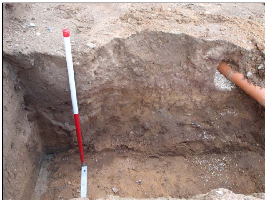
Plate 1. Central footing, looking south
