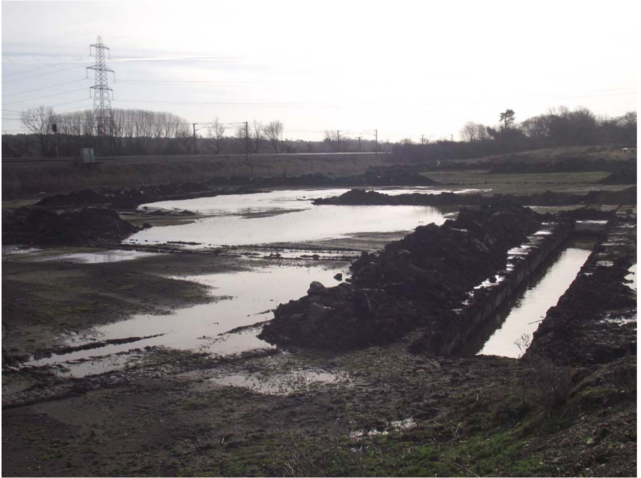
Plate 1. View of site looking east showing waterlogged trenches and wet conditions
