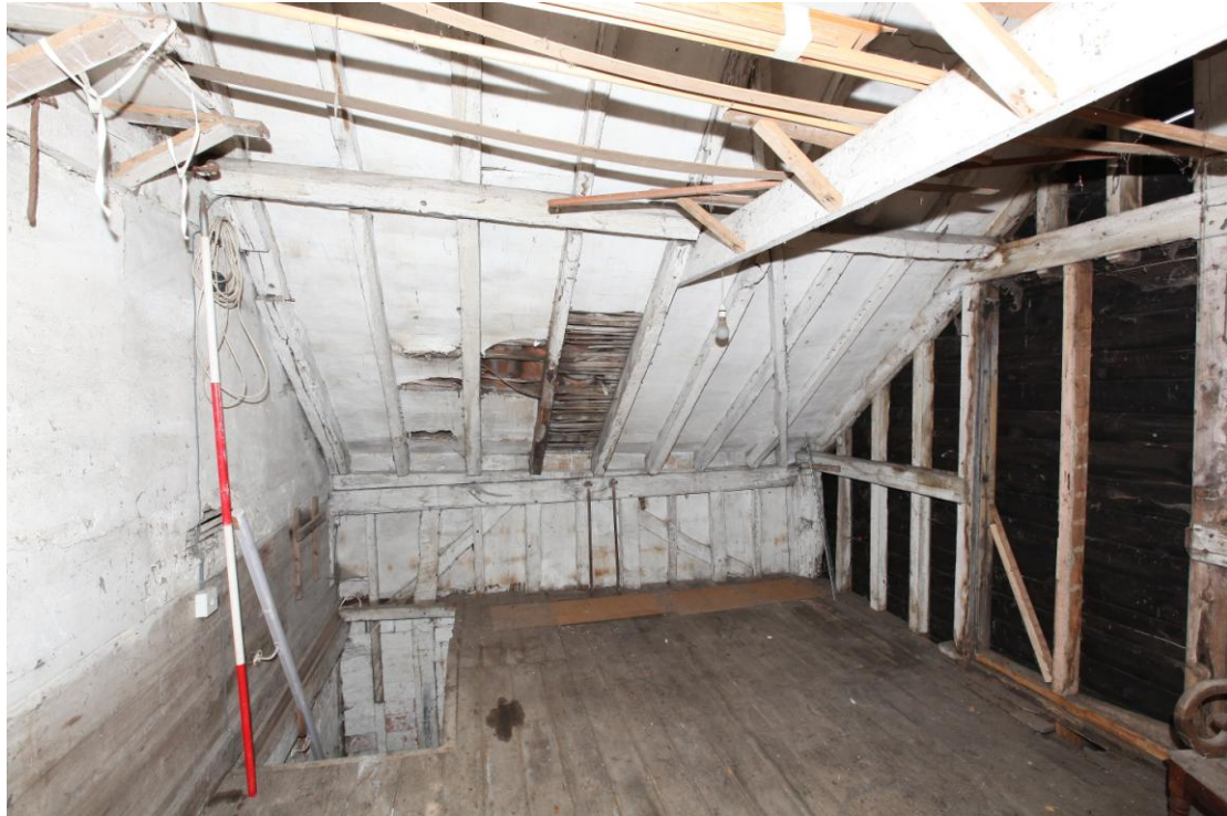
Illus. 13. The eastern interior of the loft above the southern bay (A) showing the 19th century whitewashed roof and rebuilt southern gable with a blocked original (19 th century) external door in the southern gable to the right. This door would have been reached by an external stair and suggests the loft operated as a granary. The apotropaic (i.e. evil-averting) symbols in illus. 14 below are on the internal plaster wall to the left.
