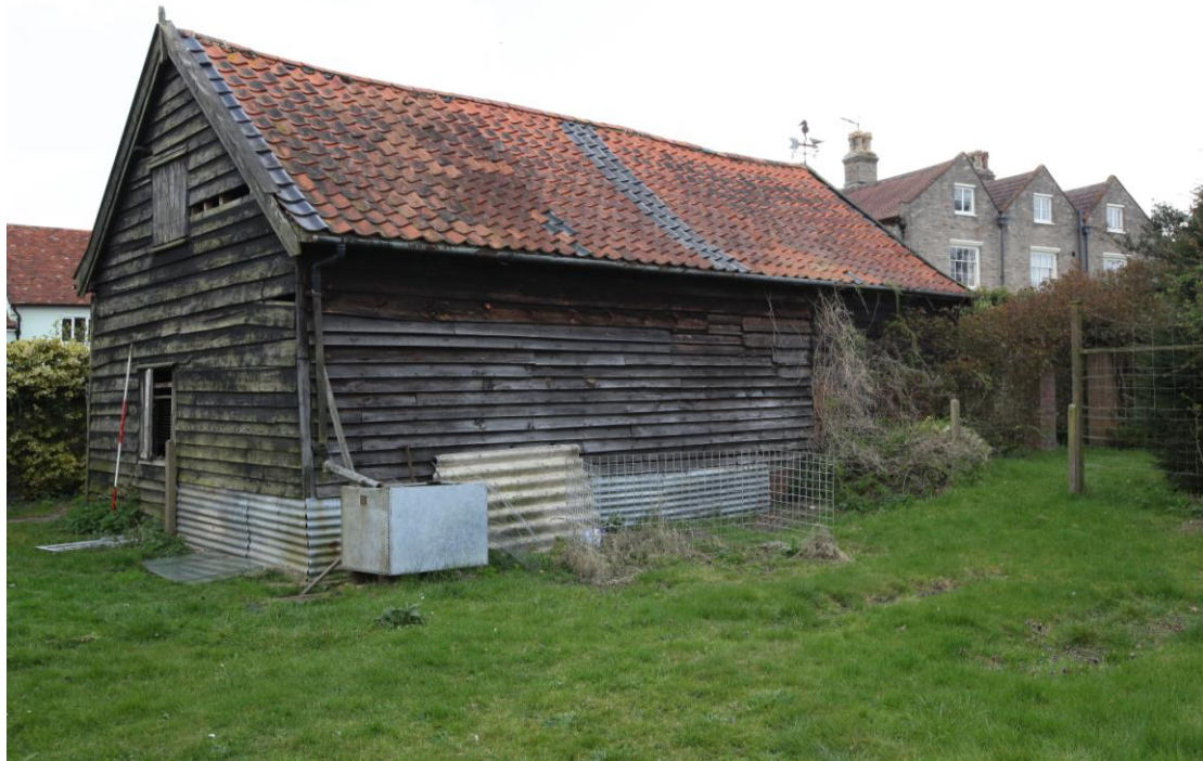
Illus. 3. The barn from the north-west showing its proximity to the rear gables of Hill House to the right. The glazed window and hatch of the northern gable to the left date are 19 th century insertions and much of the weatherboarding was renewed in the 20 th century. The small central doorway to the threshing bay (B) has been blocked.
