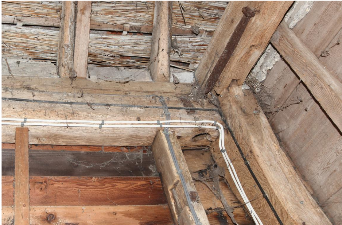
Illus. 11. A detail of the eastern roof-plate in the central bay (B) showing the cylindrical housing for the pin hinge of the original barn doors to the right. An identical feature lies to the left of the bay. The studwork beneath is modern.
