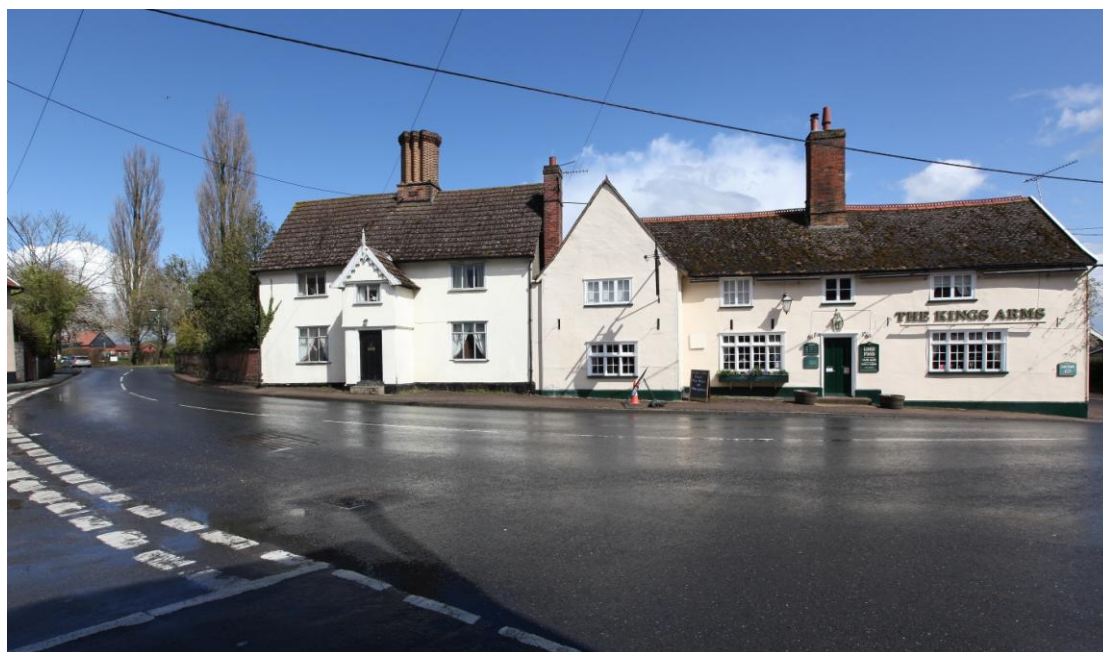
Illus. 1. The western facade of Glebe House (left) adjoining the junction of Duke Street and Bacton Road with the King's Arms to the right. The southern gable of the barn is visible behind the trees to the left of the house. The date 1611 in 20th century ironwork is attached to the front of the chimney but the present 'lobby entry' layout of the building is likely to be later.
