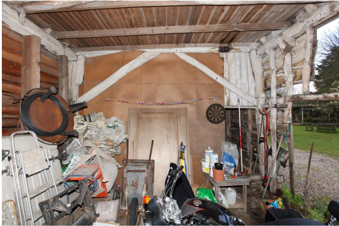
Illus. 5. The interior of the central bay (B) from the south showing the intact arch-braced open truss adjoining the secondary partition of the northern bay (C).
