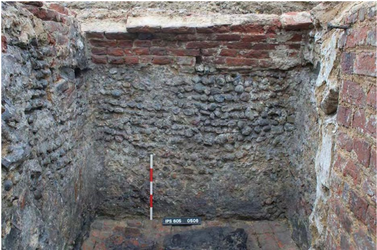
Plate 7. Vaulted chamber at the NW corner of the 'merchant's house' (0.5m scale)
