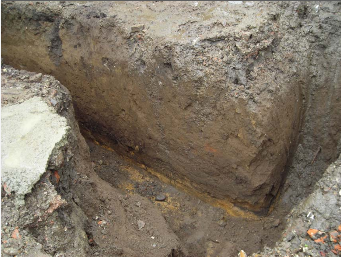
Plate 2. Oblique view of the central footing, looking south west
