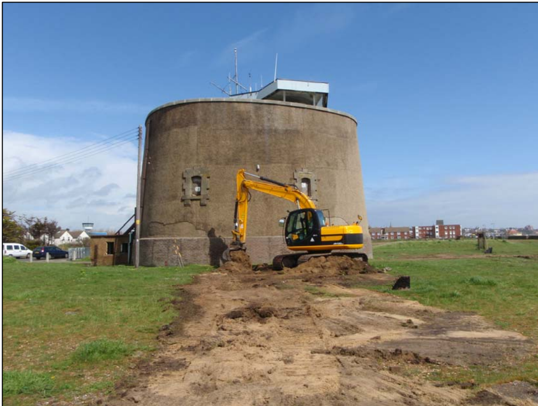
Plate 37. Backfilling of Trench 7
