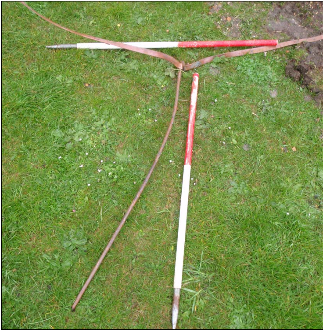
Plate 15. Trench 10, copper strip and copper coated earthing rod (ref. HPK57)
