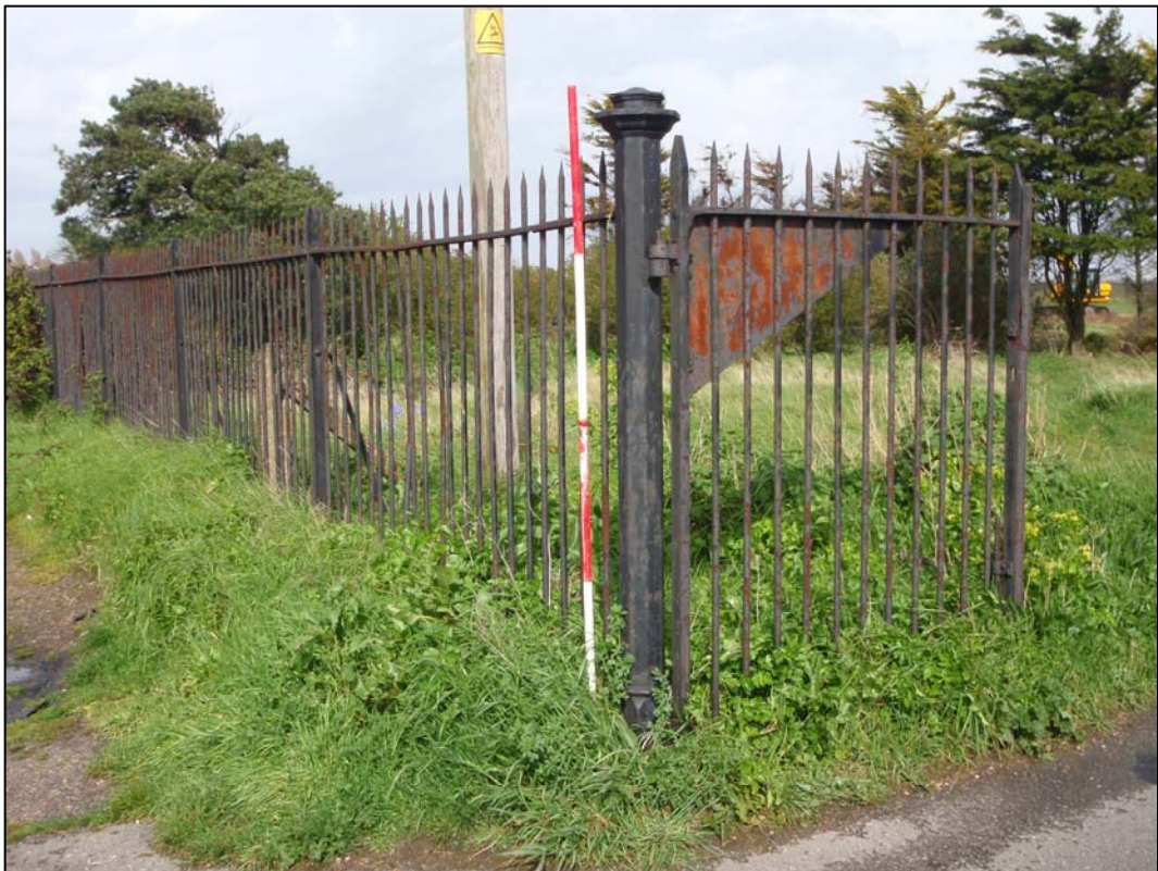
Plate 6. section of fence and gate adjacent the entrance (ref. HPL046)
