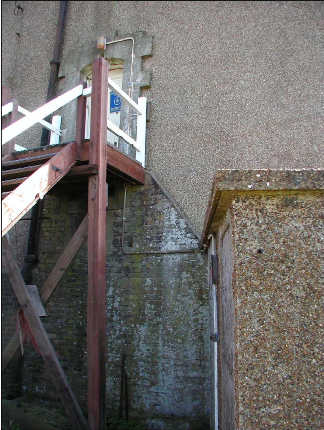
Plate 33. Area of what is probably the original brick facing at the rear of the tower
