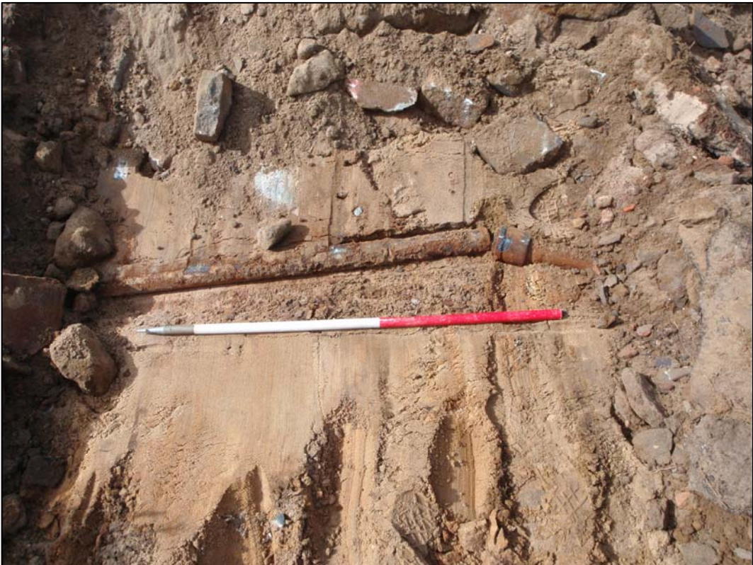
Plate 2. Trench 1, cast iron cable duct (ref. HPK01)
