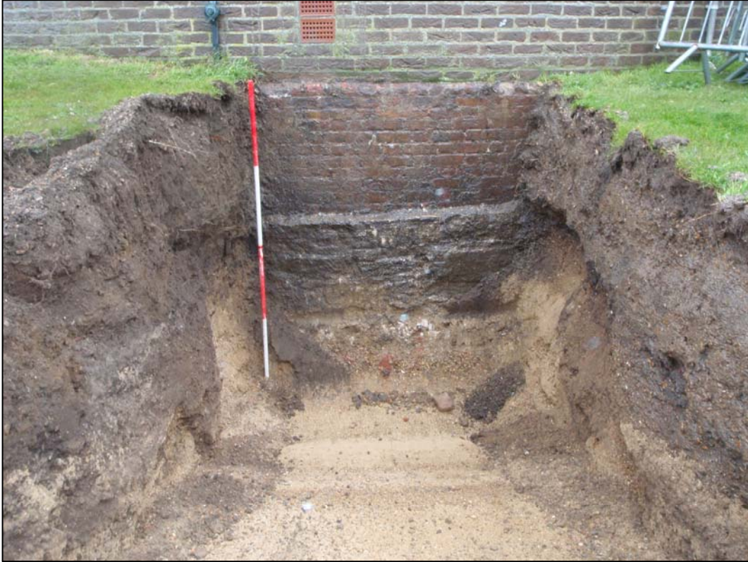
Plate 21. Trench 10, below ground wall and footing of the Martello Tower (ref. HPK53)
