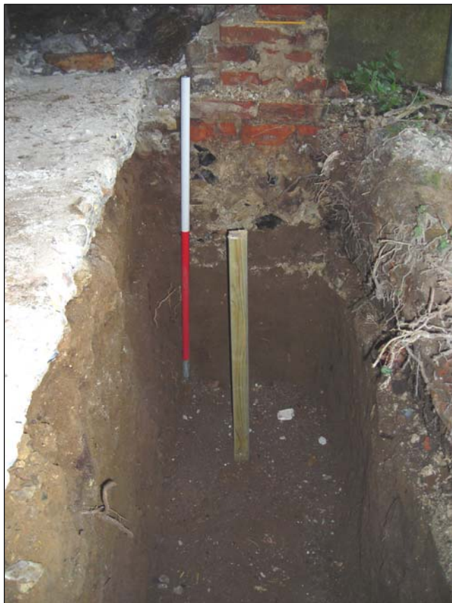
Plate 1. Section through existing footing in the western wall of the barn
