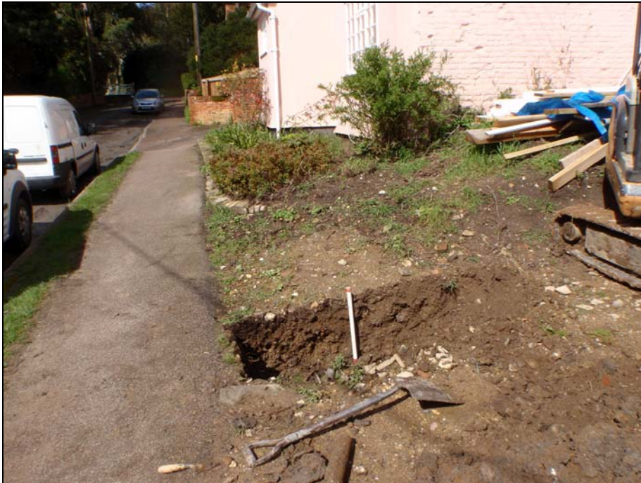
Plate 3. Test trench across possible ditch, facing west.
