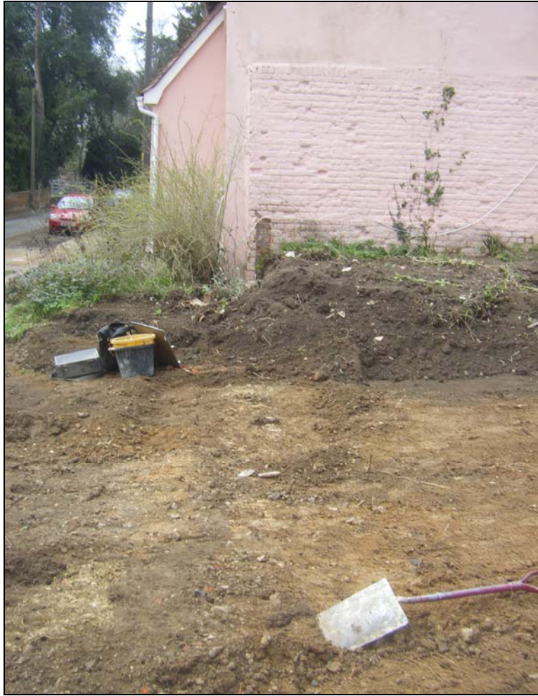
Plate 2. Foundation closely aligned with Grade II listed building, facing west.
