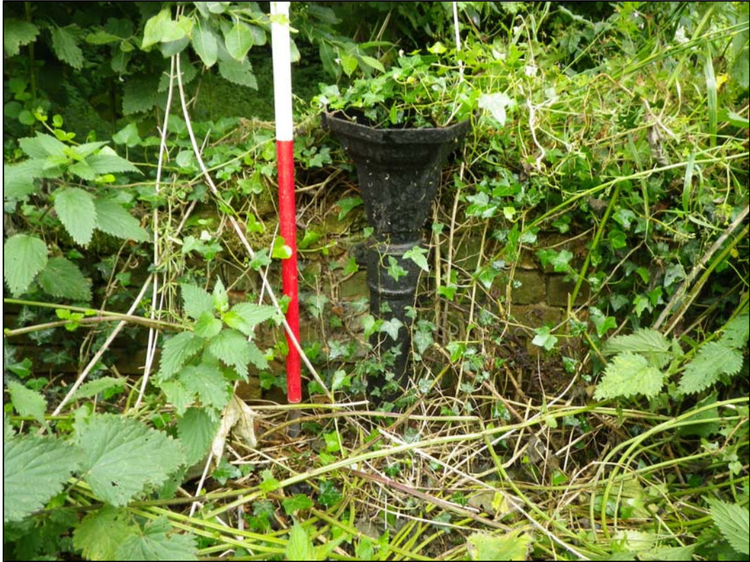
Plate 3 rainwater down pipe (ref. HLW 67)
