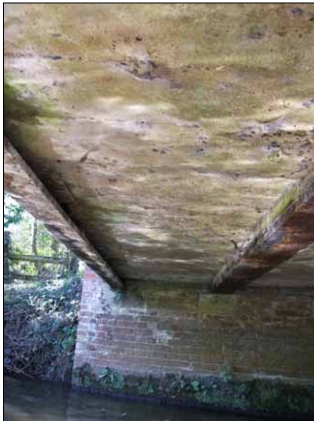
Plate 3. Underside of Scotland Street bridge
