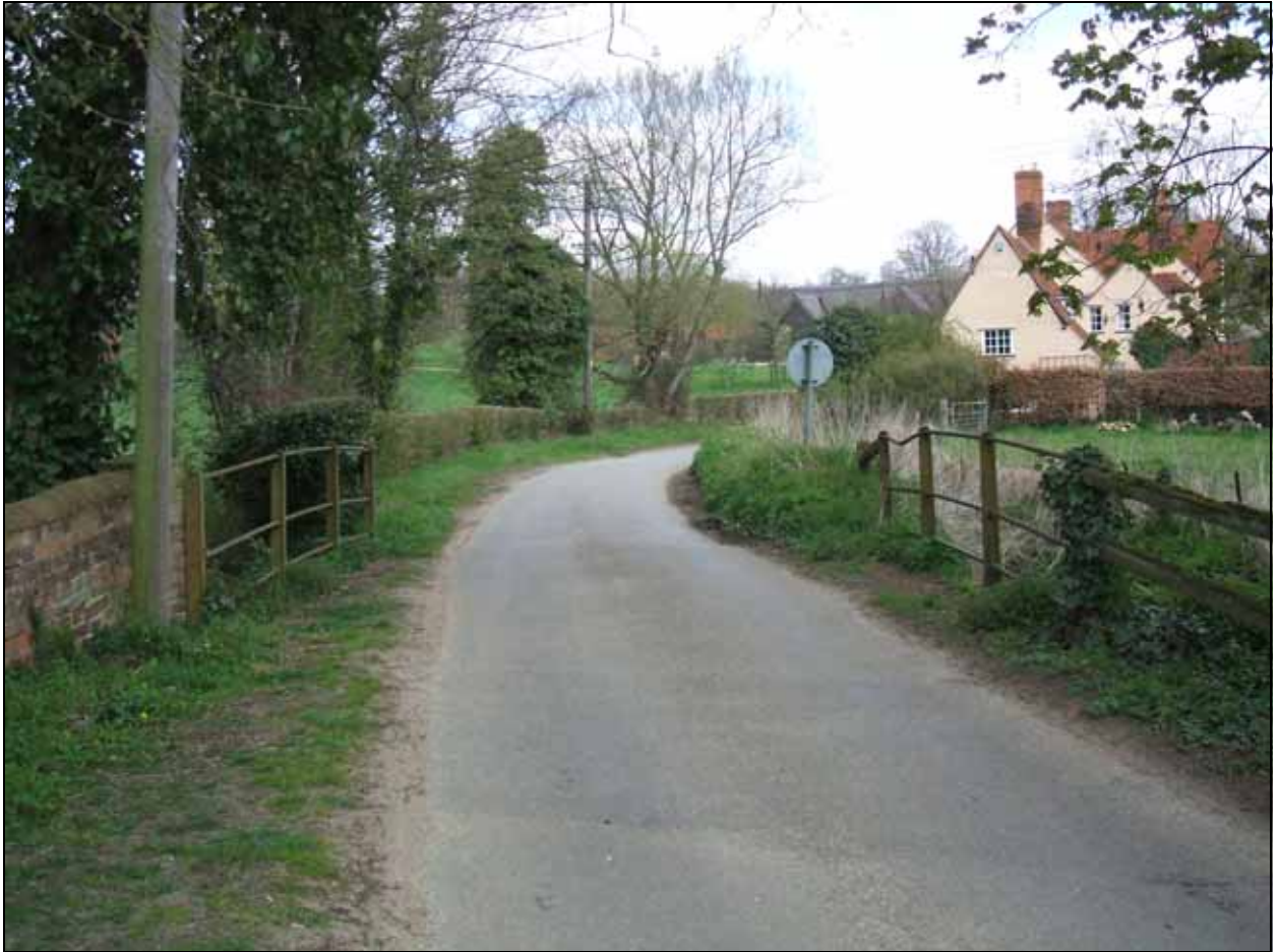
Plate 2. Scotland Street Bridge, looking east.
