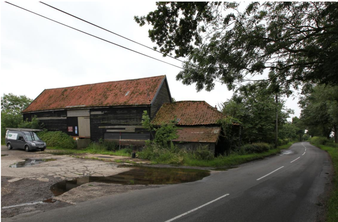
Illus. 1. A general view of the site from the north showing the rear elevations of the weatherboarded and pantiled barn (1) and cart lodge (2) at right-angles to the road between Mendlesham and Stowmarket.
