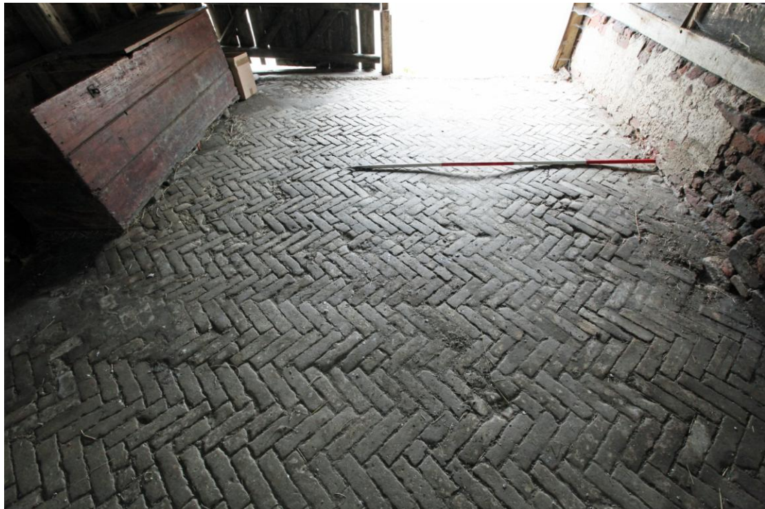
Illus. 8. A detail from the north of the exceptionally fine and complete original herringbone-pattern threshing floor of gault brick showing the painted deal 19 th century grain bin to the left. Several small apotropaic circles survive on the internal weatherboarding to the right.
