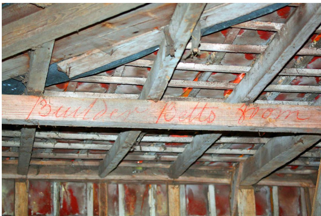
Illus. 12. A further detail of the red-ochre inscription on the underside of the barn's southern purlin. No. 17 of 20 photographs: 'Builder Betts from' (Stowmarket). (Slightly enhanced in Photoshop.)
