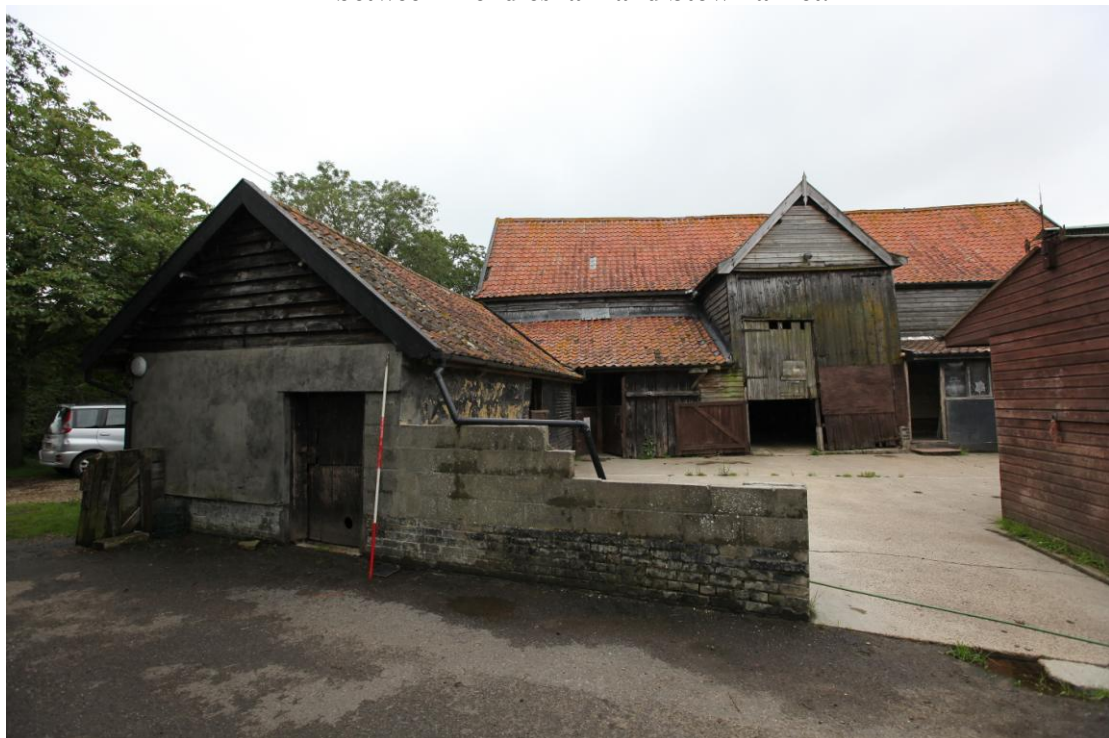
Illus. 2. A general view of the barn (1) and enclosed yard from the south-west showing from left to right the brick and clay-lump cattle shed (3), the lean-to loose boxes containing re-used charred timber (4), the barn's original entrance porch and the modern cement-block office (5). The timber-clad structure to the extreme right is a modern stable range.
