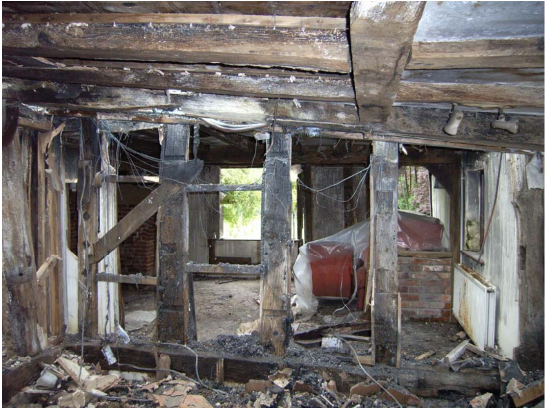
A2.9 Elevation J-G from west showing infill trenches and a window sill or lintel re-used as a stud to left (with original brace attached). Former door and stair trap to right.
