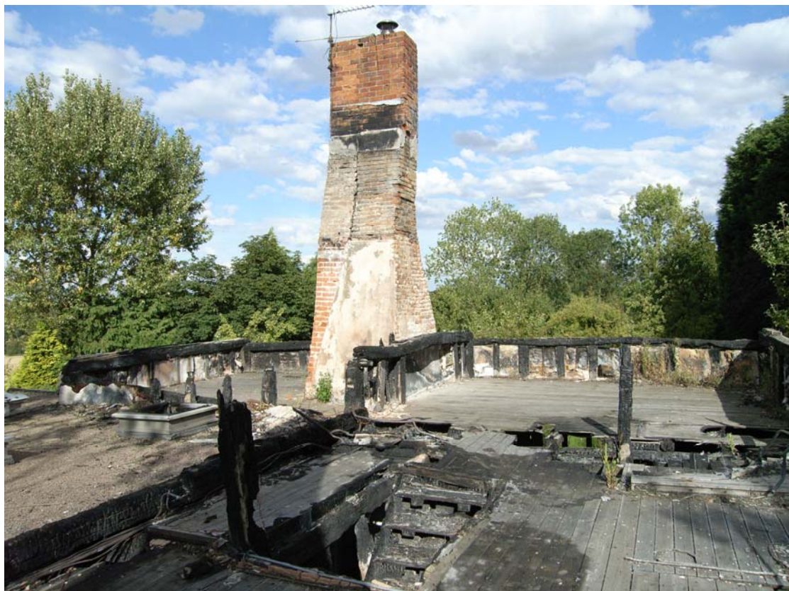
A2.4 Upper storey of structure G-H-M-N from west showing 17 th century chimney to right with secondary chimney to left.
