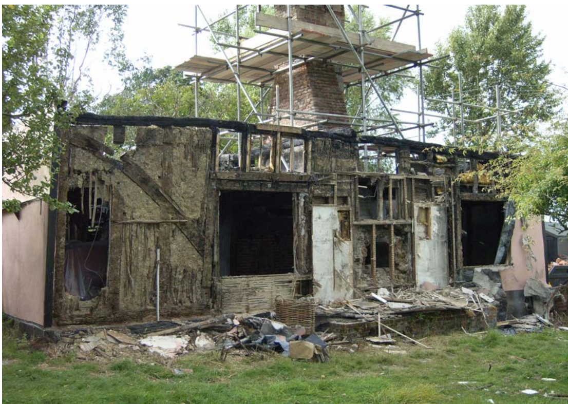
A2.2 External elevation H-N from south-east after commencement of demolition, showing original brace to left and infill of wattle-and-daub attached to externally trenched laths. A secondary bread oven against the eastern side of the chimney formerly projected beyond the plane of the wall.
