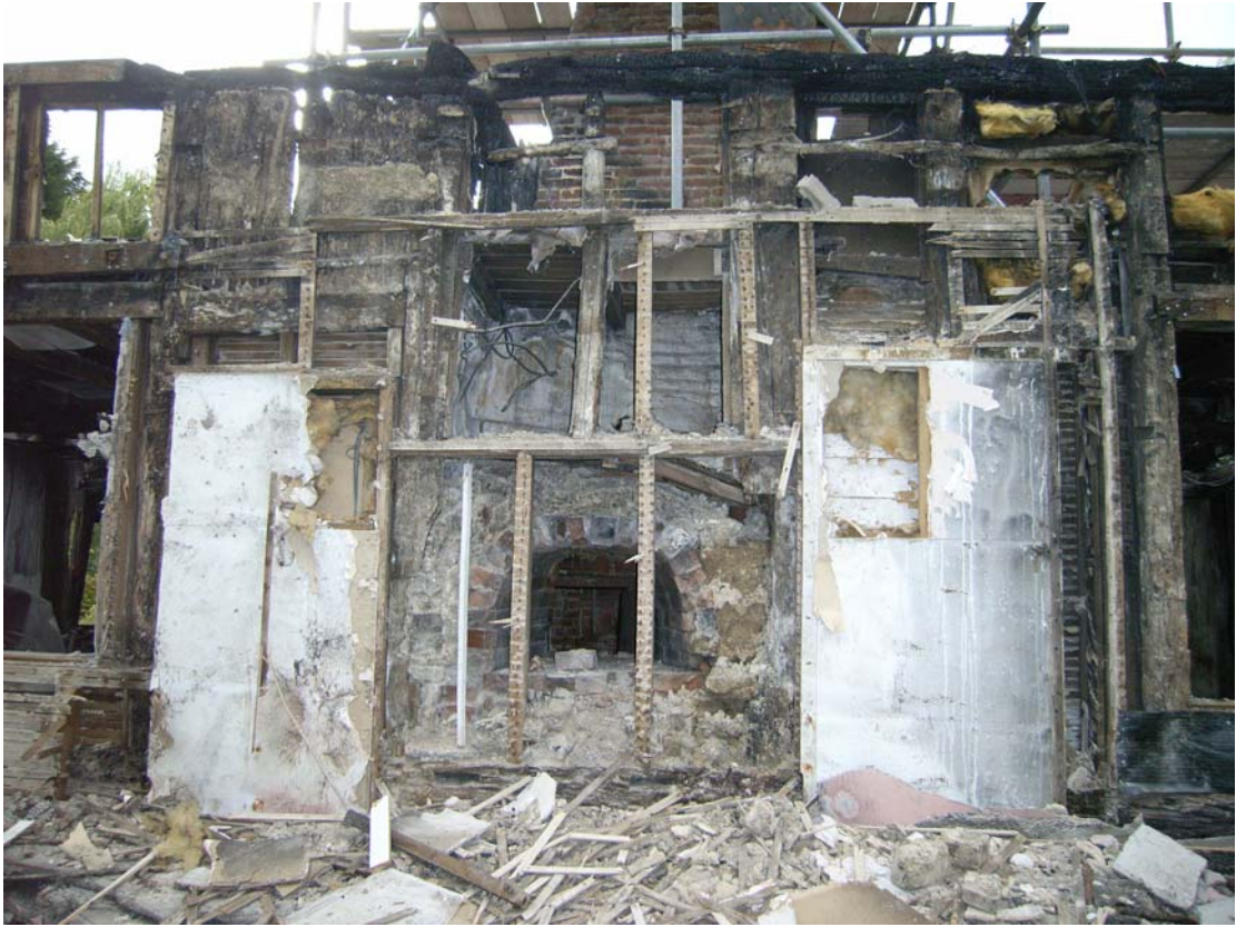
A2.7 Detail of external elevation H-I from east showing truncated brick oven between posts I and J in centre
