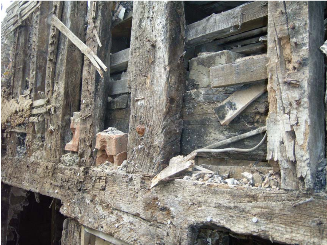
A2.11 Detail of external elevation A-E from south-east showing externally weathered studs with notches for infill staves (in contrast to infill of structure G-M-H-N).
