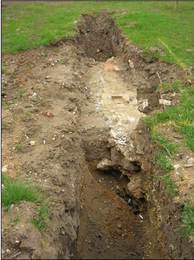
Plate 1. Foundation 0003, looking west, after initial excavation of trench.
