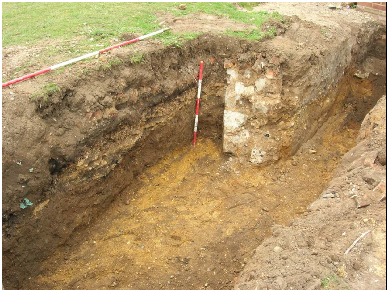
Plate 2. Section 0018 and cross-section of 0003 foundation, facing north-east (2m scale horizontal, 1m scale vertical)
