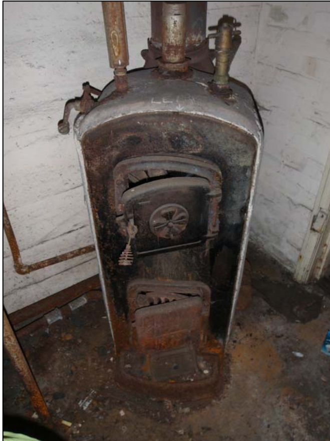
Plate 44. Room B5, solid fuel heater, camera facing east (ref. HLX 70)
