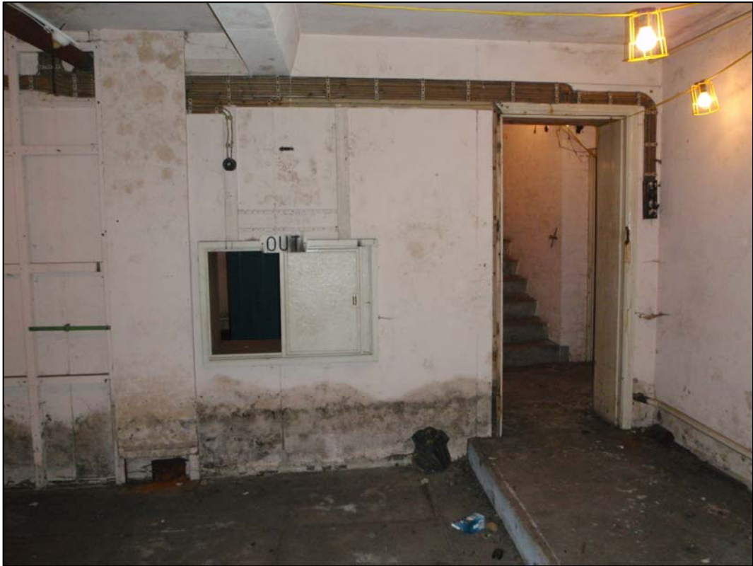
Plate 34. Room B2, hatch through to B3, camera facing south-west (ref. HLX 79)
