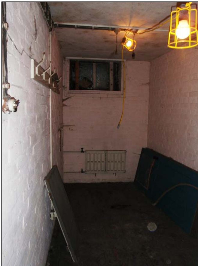
Plate 21. Room G9, camera facing south-east (ref. HLX 52)
