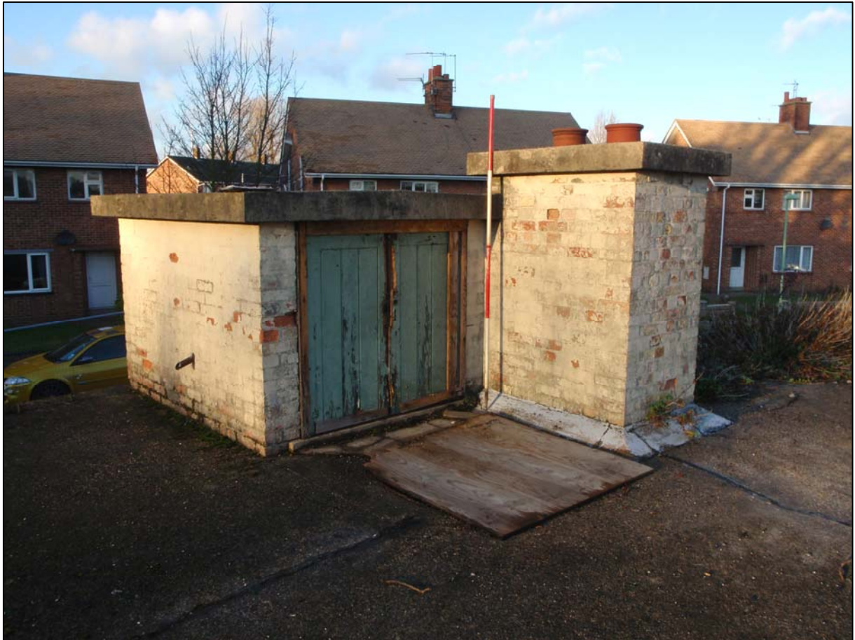
Plate 64. Roof mounted structure and chimney, camera facing north (ref. HLY 59)
