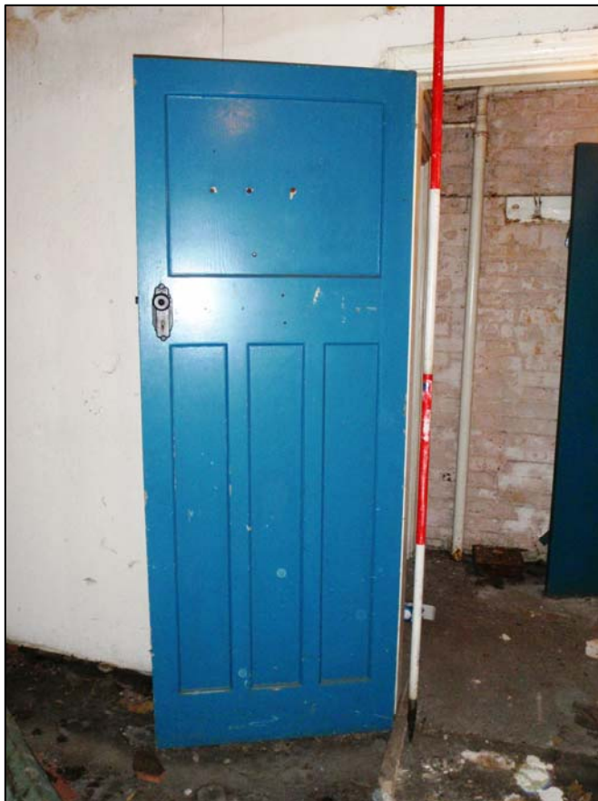
Plate 17. Room G7, camera facing north-east (ref. HLX 42)
