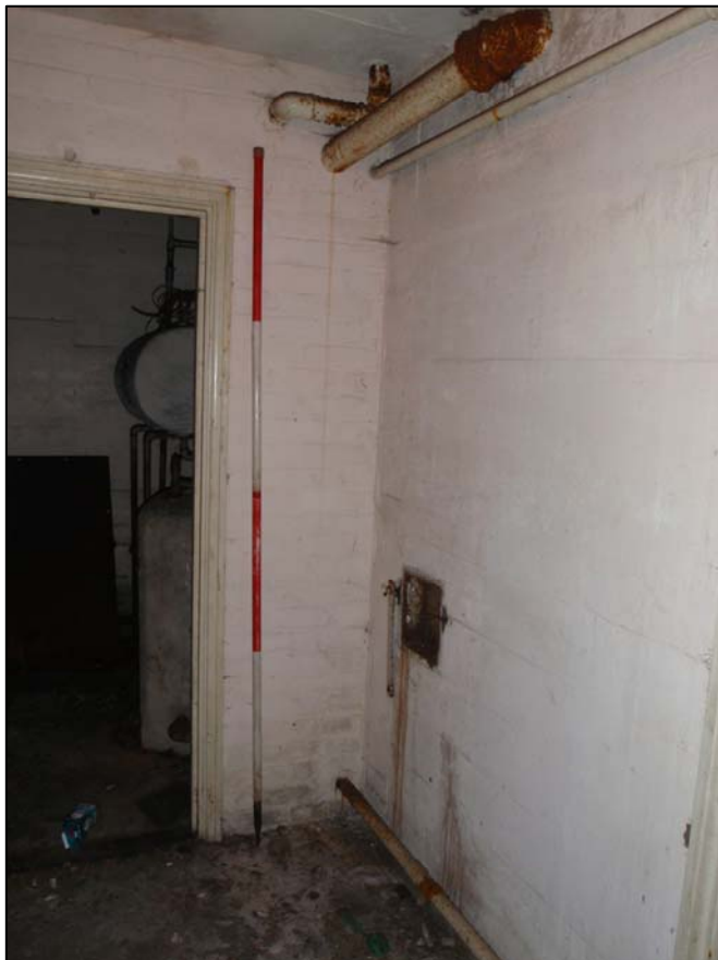
Plate 45. Room B1, camera facing north-west (ref. HLX 67)
