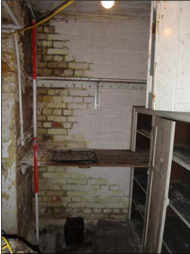
Plate 8. Room G4, camera facing north-east (ref. HLX 25)
