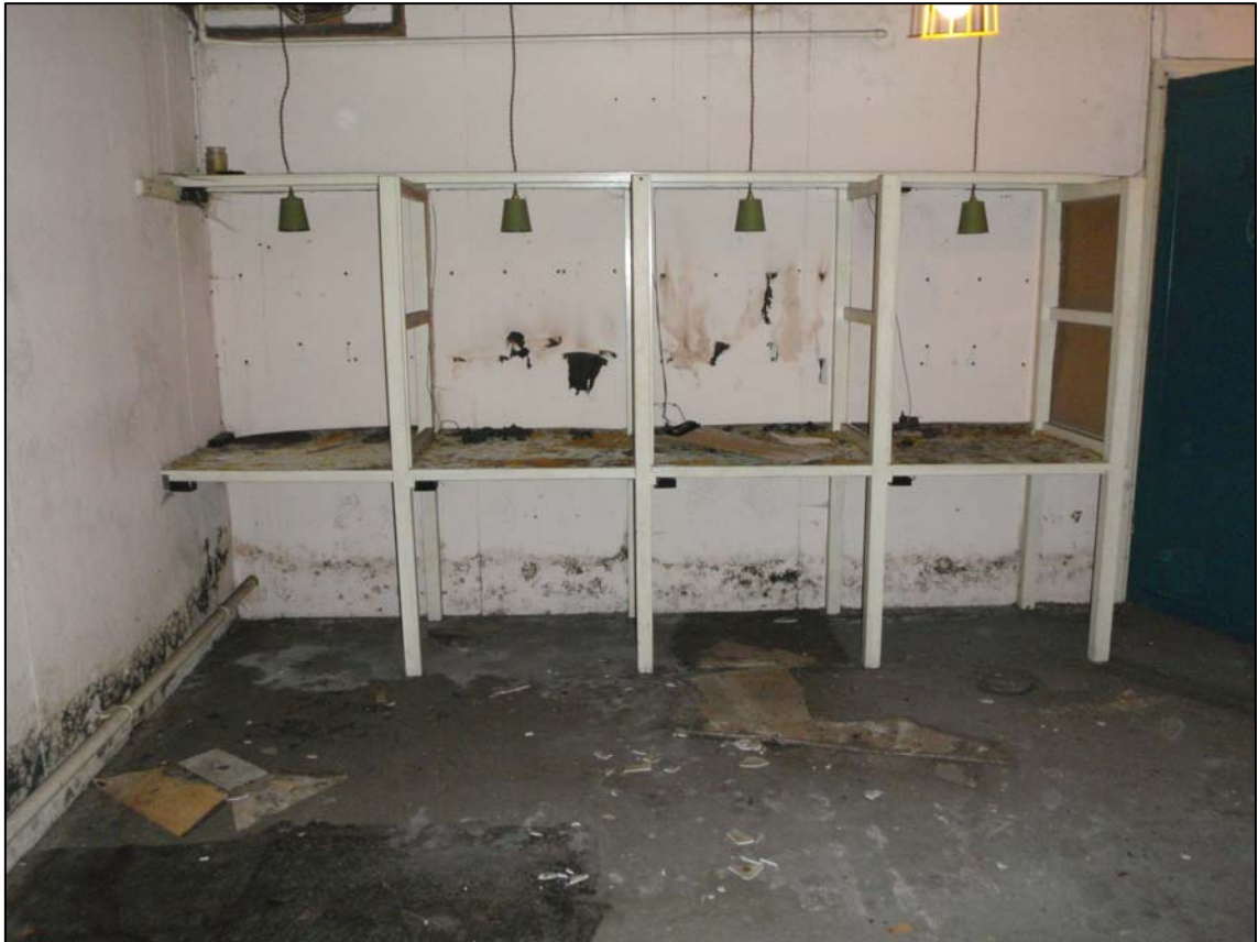
Plate 36. Room B3, camera facing north-west (ref. HLX 89)
