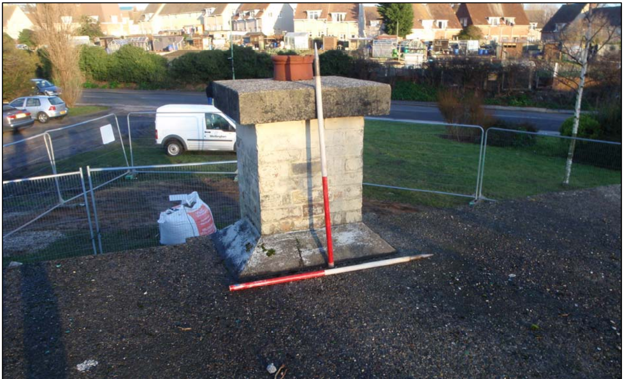
Plate 65. Roof, chimney, camera facing north-east (ref. HLY 61)
