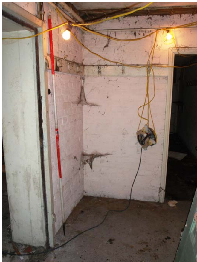
Plate 15. Room G6, camera facing south-east (ref. HLX 34)
