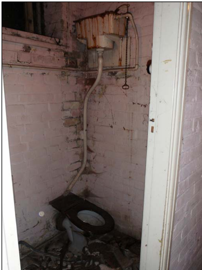
Plate 23. Room G10, camera facing west (ref. HLX 54)
