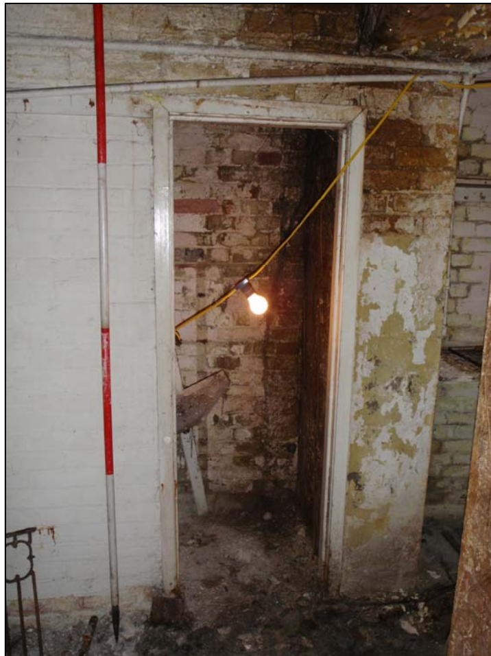
Plate 11. Room G5, camera facing north-east (ref. HLX 27)
