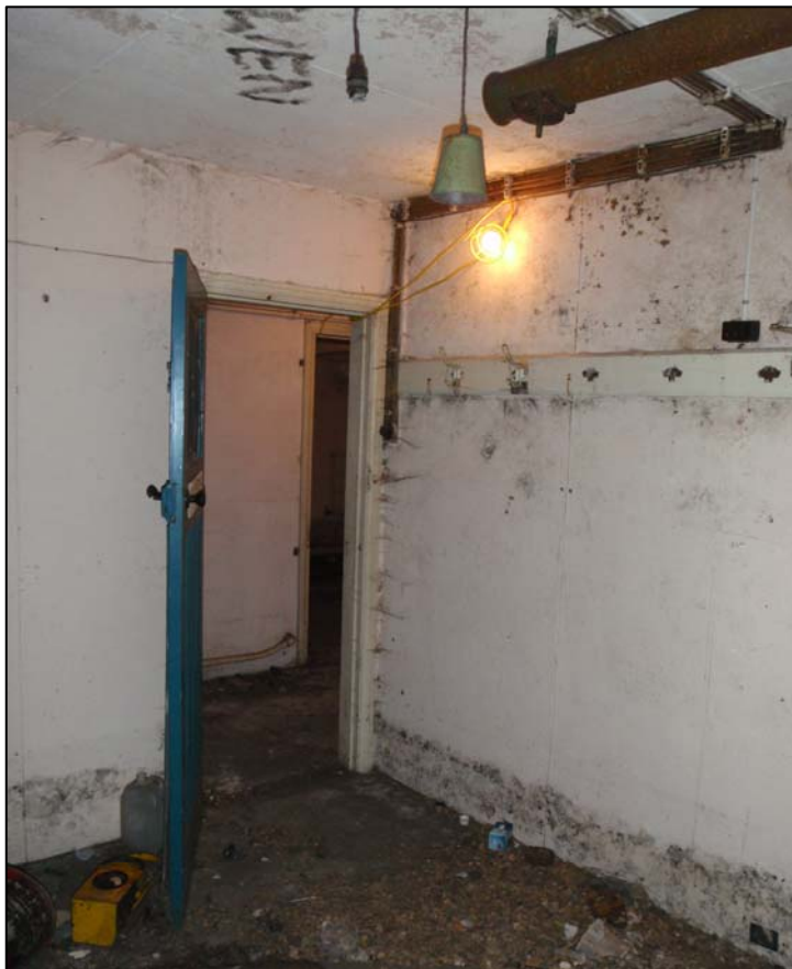
Plate 41. Room B4, door, camera facing east (ref. HLX 75)
