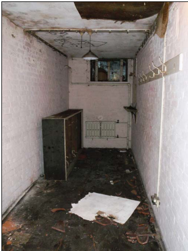
Plate 19. Room G8, camera facing south-east (ref. HLX 50)
