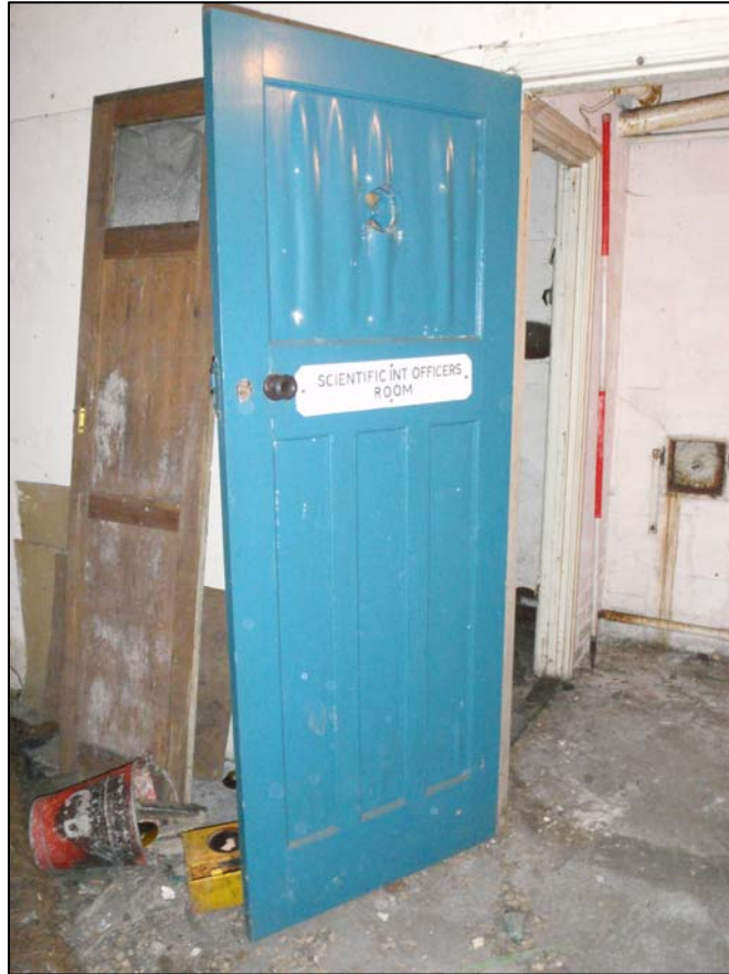
Plate 42. Room B3, door, camera facing north (ref. HLX 73)
