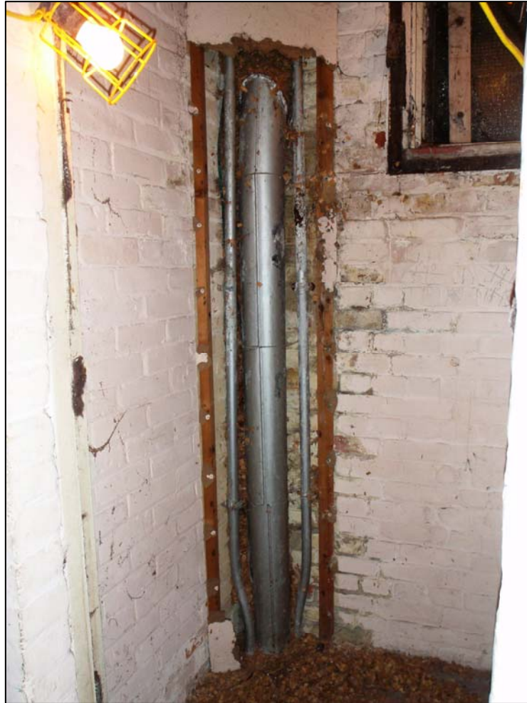
Plate 26. the exposed air supply pipe, camera facing south-west (ref. HLX 60)
