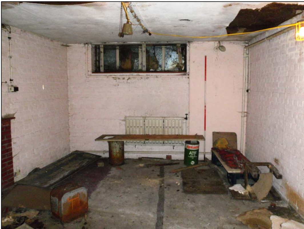
Plate 5. Room G3, camera facing south-east (ref. HLX 15)
