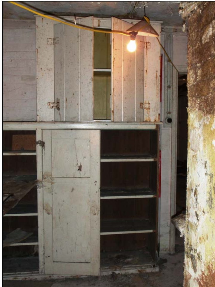
Plate 7. Room G4, camera facing south-east (ref. HLX 23)
