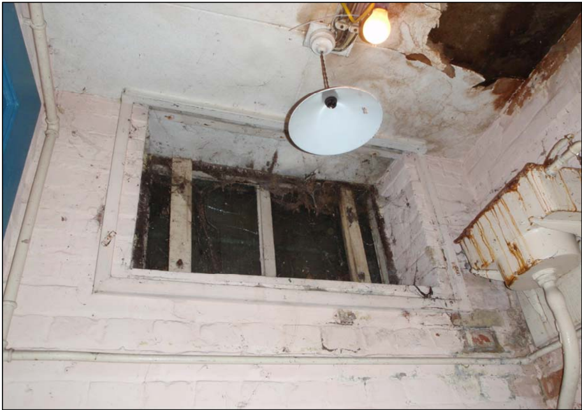
Plate 66. Room G10, window surround for internal shutter (ref. HLX 59)
