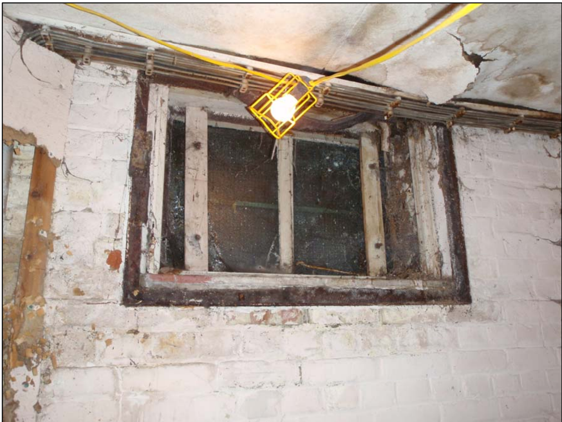
Plate 67. Room G12, window surround for internal shutter with felt for additional gas tight seal (ref. HLX 61)
