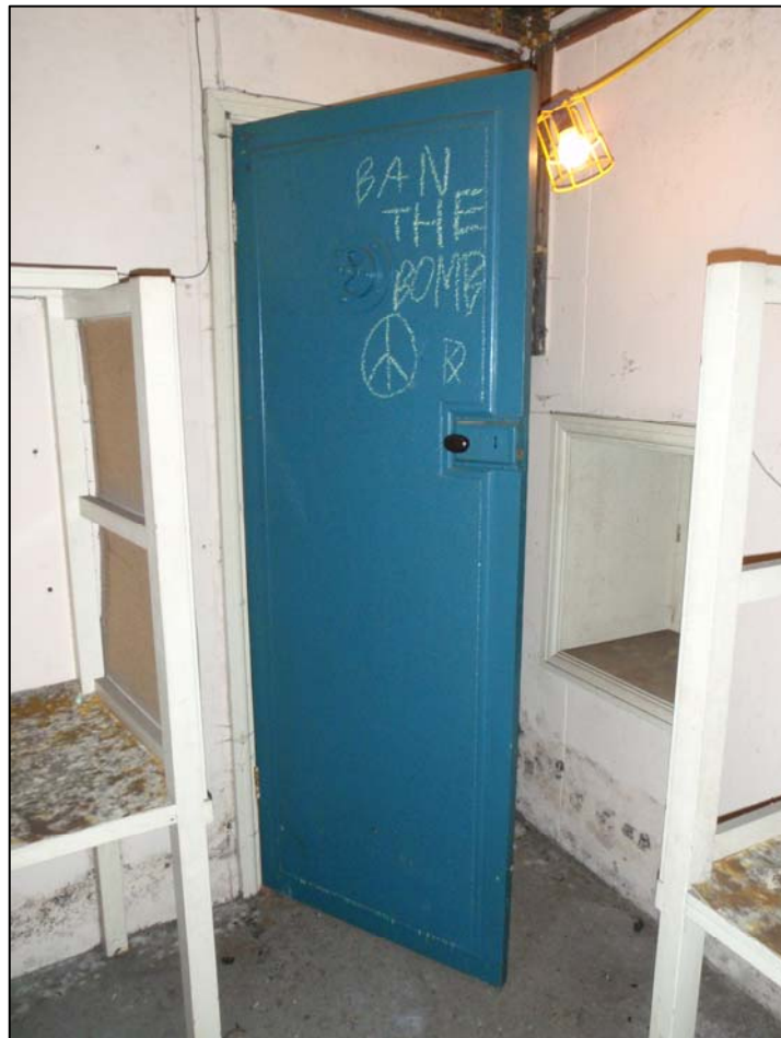
Plate 35. Room B3, door, camera facing north (ref. HLX 86)
