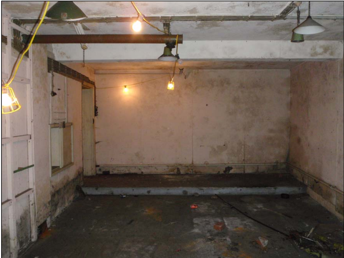
Plate 30. Room B2, camera facing north-west (ref. HLX 85)
