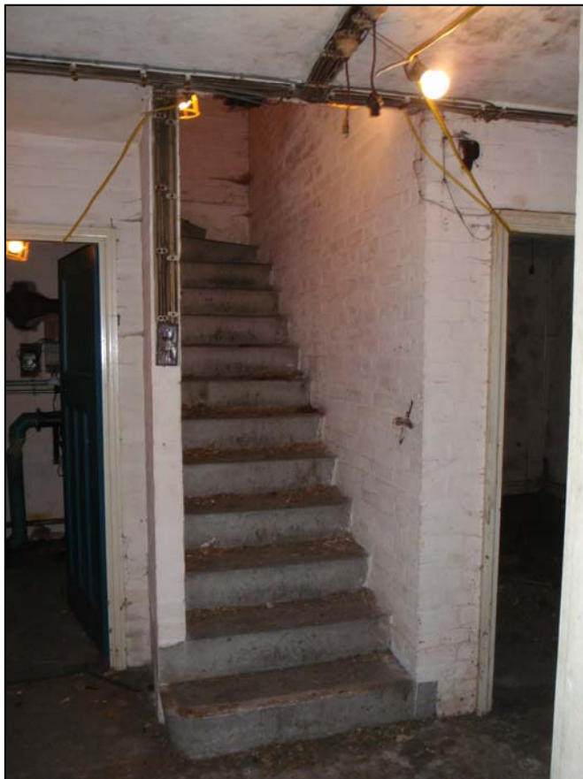
Plate 29. Room B1, bottom of the stairs, camera facing west (ref. HLX 76)
