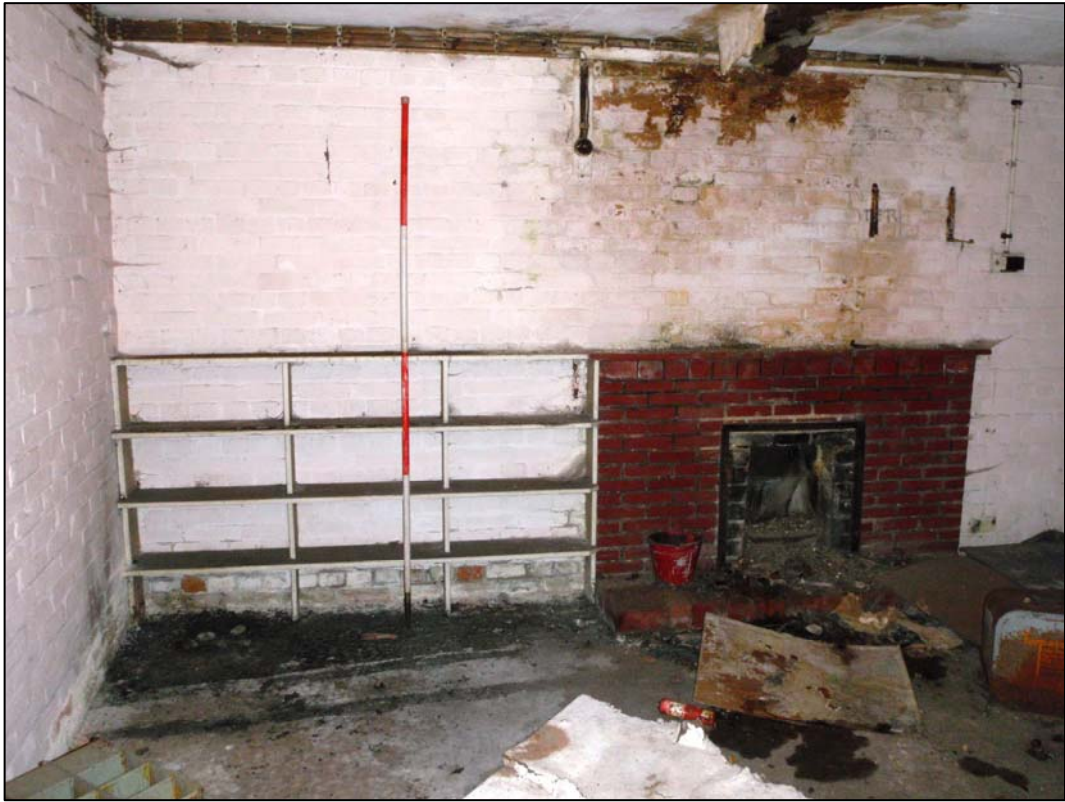
Plate 6. Room G3, camera facing north-east (ref. HLX 14)
