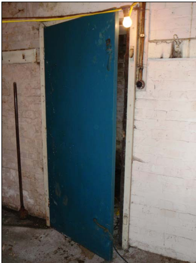
Plate 13. Room G6, view of the 'gas door', camera facing north-east (ref. HLX 48)
