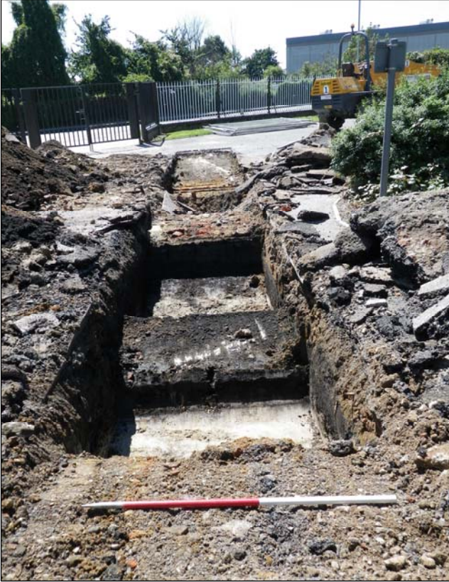
Plate 4. Trench 3, looking south west
