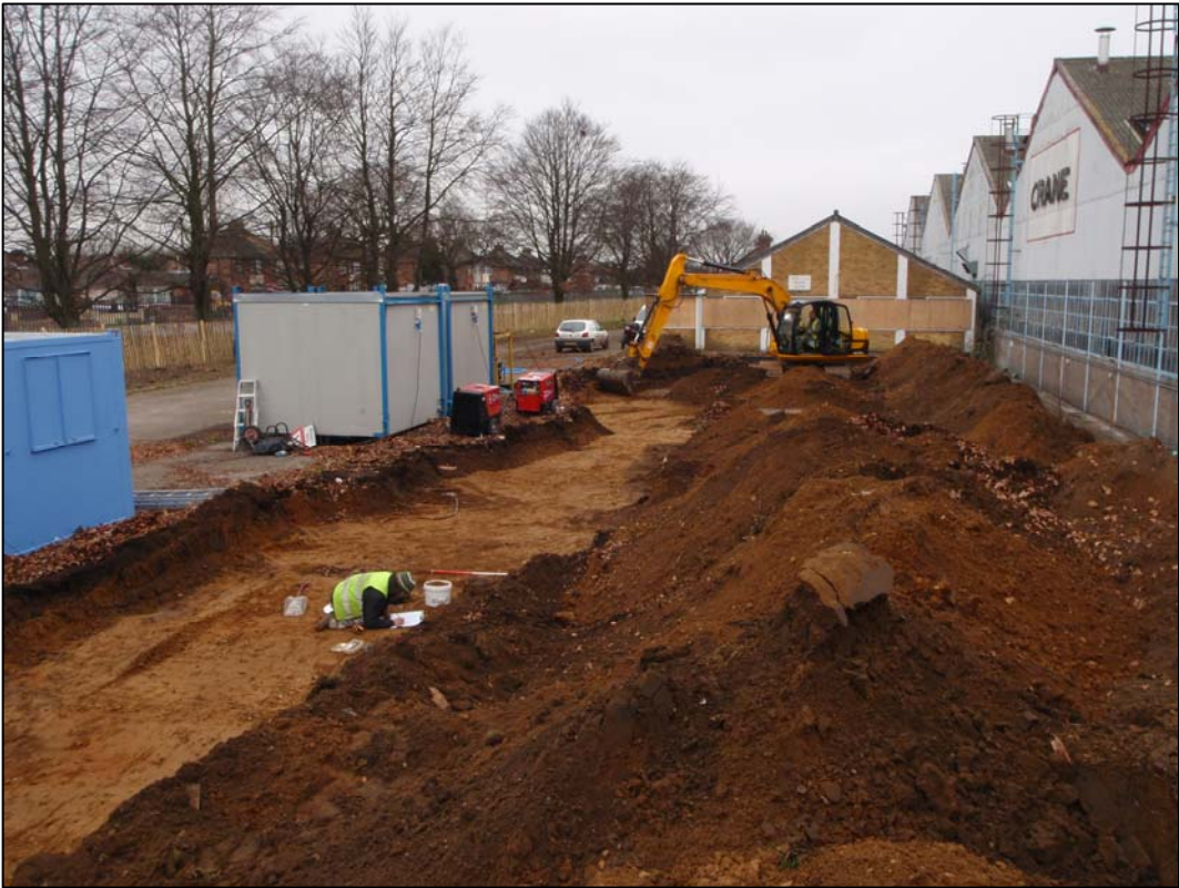
Plate 1. General view of site during soil strip (ref. HLW 76)
