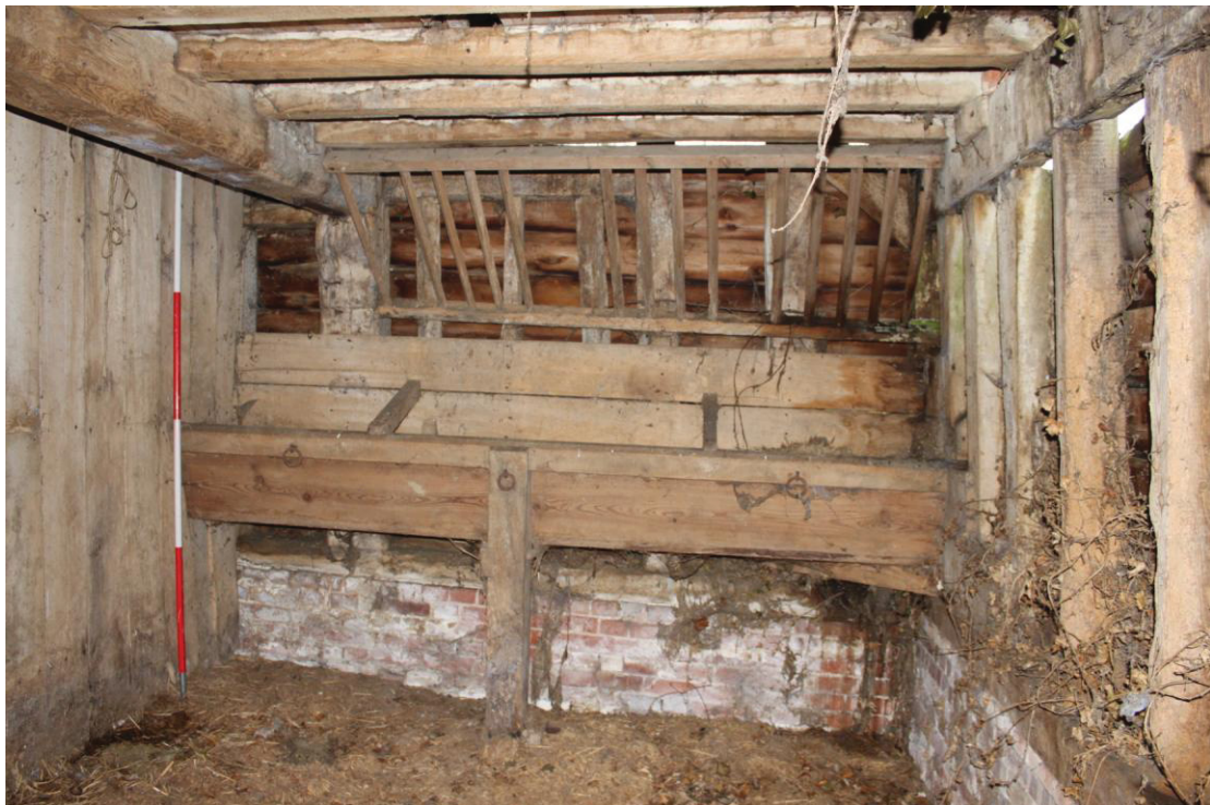
Illus. 10. The feeding trough and hay rack at the western end of the southern internal elevation (at horse height), showing the western gable to the right. Note the original diamond mullion window behind the rack (with original mullion to left), and evidence for additional mullions in the gable. A narrow shutter groove spans the entire width of this gable. The boarding to the left is a stall divider.
