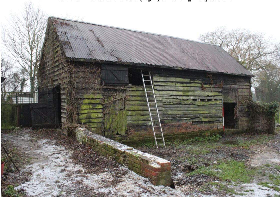
Illus. 3. Exterior of the outbuilding (1) from south-west showing loft loading hatch in western gable to left and farmhouse to right. The cladding and brick plinth are additions of the mid-19 th century, at which time the building may have been moved several metres to the east (right) of its original position.
