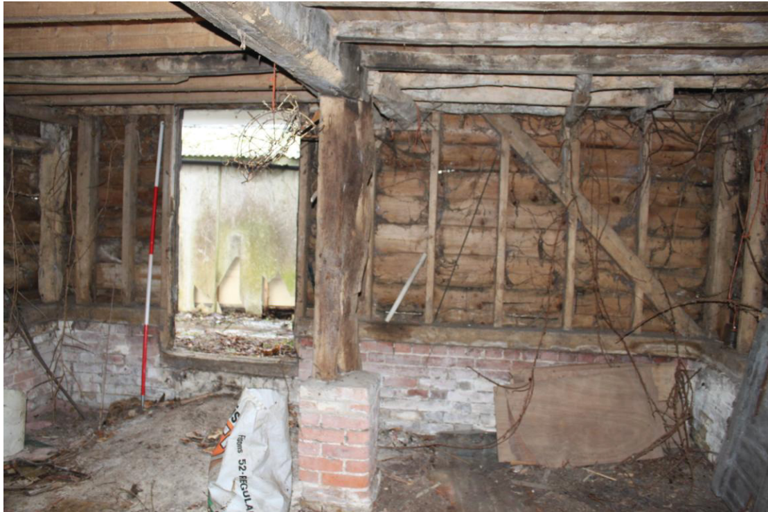
Illus. 7. Eastern internal gable showing 20 th century framing with a door opening towards the farmhouse. The central post is an insertion of the 19 th century which supports the end of the 17 th century axial ceiling joist where it would formerly have abutted a chimney.
