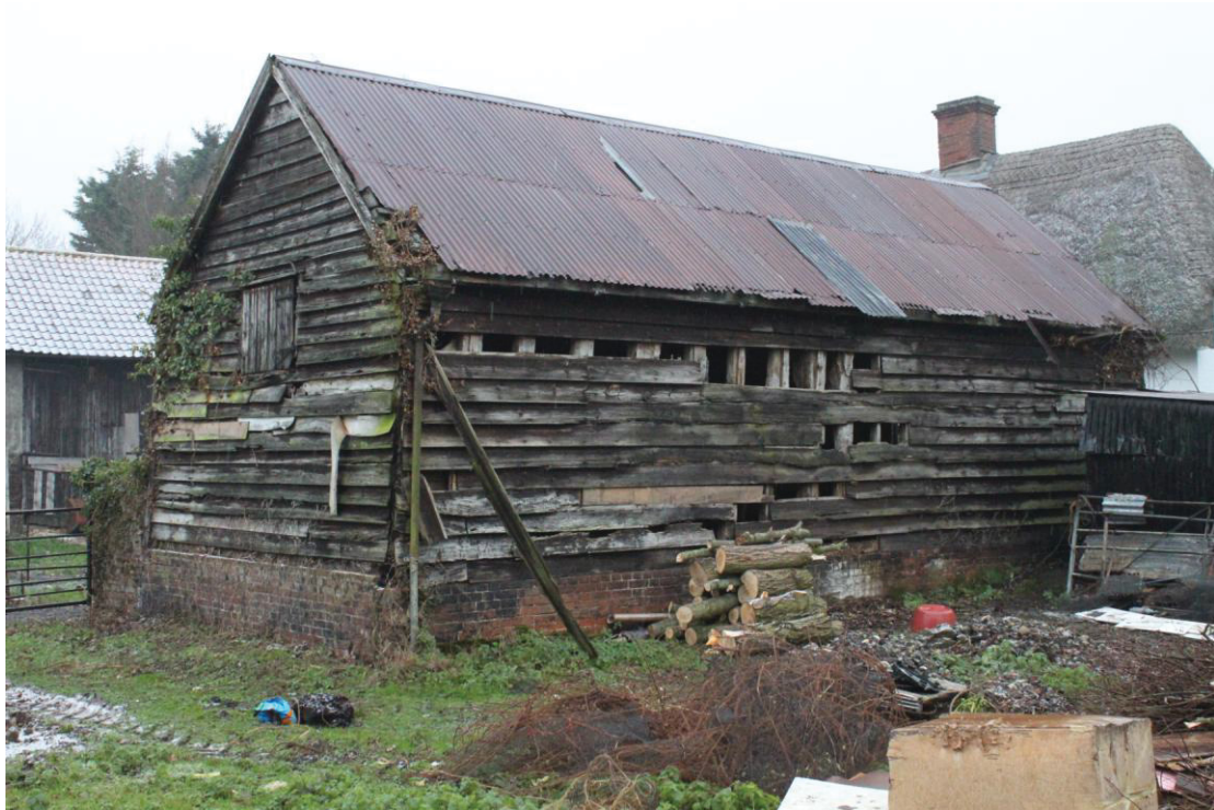
Illus. 3. Exterior of the outbuilding (1) from south-west showing loft loading hatch in western gable to left and farmhouse to right. The cladding and brick plinth are additions of the mid-19 th century, at which time the building may have been moved several metres to the east (right) of its original position.
