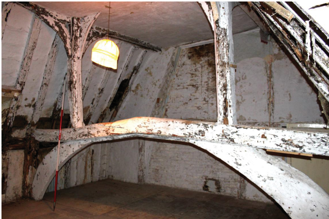
Illus. 2. The impressive queen-post open-truss of the 15 th century open hall in the farmhouse (2) seen from the low-end to the north-west. The whitewash conceals heavy sooting. Included for site context.
