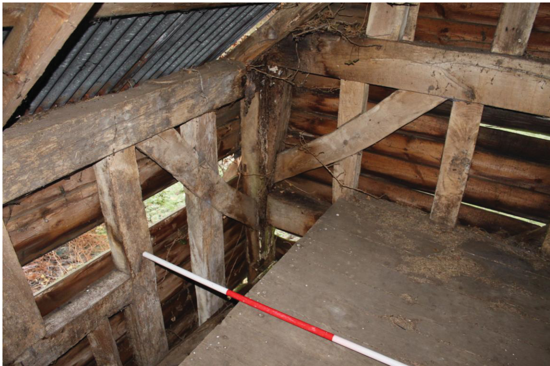
Illus. 8. Internal south-western corner of western loft showing corner braces & original diamond-mullion window to left. The left-hand mullion (not visible here) is the only original mullion to survive in situ . The western half of the building dates from the late-16 th century in contrast to the 15 th century eastern half.
