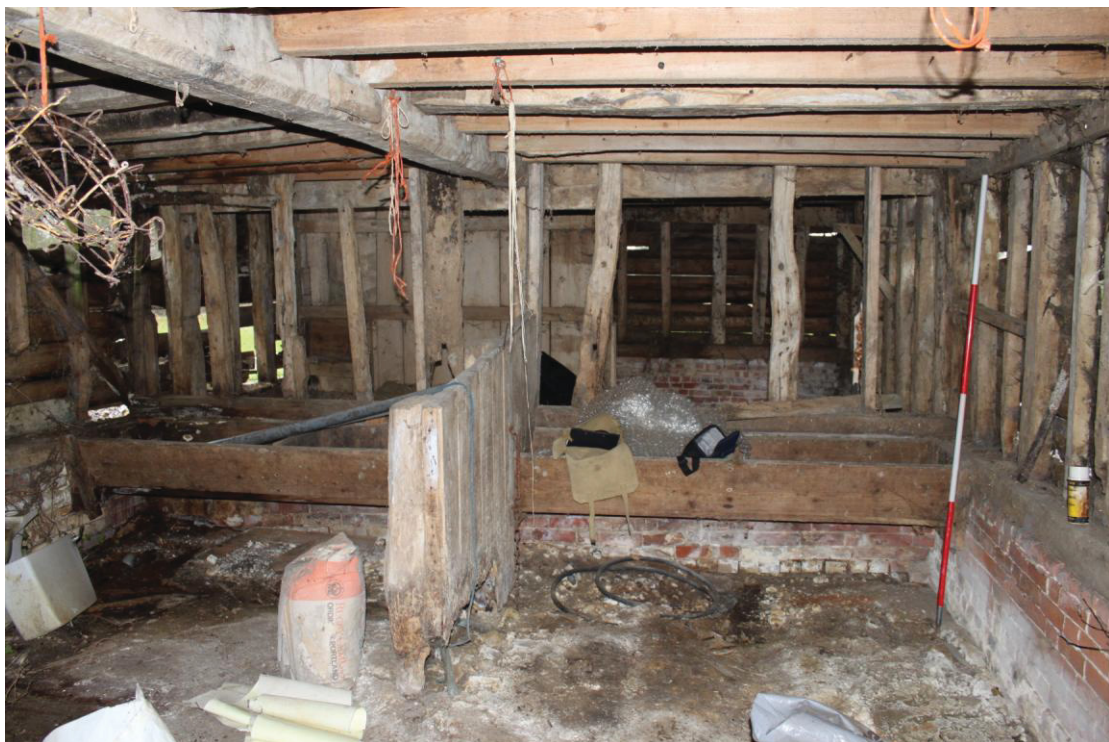
Illus. 6. Internal 'high-end' partition from east showing the low cattle manger and axial stall divider on the ground floor. A sooted original stud is visible to the left of the divider.
