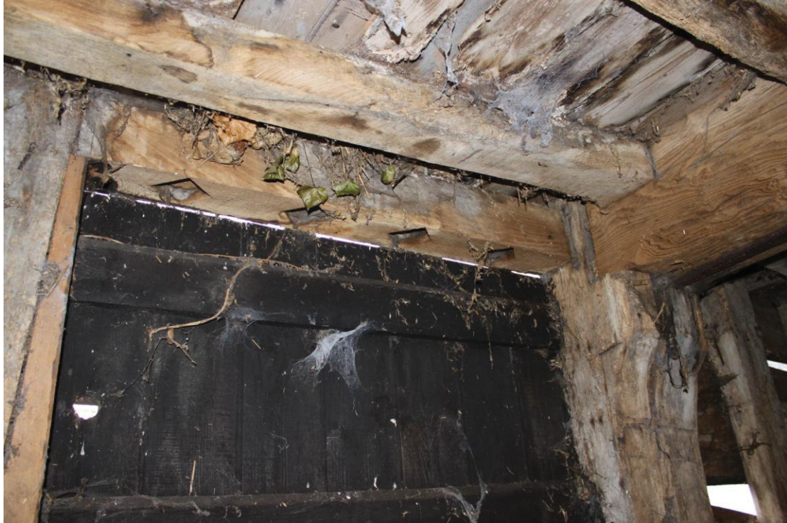
Illus. 9. Detail of the original diamond mullion mortises in the lintel of the northern door of the western stable. The step-stop chamfered binding joist with a neatly-cut corbel block is visible to the right.
